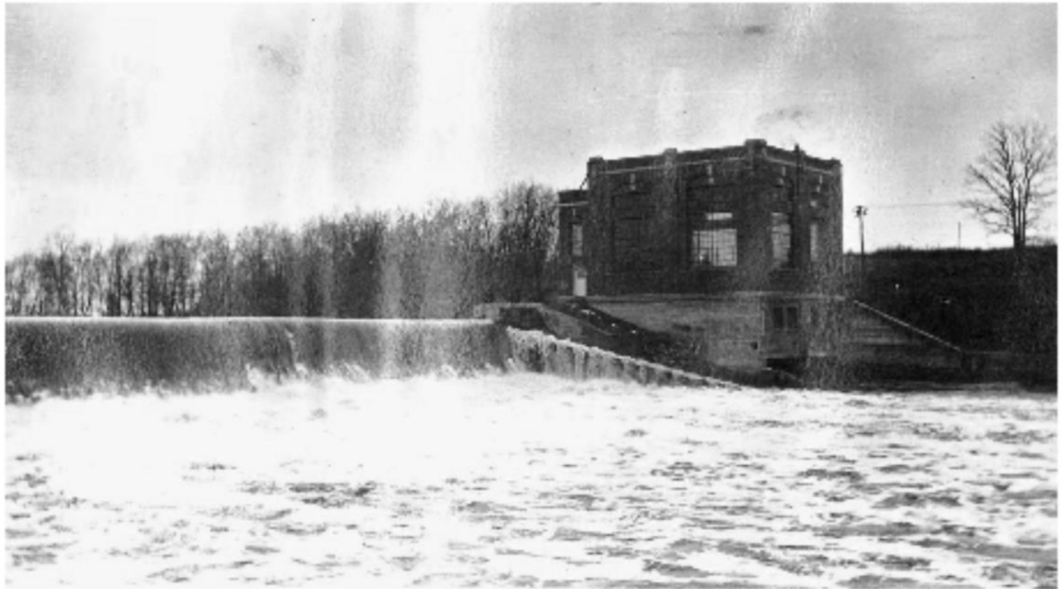
Photograph 3: View of Dam spillway
