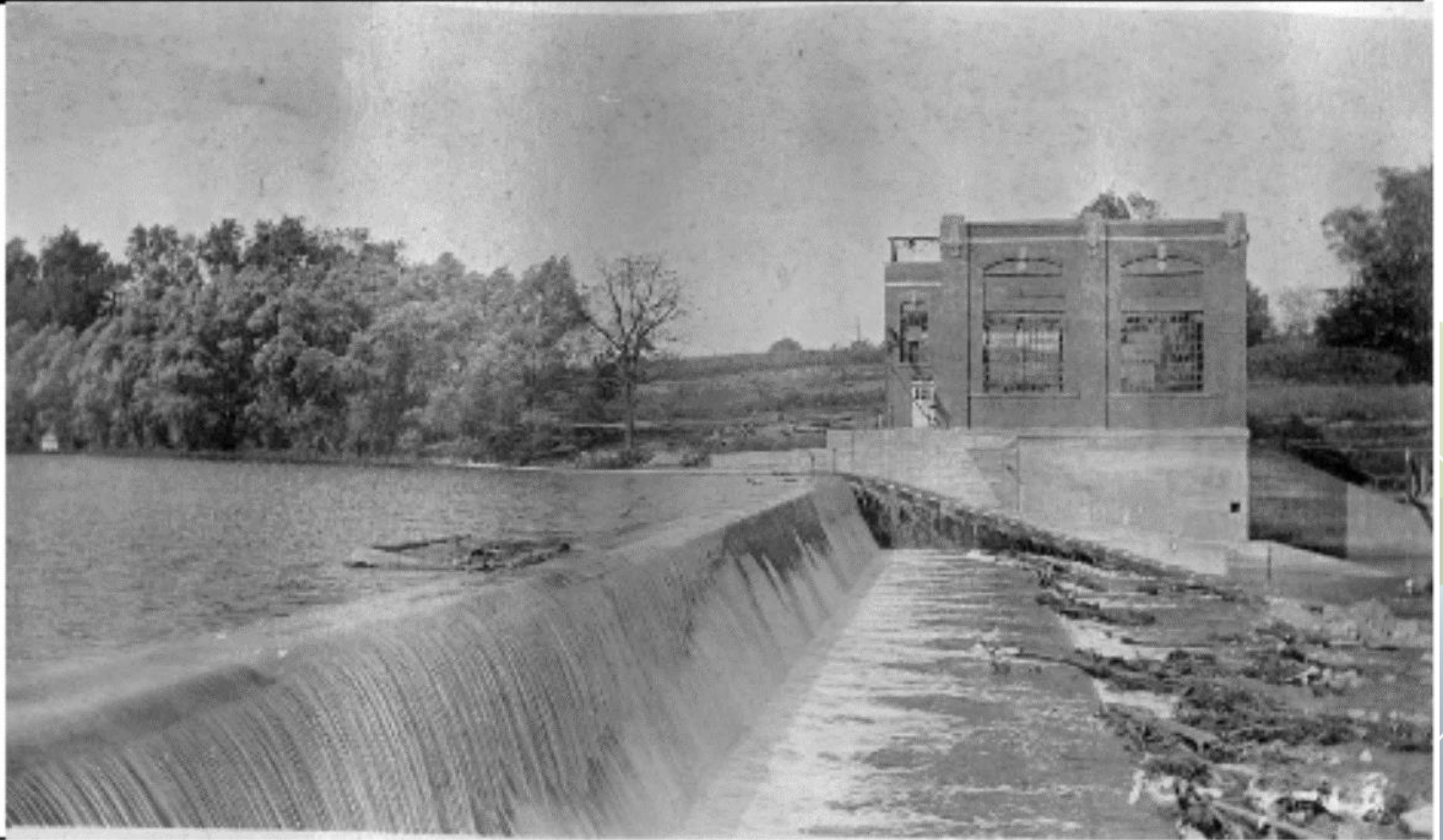
Photograph 6: Spillway after reconstruction
