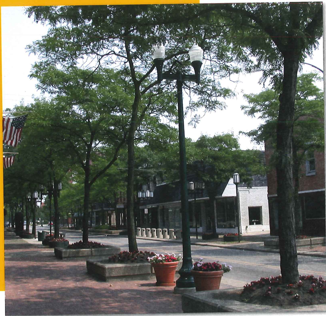
View of the Streetscape project completed by Beckett & Raeder, Inc. for the city of Ypsilanti, Michigan
