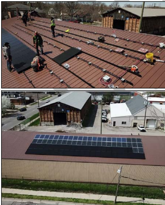
Figure 1. Solar array Installation on City of Ypsilanti Department of Public Service carport. Source: solarypsi.org
