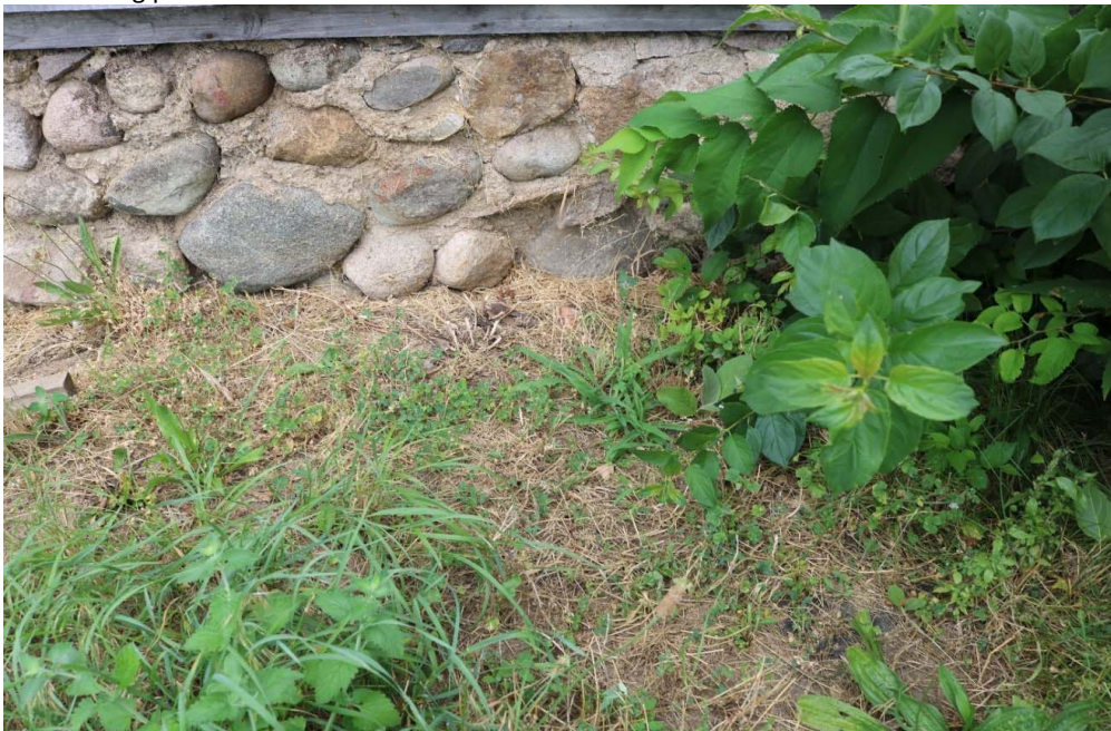
Surrounding photos of northeast corner of house – north side where porch used to stand
