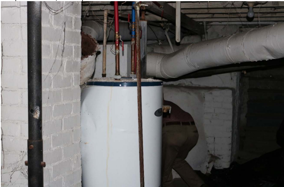
Octopus Ductwork, chimney is white brick, furnace is located on the other side of water heater
