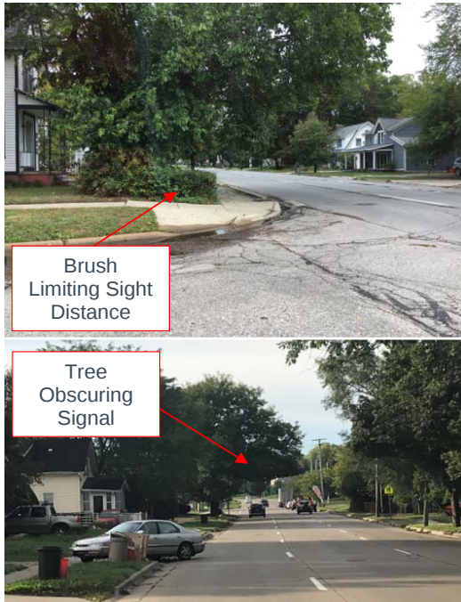
Figure 5-25 Sight Distance and Signal Obstructions
