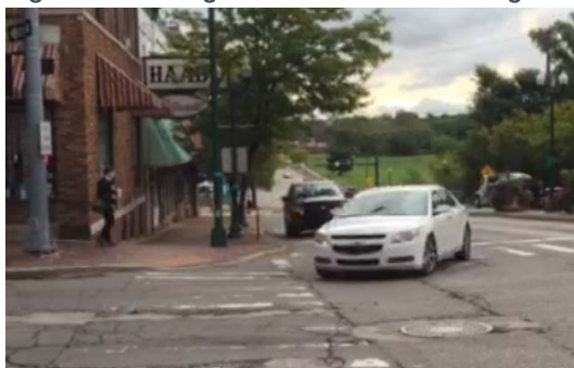
Figure 5-24 Right-Turn Conflict at Michigan Avenue
