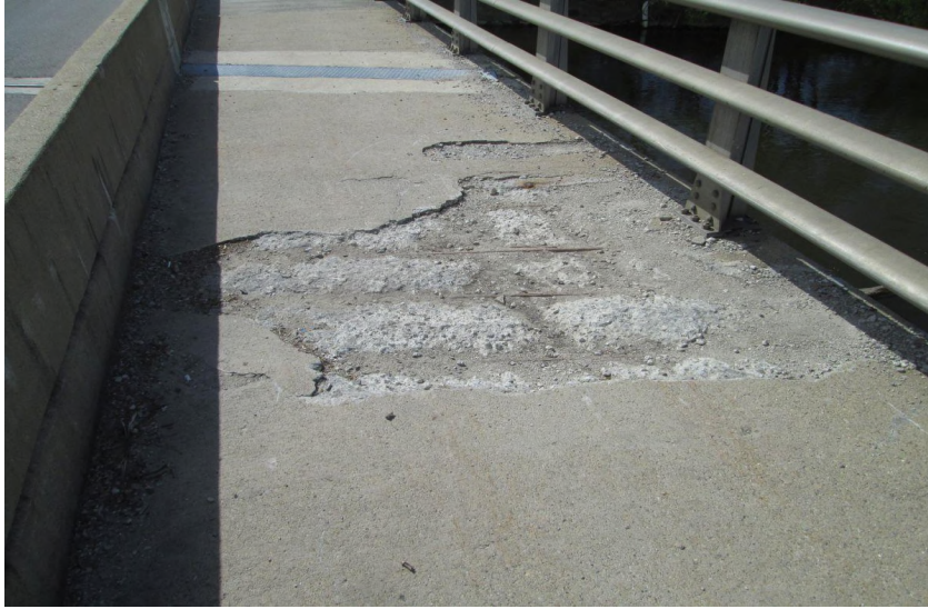
Sidewalk Spalling
