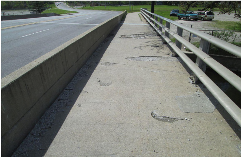
Sidewalk Spalling
