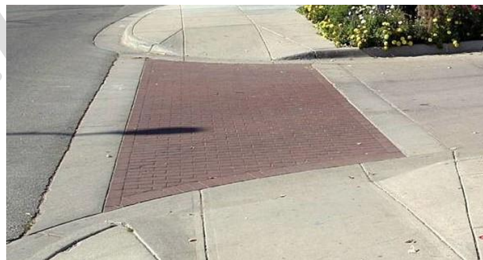
Figure 25: Driveway Apron Example
