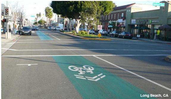
Painted sharrows next to existing parking
