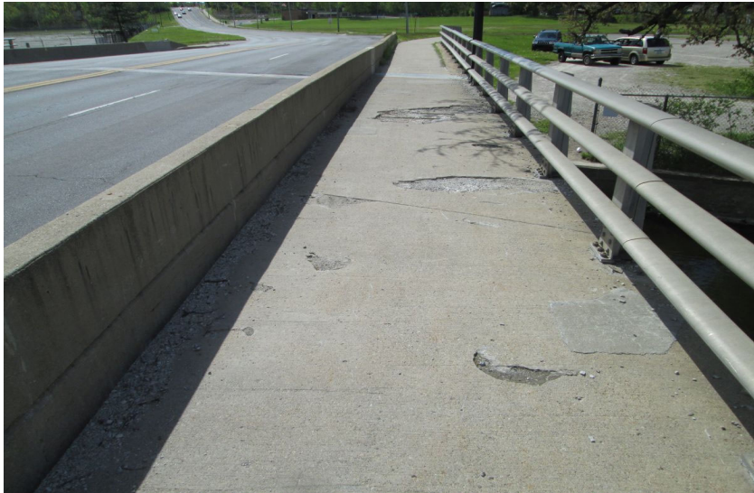
Sidewalk Spalling
