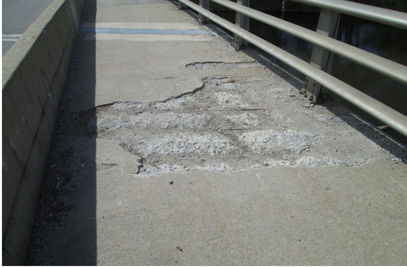
Sidewalk Spalling
