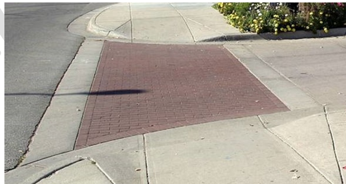
Figure 25: Driveway Apron Example
