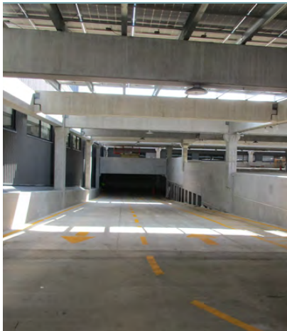
BRIDGE AND STOCKING PARKING STRUCTURE GRAND RAPIDS, MICHIGAN
