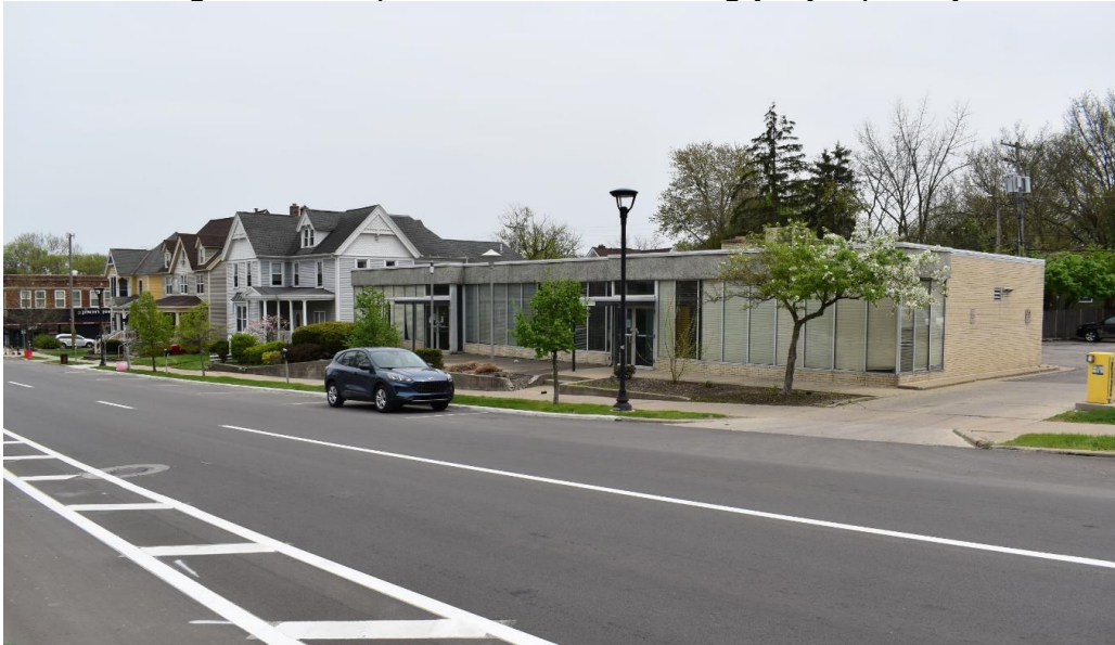
Figure 2: Photo, Front of Current Building (May 11, 2022)
