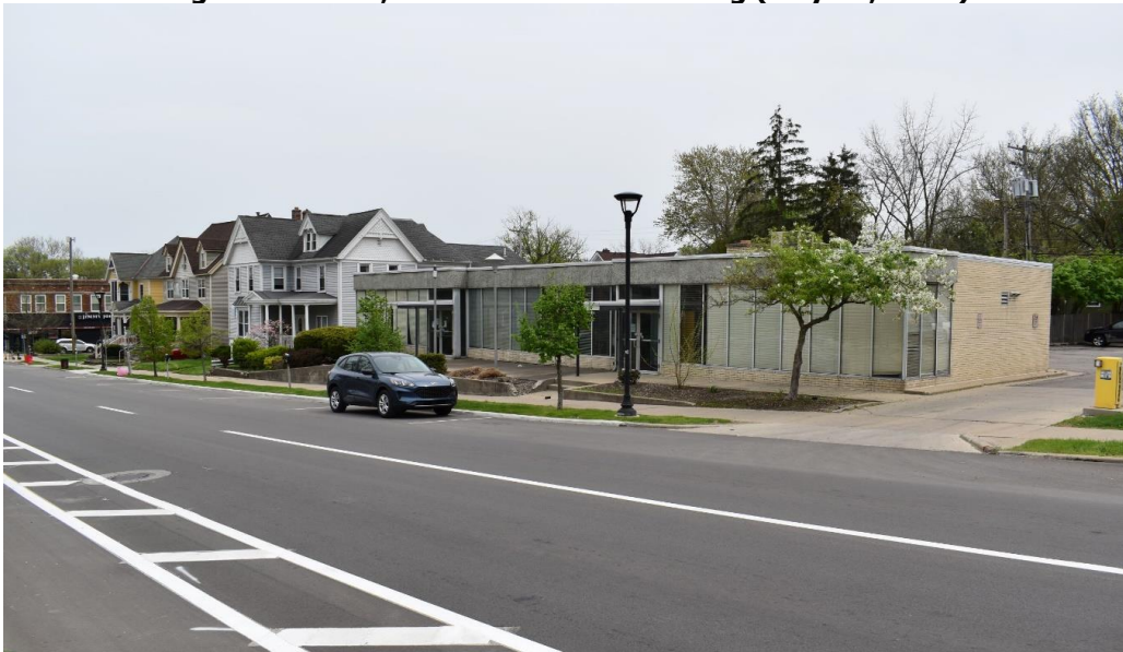
Figure 2: Photo, Front of Current Building (May 11, 2022)
