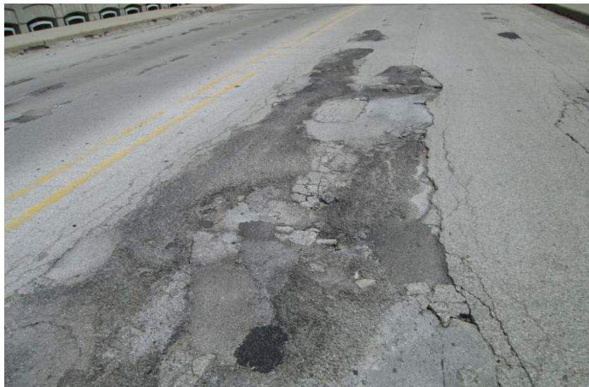
Typical Spalling
