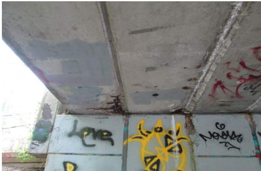
Stringers - East Span
