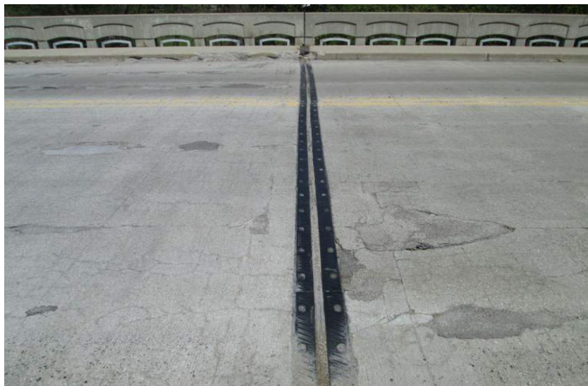
Pier Joint East
