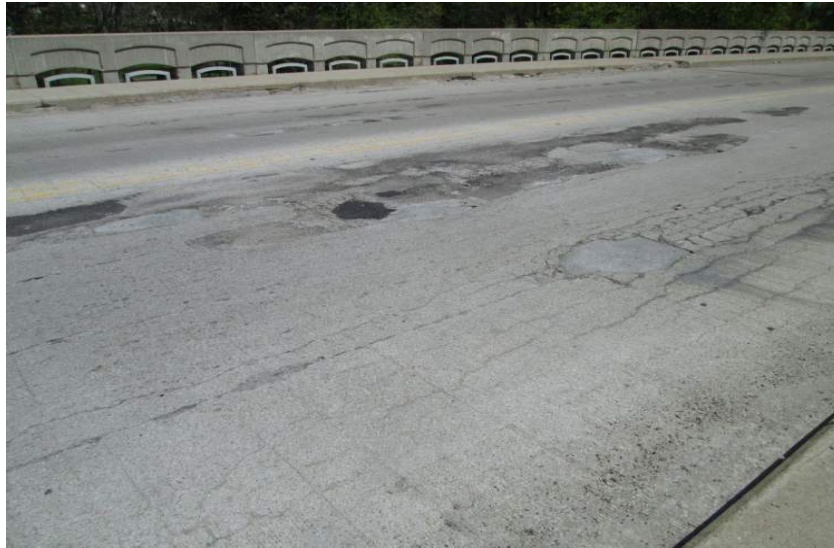
Surface Middle Span
