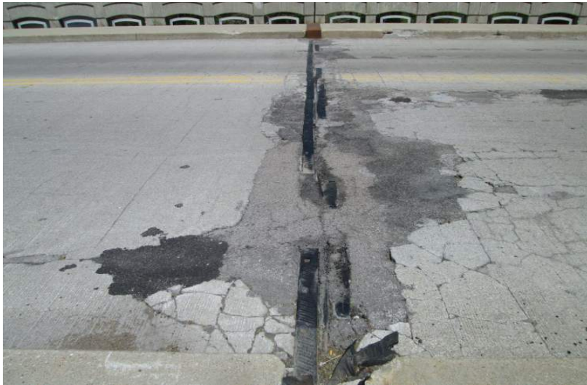
Pier Joint West
