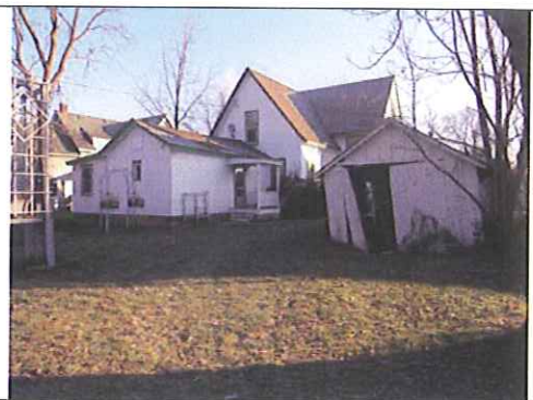
House at 509 N. Adams – view from the rear
