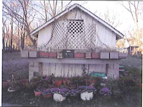
Shed exterior – east elevation
