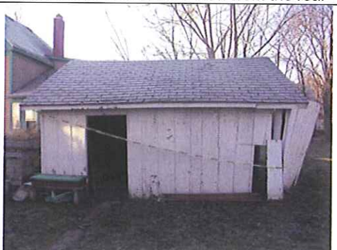
Shed exterior – north elevation
