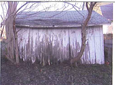
Shed exterior – south elevation
