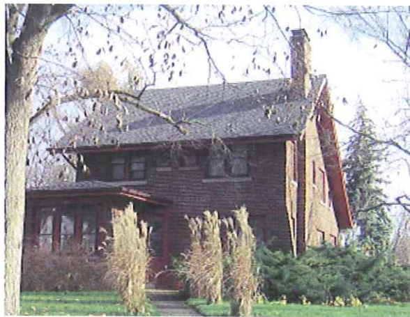
This masonry vernacular located at 204 Elm St. shows an influence from the Prairie Style by its use of battered walls.
