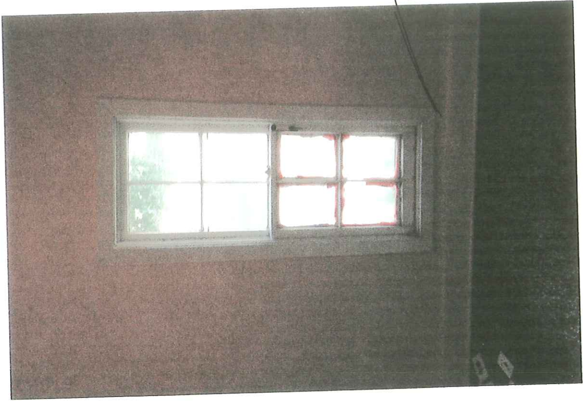
INTERIOR OF FRONT WINDOW
