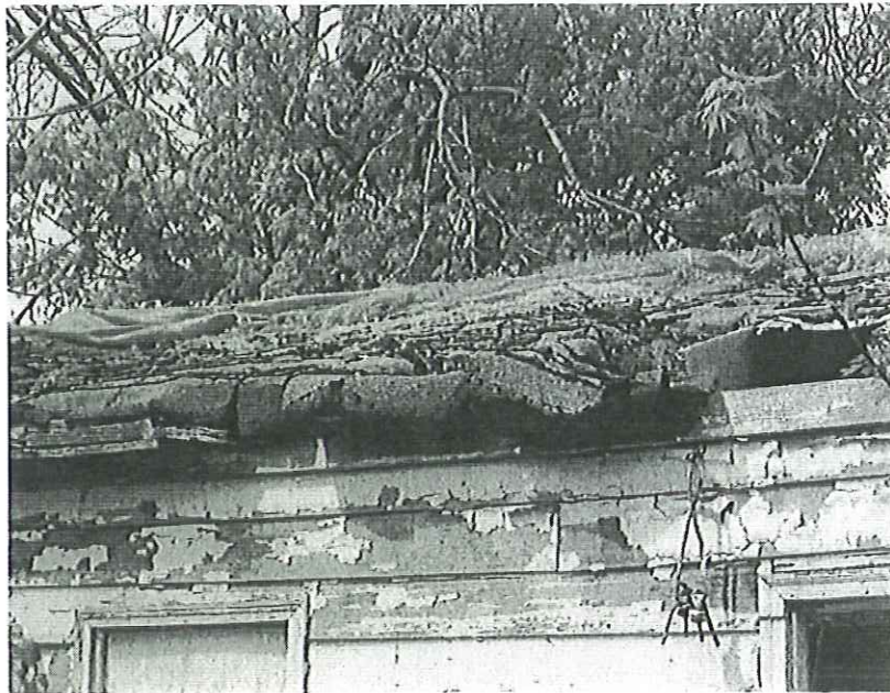
Roofing Damage Detail
