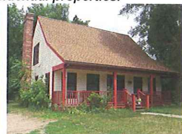
Solar panel installation would not be approved in the roof location visible in this photograph.
