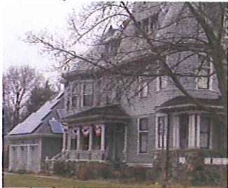
Example of solar panels that are not visible from the front of the structure and installed on an attached non-historic structure.
