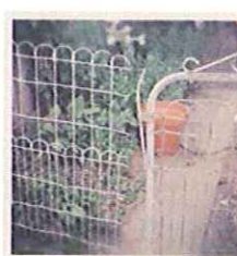
Twisted wire with wooden posts
