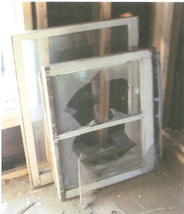
Photo 3. Broken two pane sash found upstairs.
