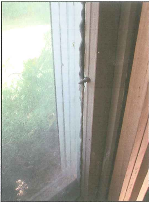
Photo 1. Single pane window with sash pin
