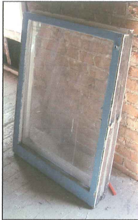
Photo 2. Single pane windows with sash pins
