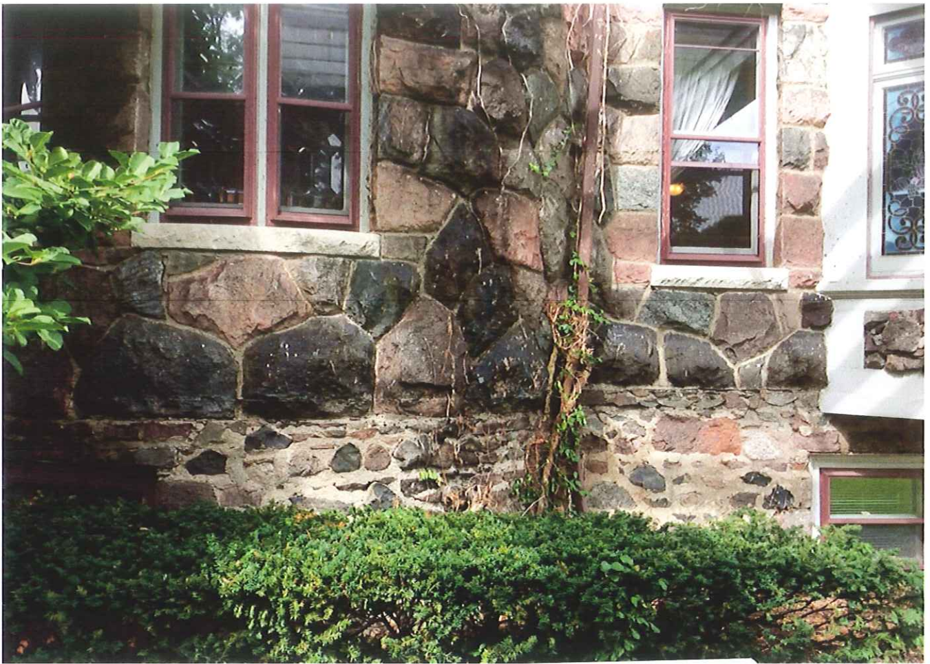
South side of building
