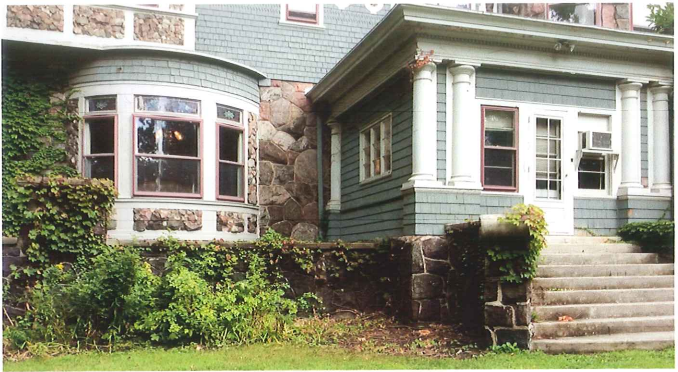
West side of building
