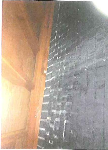
Existing brick is painted, and appears in good condition.
