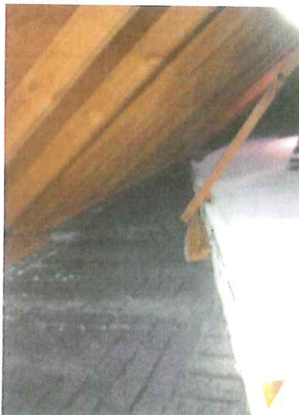
The peak of the gable was removed to install the existing wood soffit.
