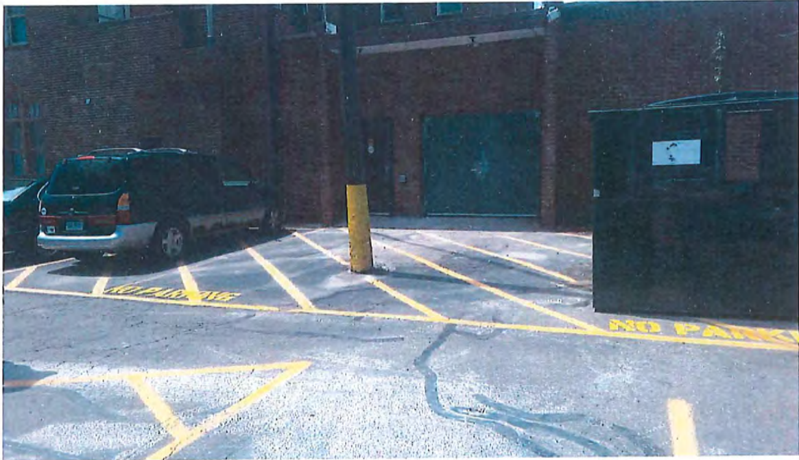
Photos of Exterior of Future Ypsi Alehouse Spent Grain Storage Area
