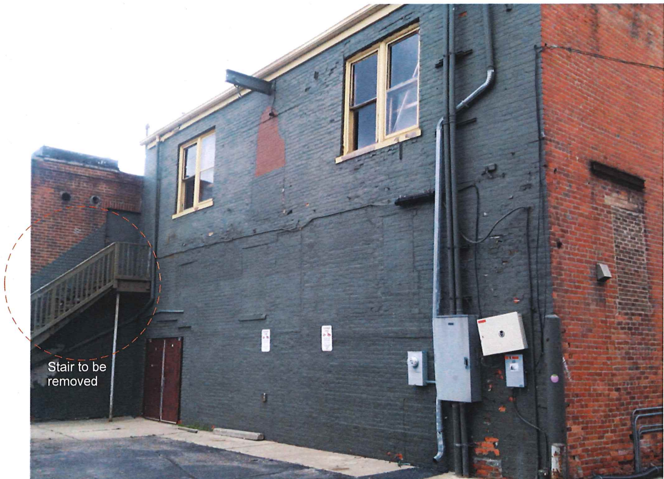
Existing Back View
