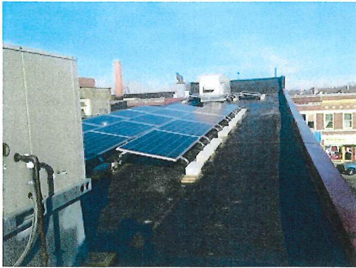
Lifting material to the roof
