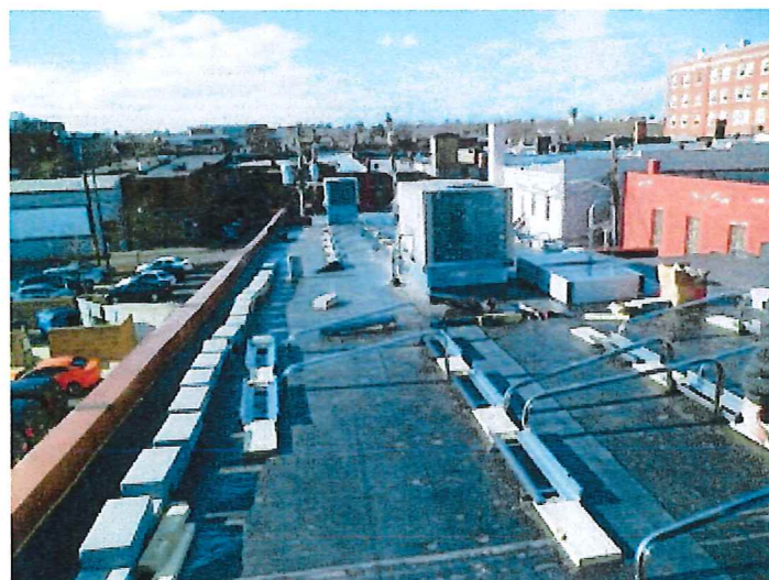
Setting up the racking
