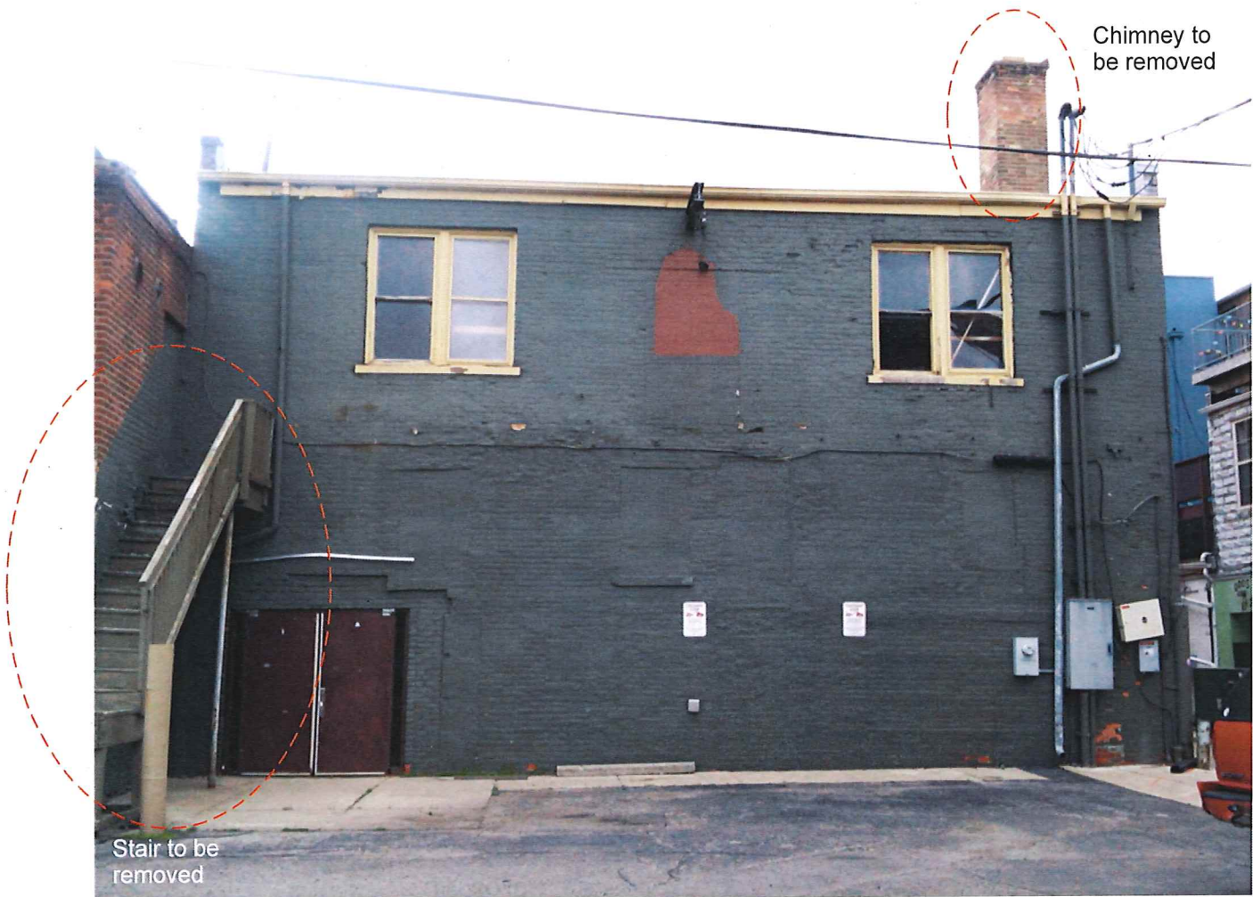
Existing Back View
