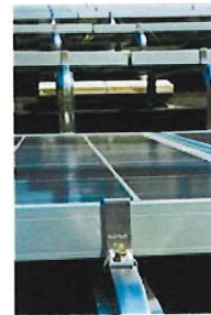
Panel Clamps with Integrated Grounding
