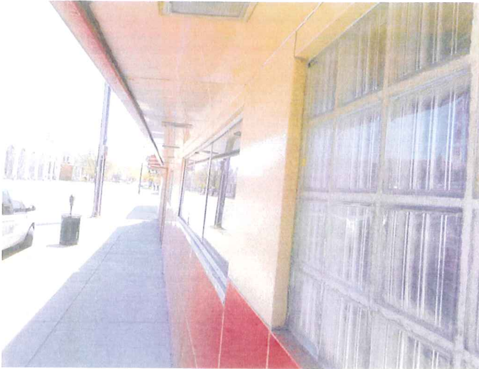
Photo #13 - Looking south along underside of canopy.
