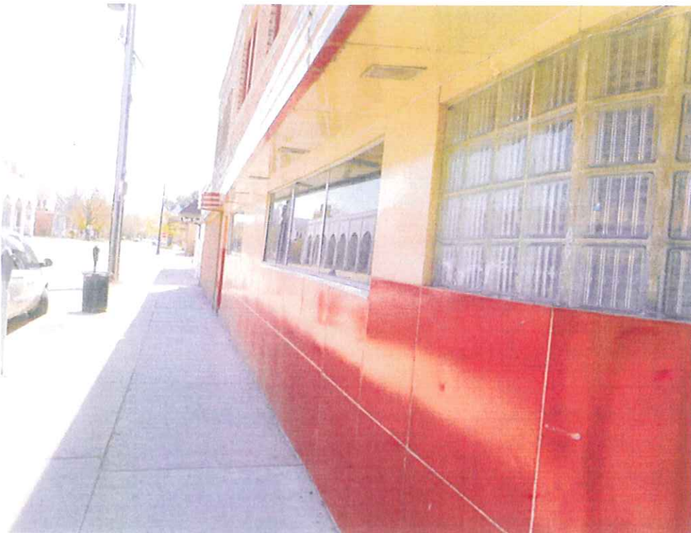
Photo #14 - Looking south along east wall.
