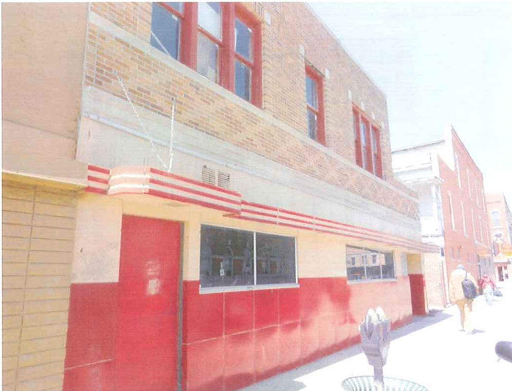
Photo #4 - Looking northwest.
