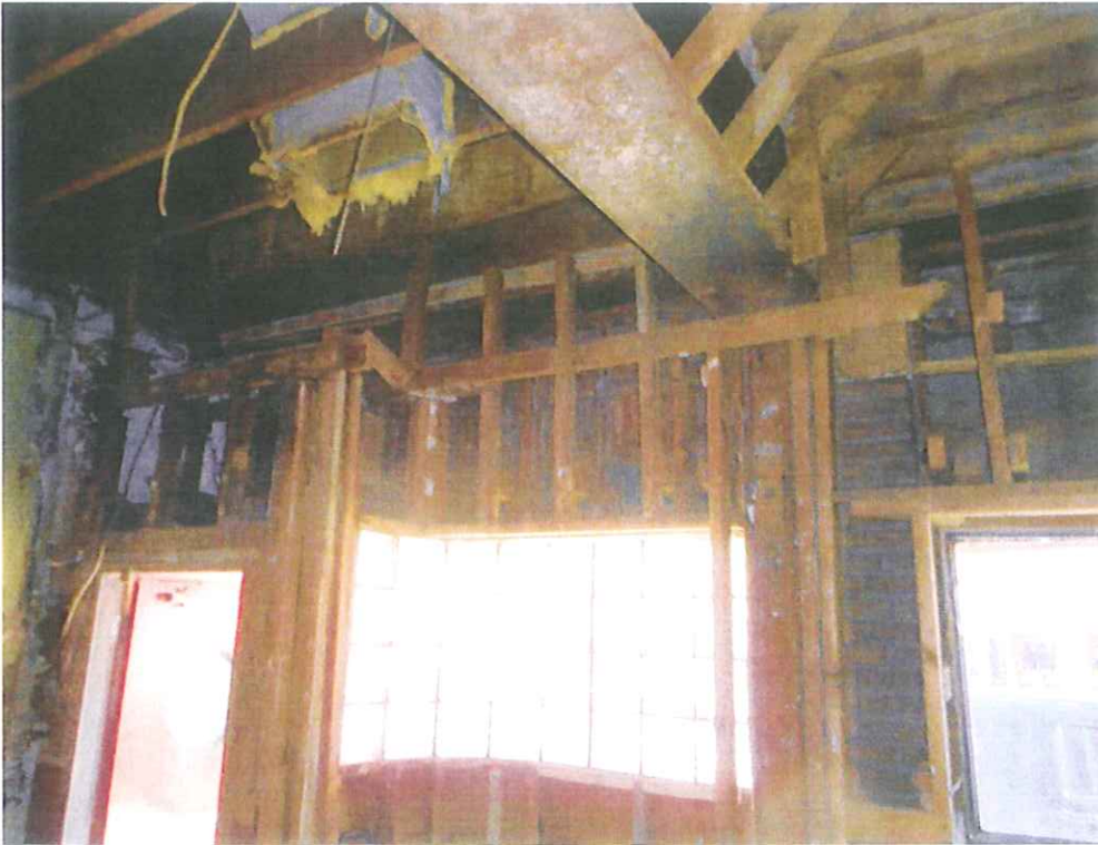
Photo #9 - Interior canopy support at north door and glass block area.
