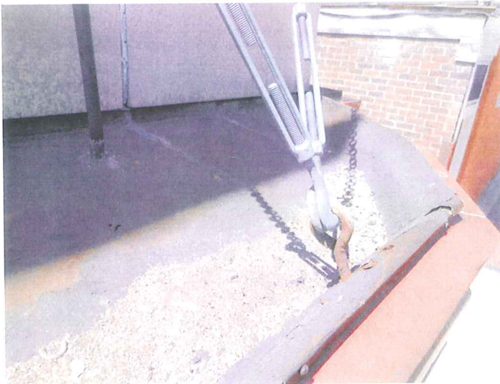
Photo #5 - Screw-eye attachment of non-original chain and turnbuckle suspender. Note several older holes through metal roof left over from previous locations of screw-eye.
