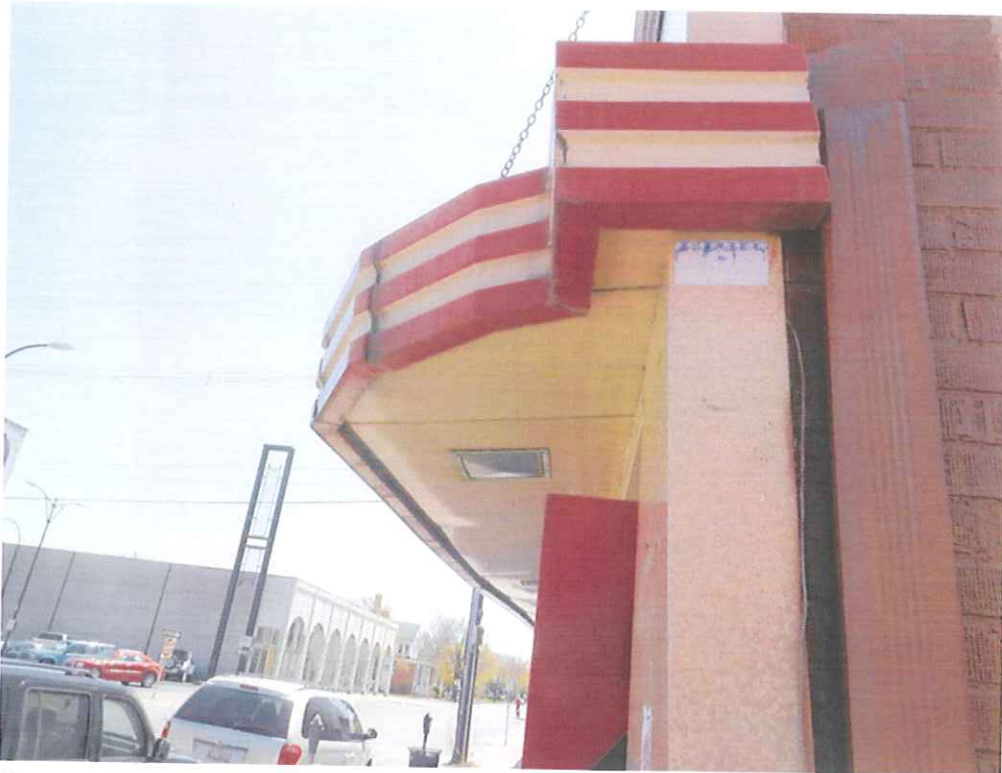
Photo #11 - Canopy drains into downspout at north end.
