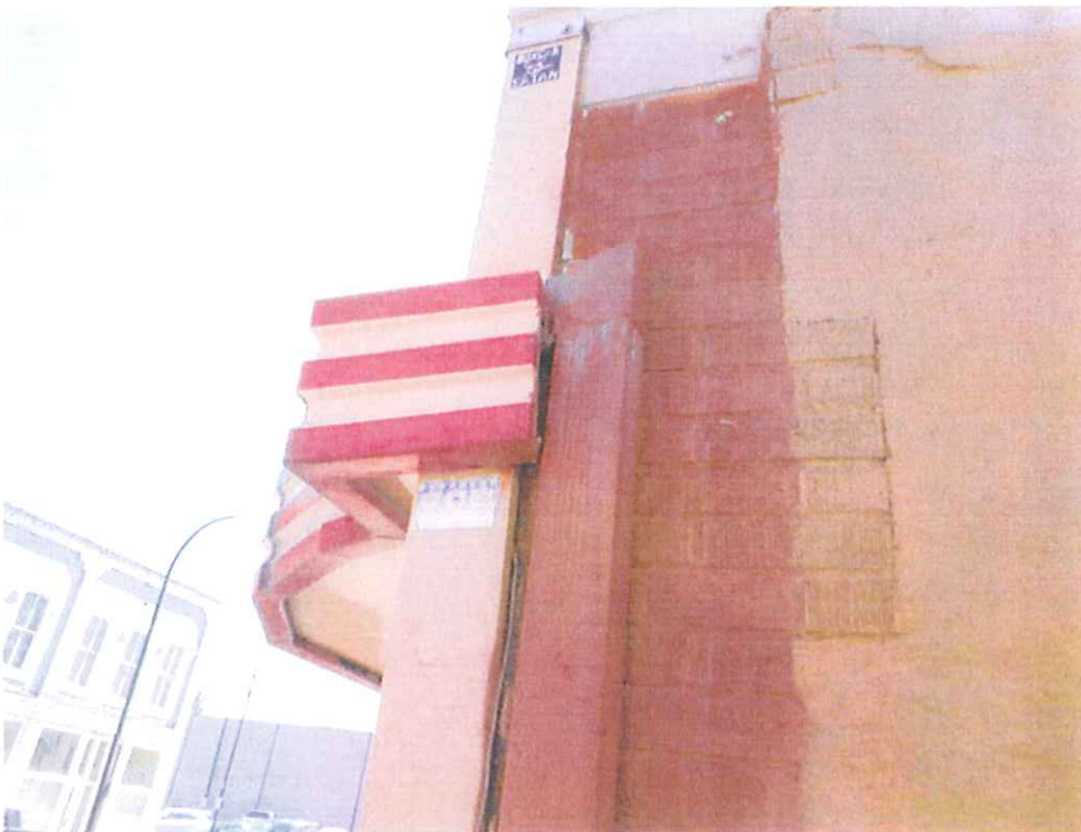
Photo #10 - Canopy drains into downspouts at north end.
