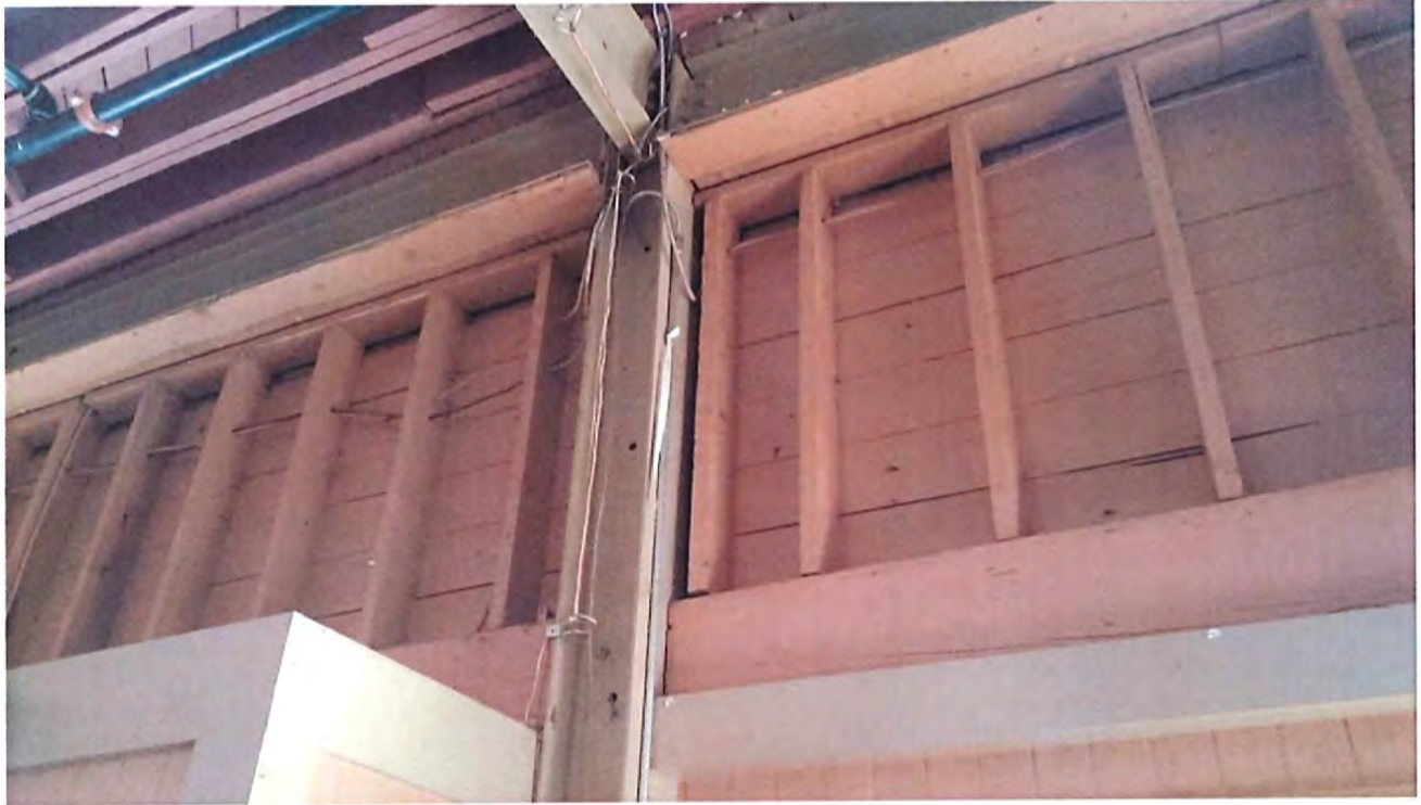
Interior view of wood awning/storefront at central steel column
