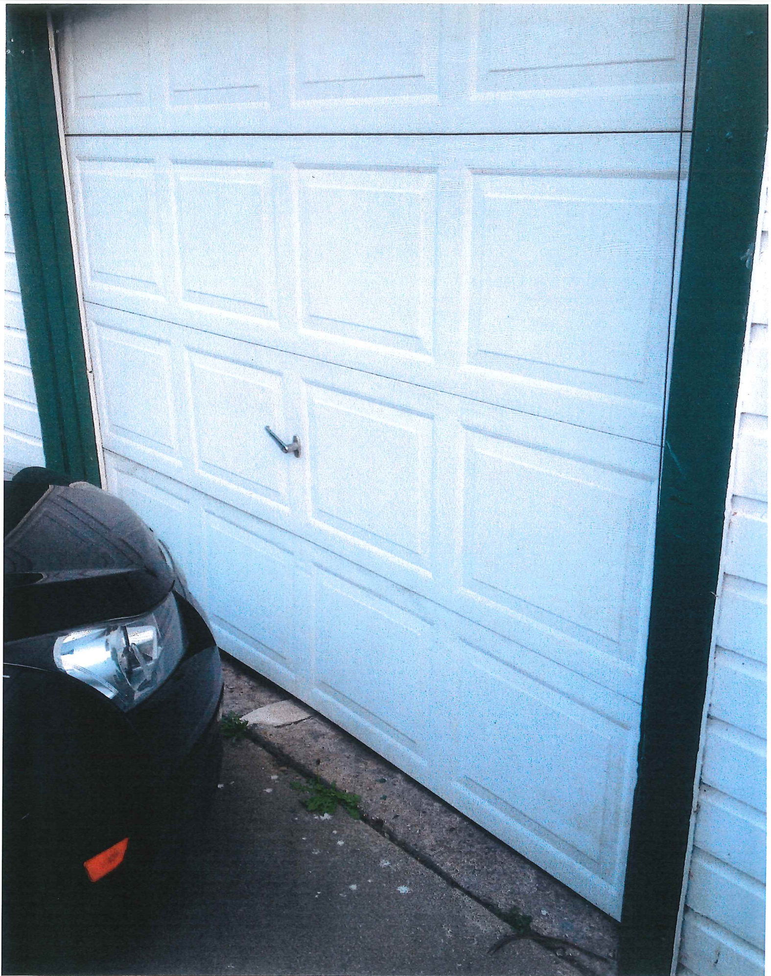
Existing garage door 228 n. River
