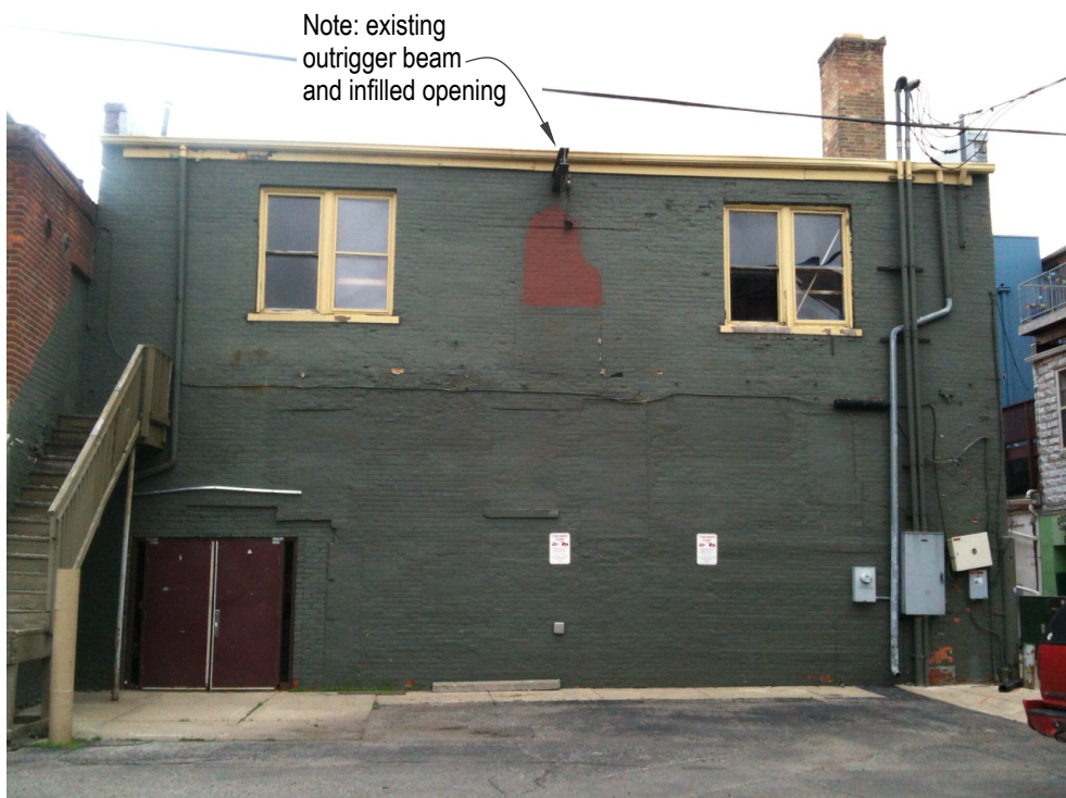
Existing back (west)
