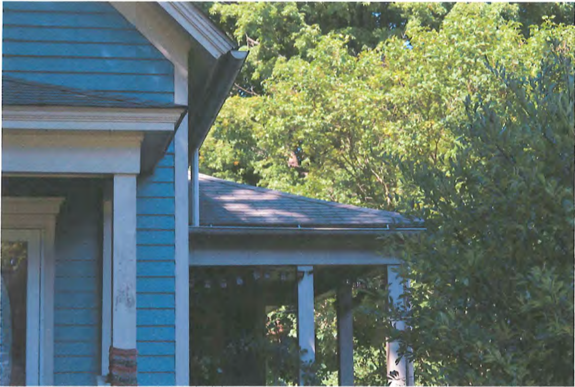
View of east side of house, looking N
