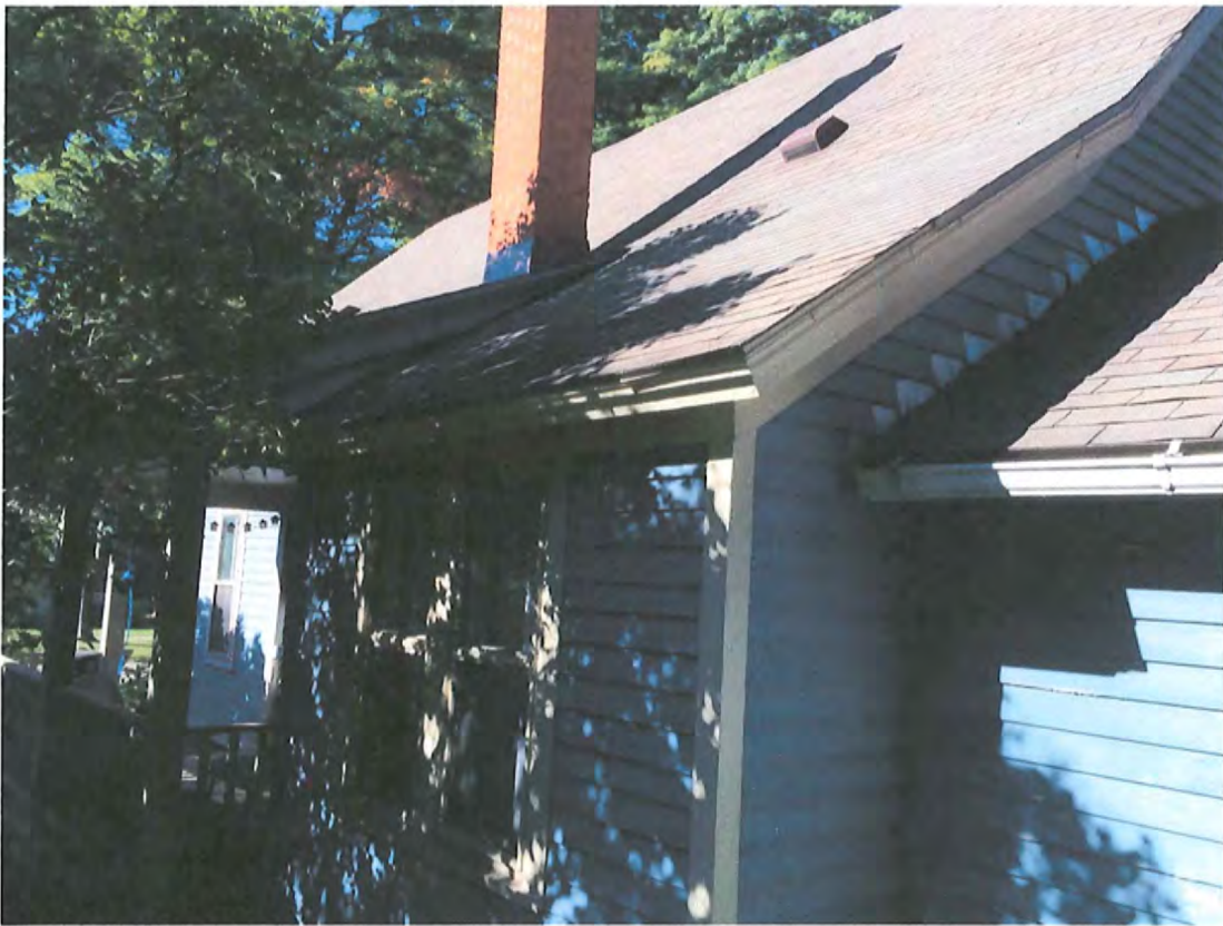
View of 2011 repair
