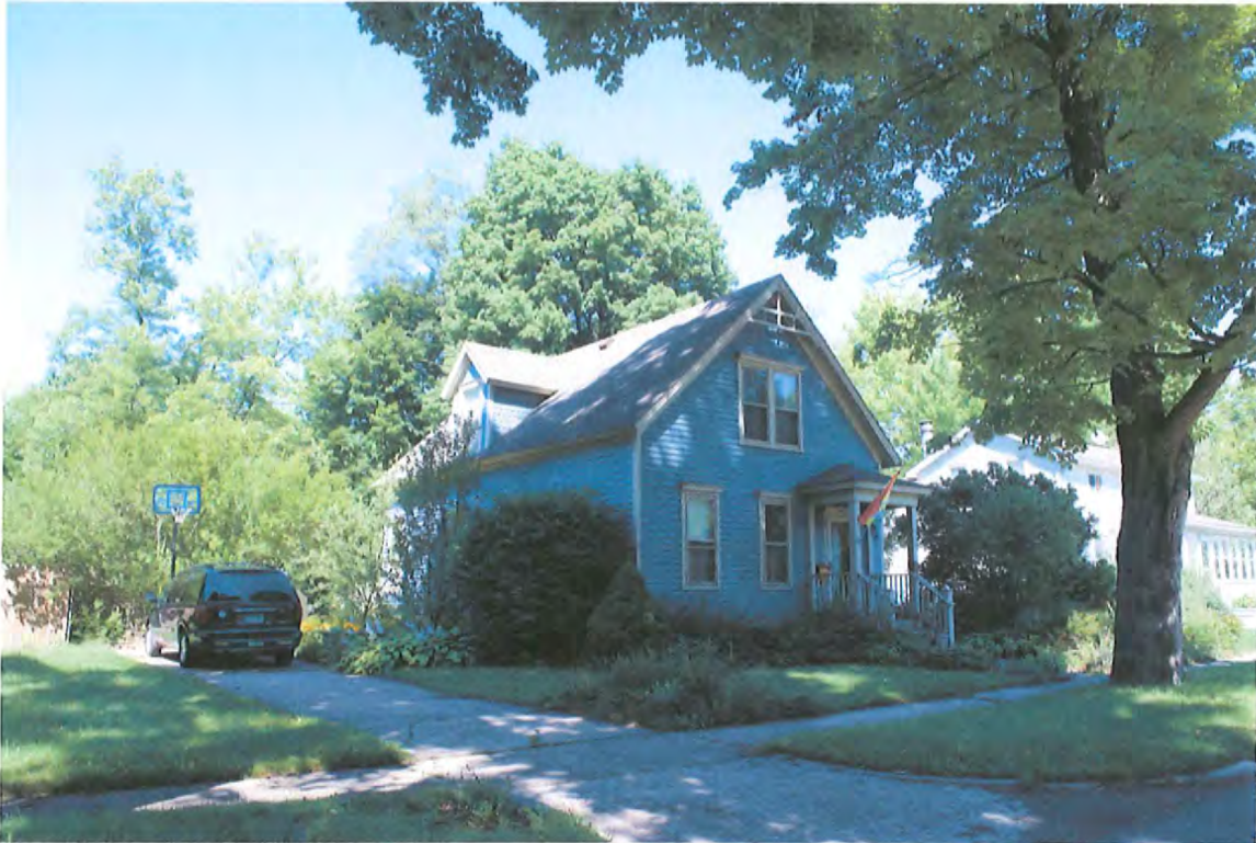
Front View looking NE
