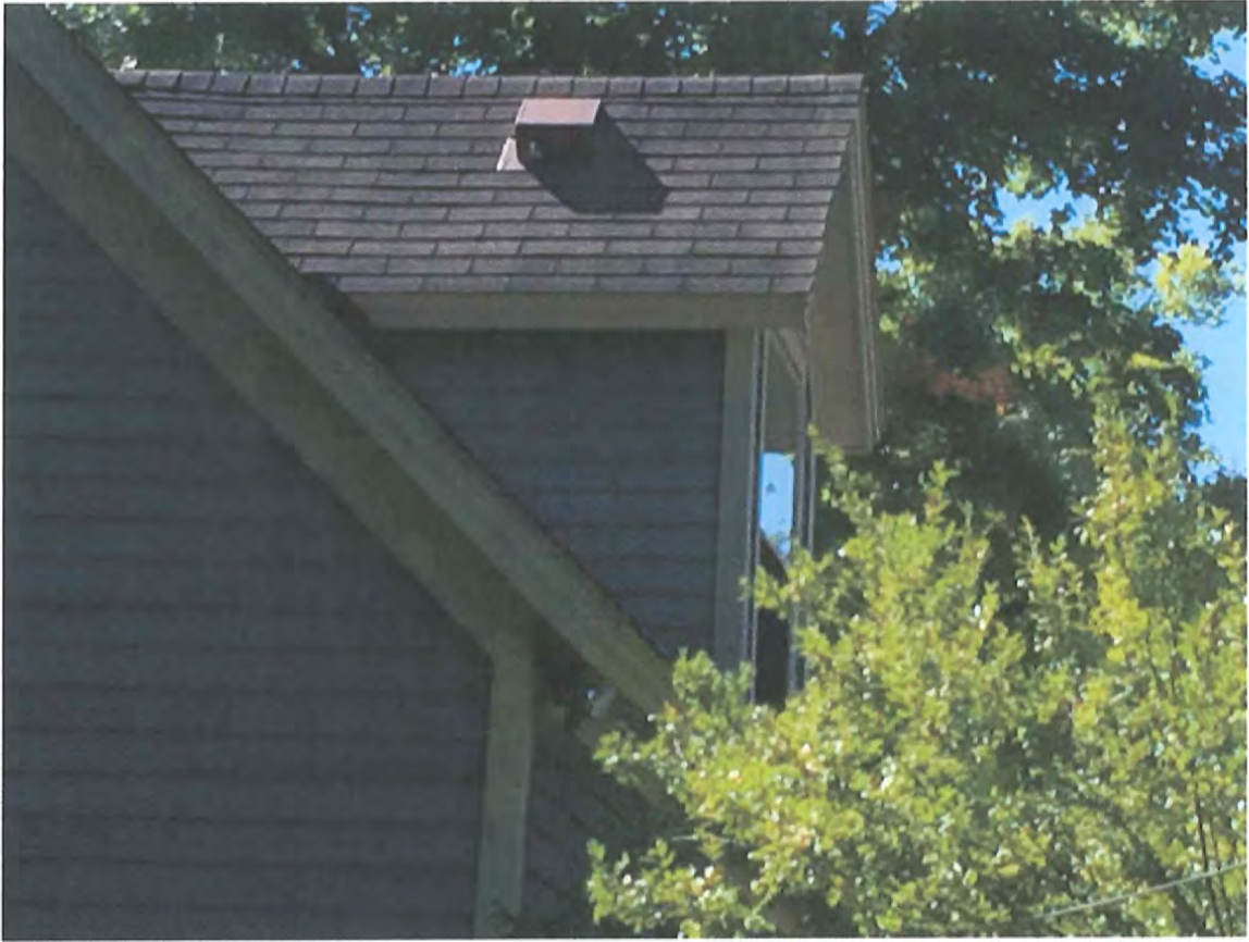
North Face of dormer
