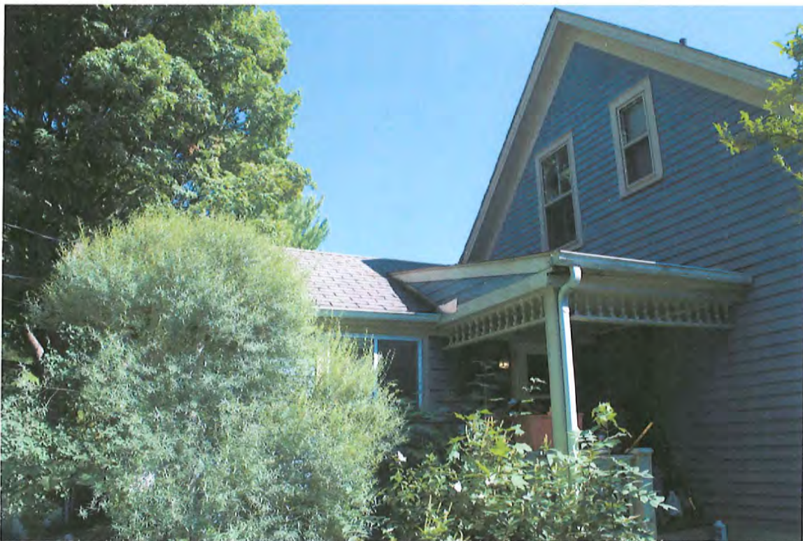
Rear View Looking SE
