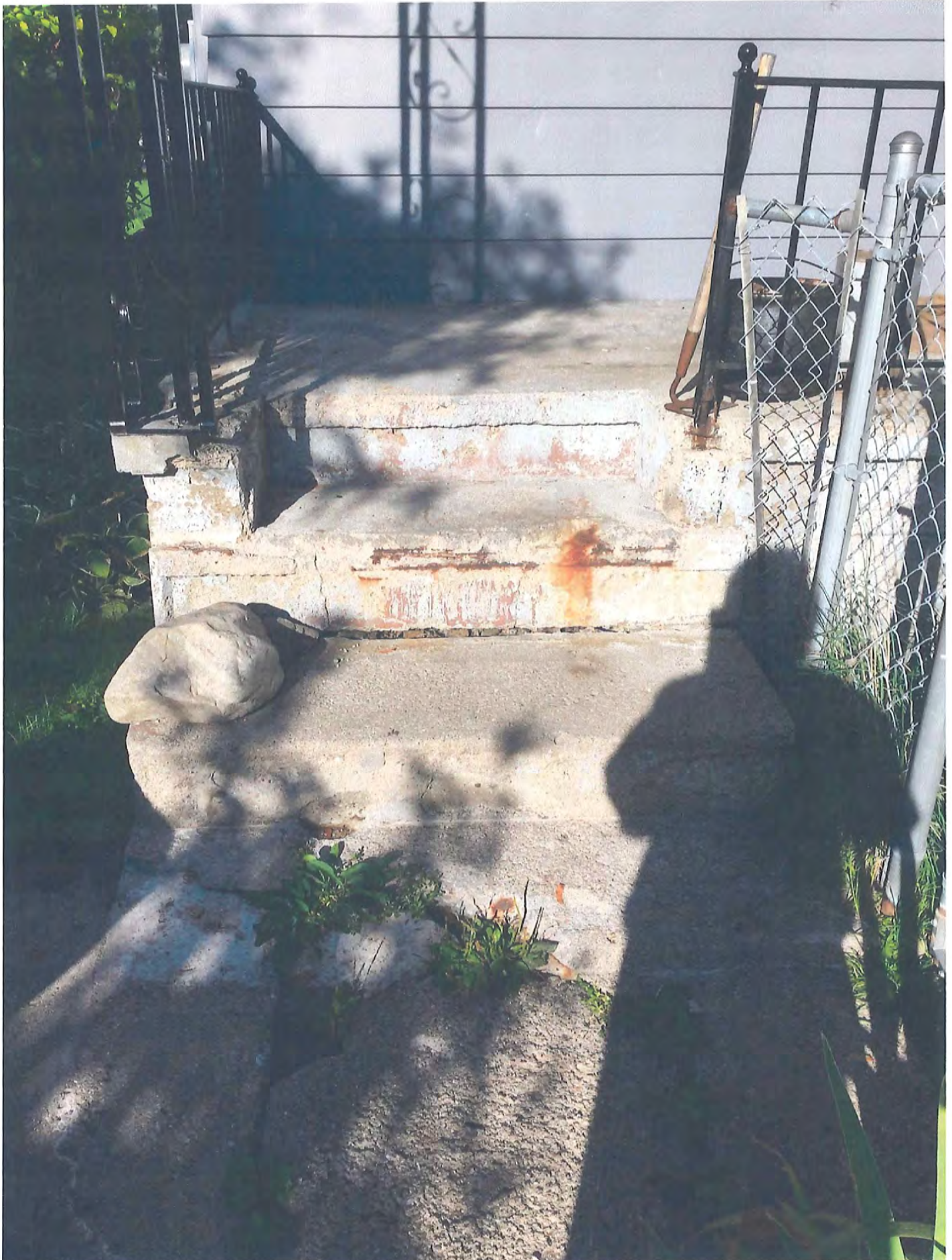
Current condition, Olive Street (rear) porch
