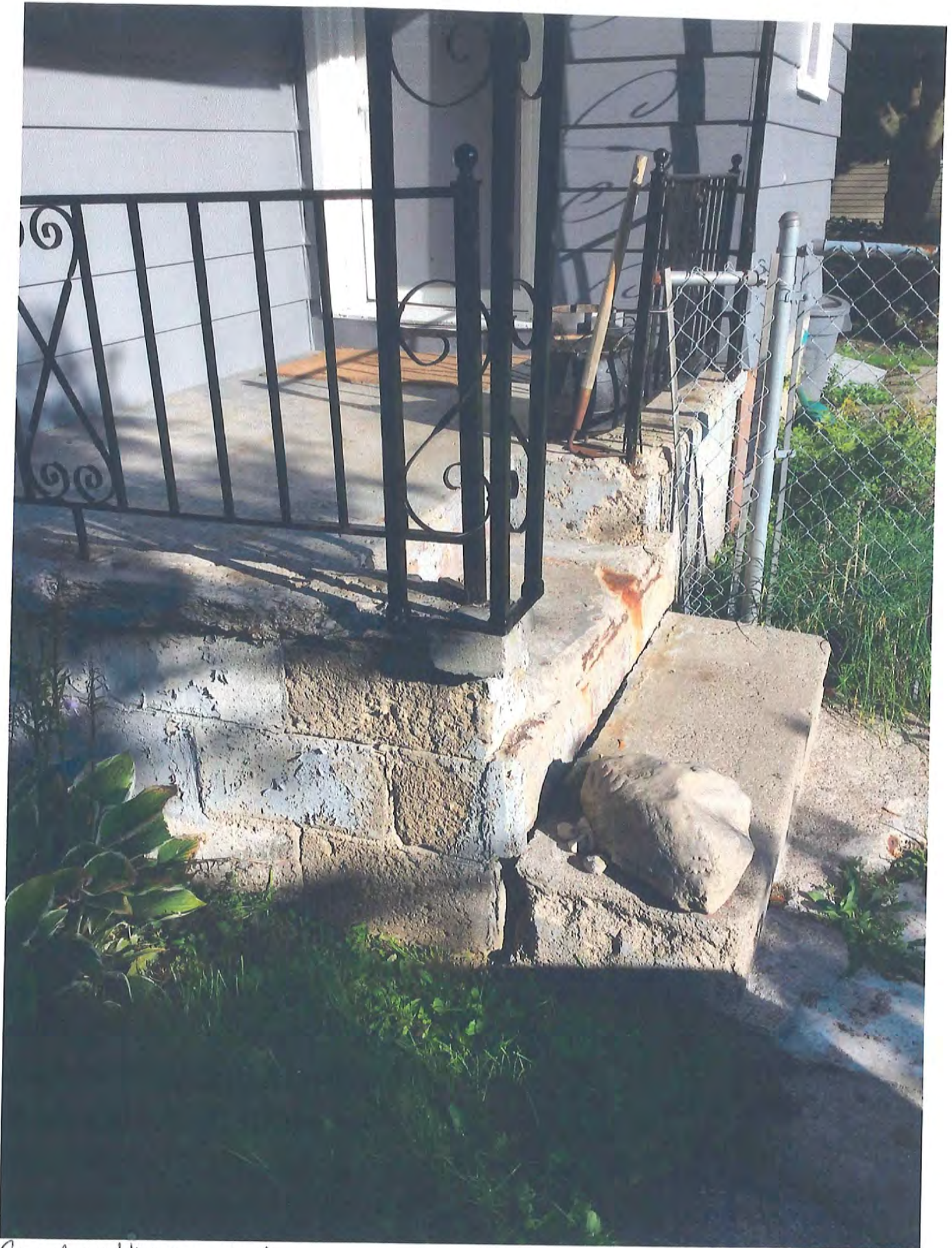
Current condition, rear porch
