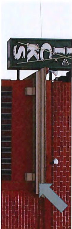
SW 7069 Iron Ore Interior / Exterior Locater Number 251-C7
