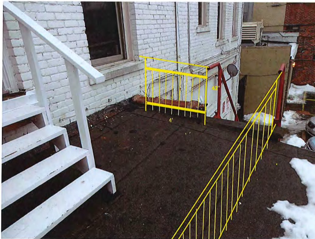
PROPOSED RAILS FOR APARTMENT #3 EMERGENCY EXIT
