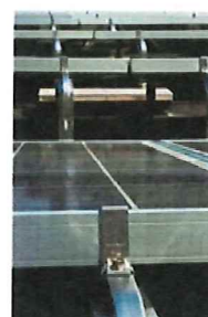
Panel Clamps with Integrated Grounding
