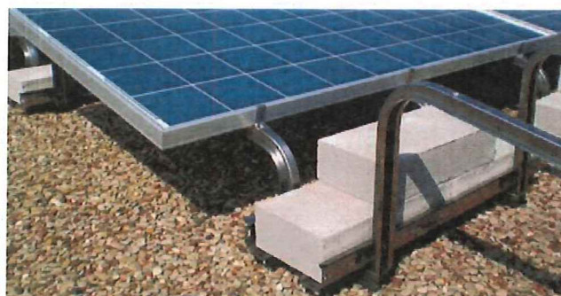
Panel Clamps with Integrated Grounding
