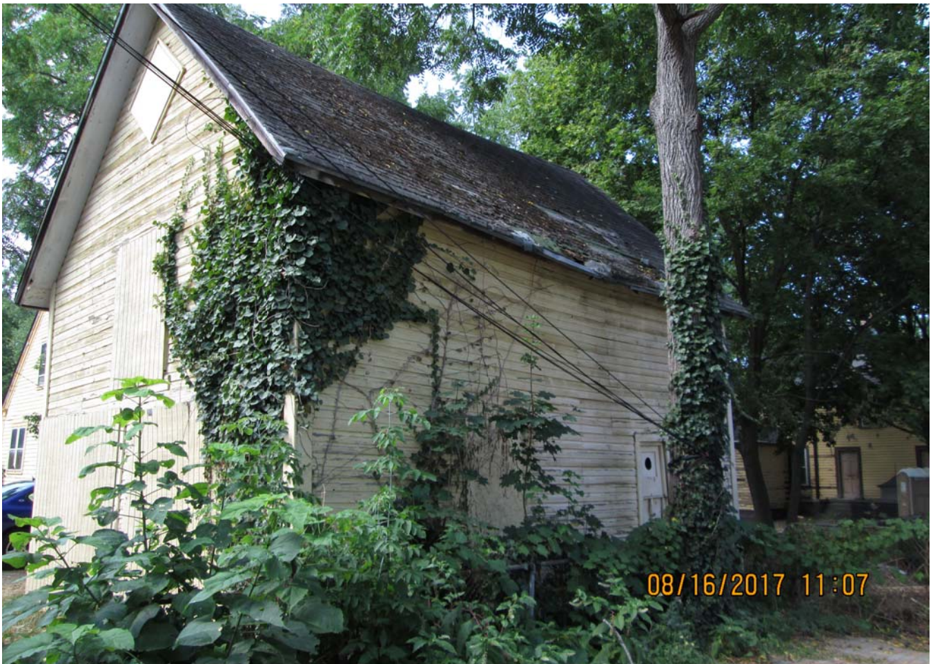
422 N Hamilton-outbuilding-north side
