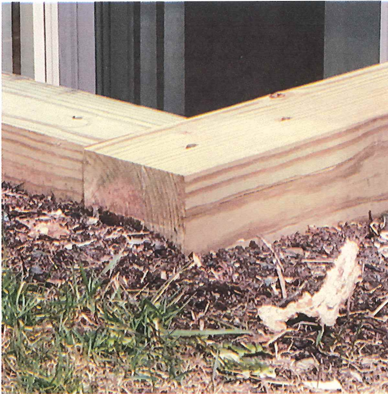
Proposed treated 6x6 window well.
