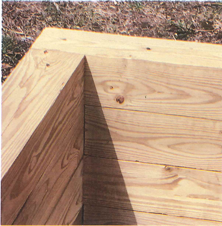
Proposed treated 6x6 window well.
