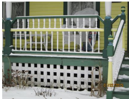
This is an example of an approved way to bring the porch railing up to code.
