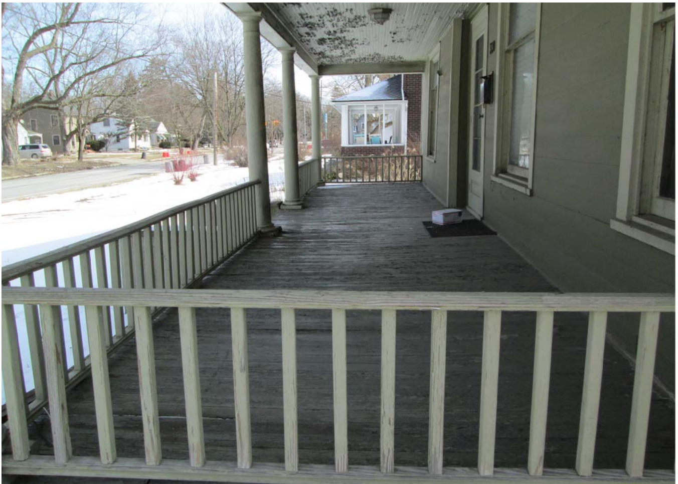
330 E Forest, Porch Detail, Facing East
