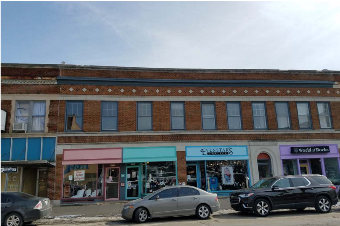
32-42 N Huron, facing east to facade, showing full parapet.
