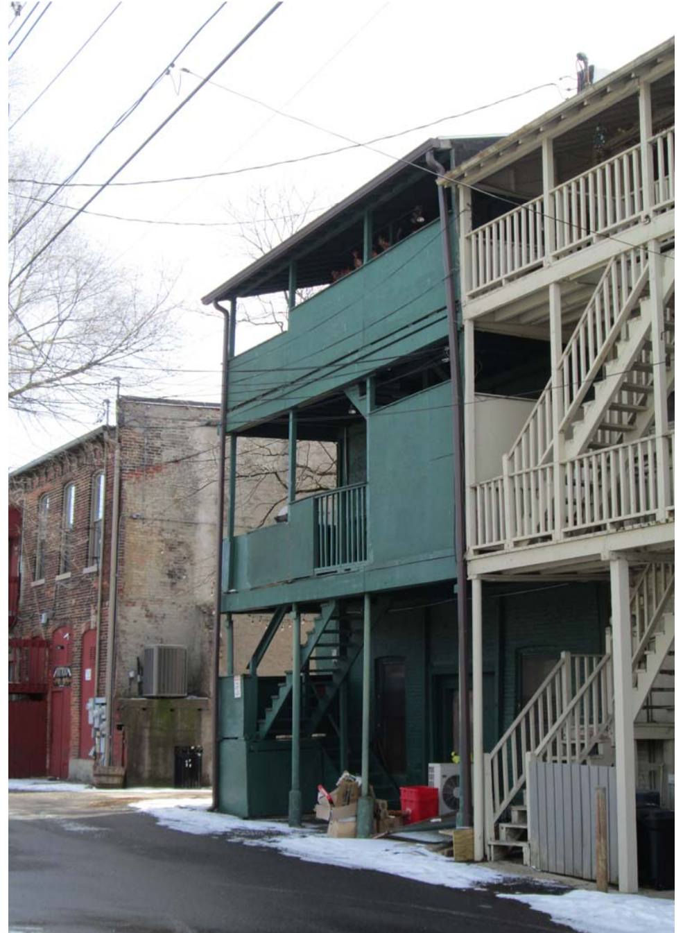
29 E Cross, Facing Southeast to North Elevation
