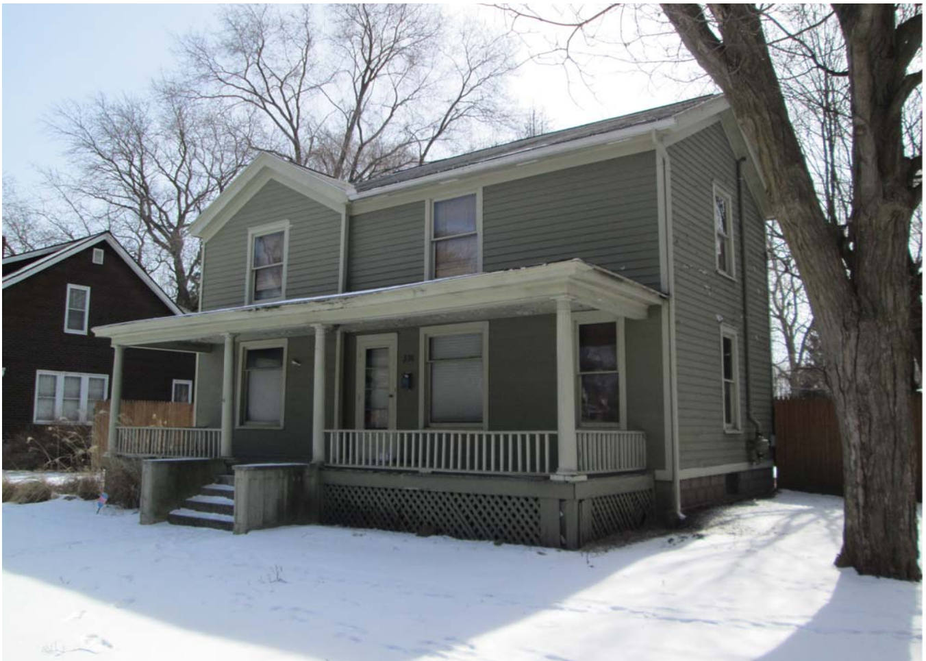
330 E Forest, Facing Southwest to Facade and West Elevation
