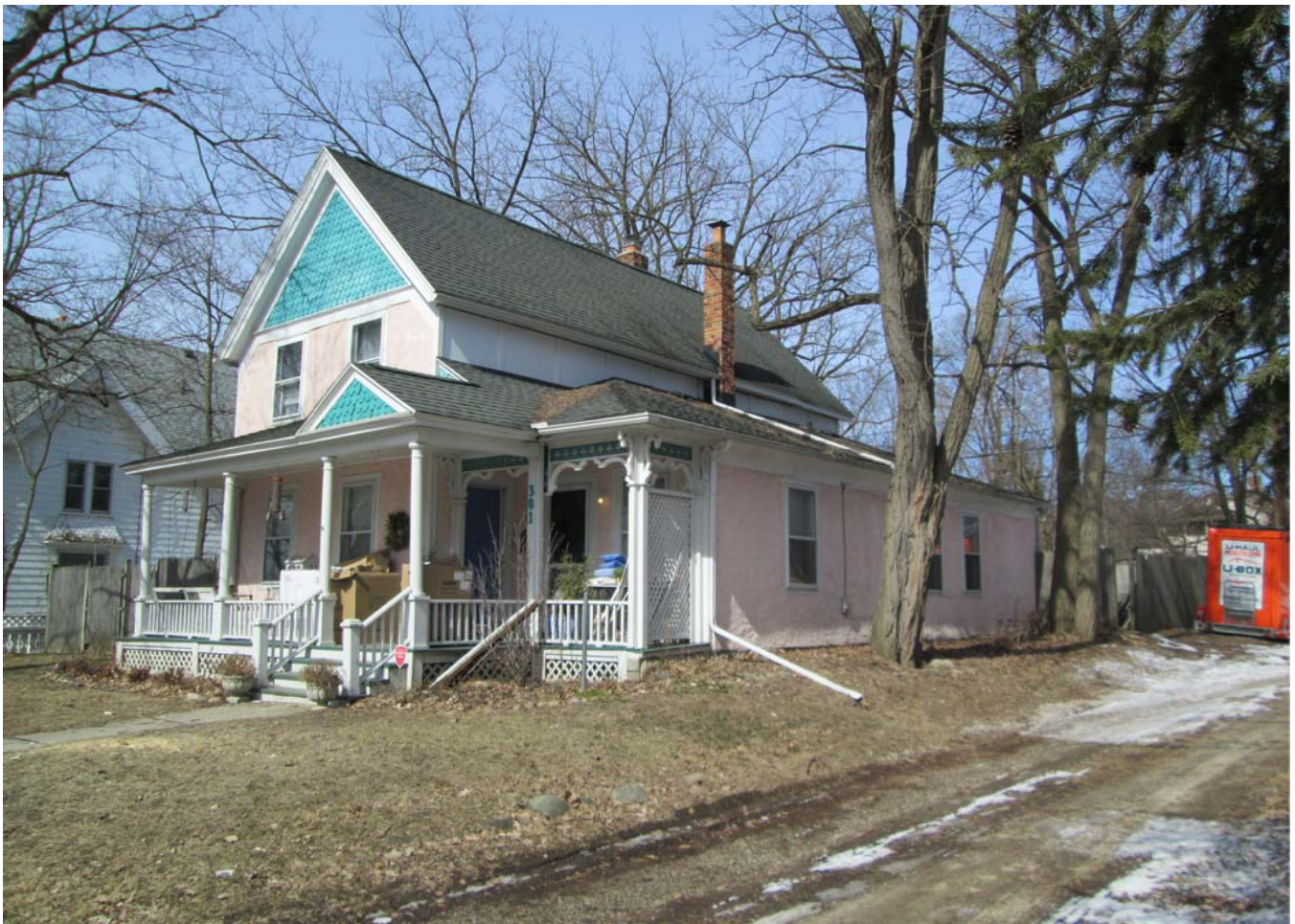
301 Maple Street, Facing Northwest to View of Facade and East Elevation from Sidewalk
