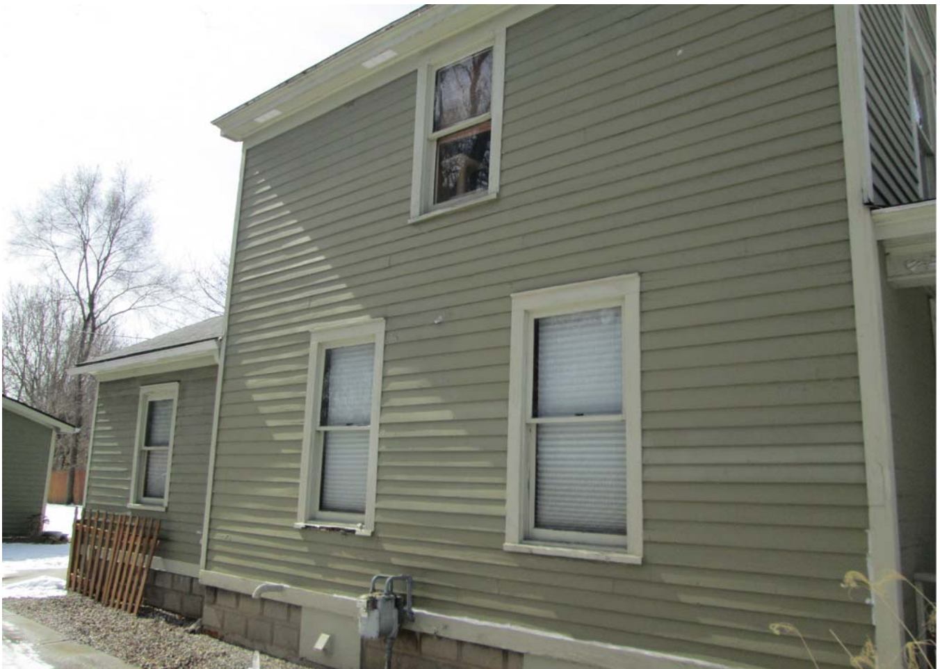
330 E Forest, Facing Southwest to Detail of Windows on West Elevation
