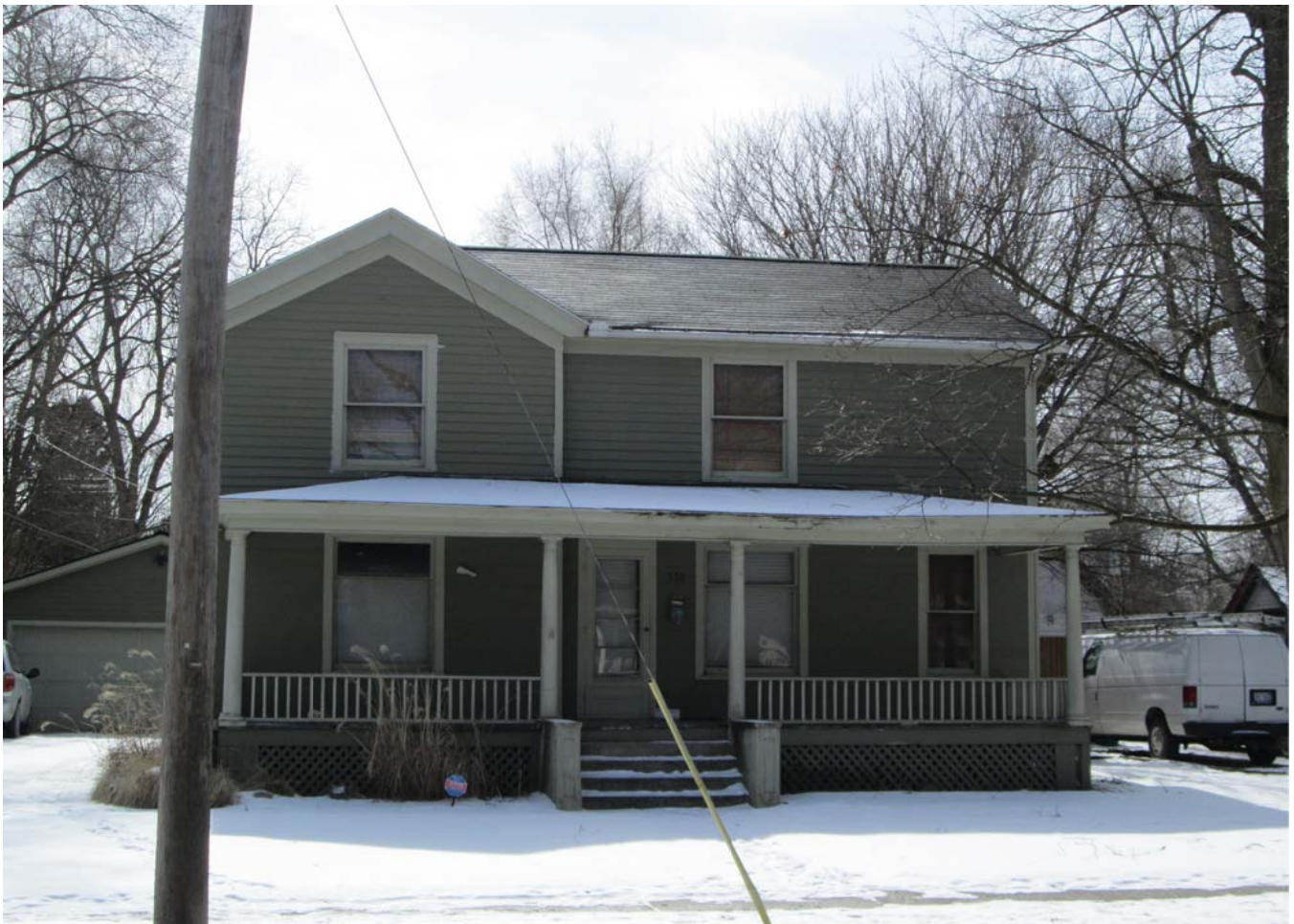
330 E Forest, Facing South to Facade
