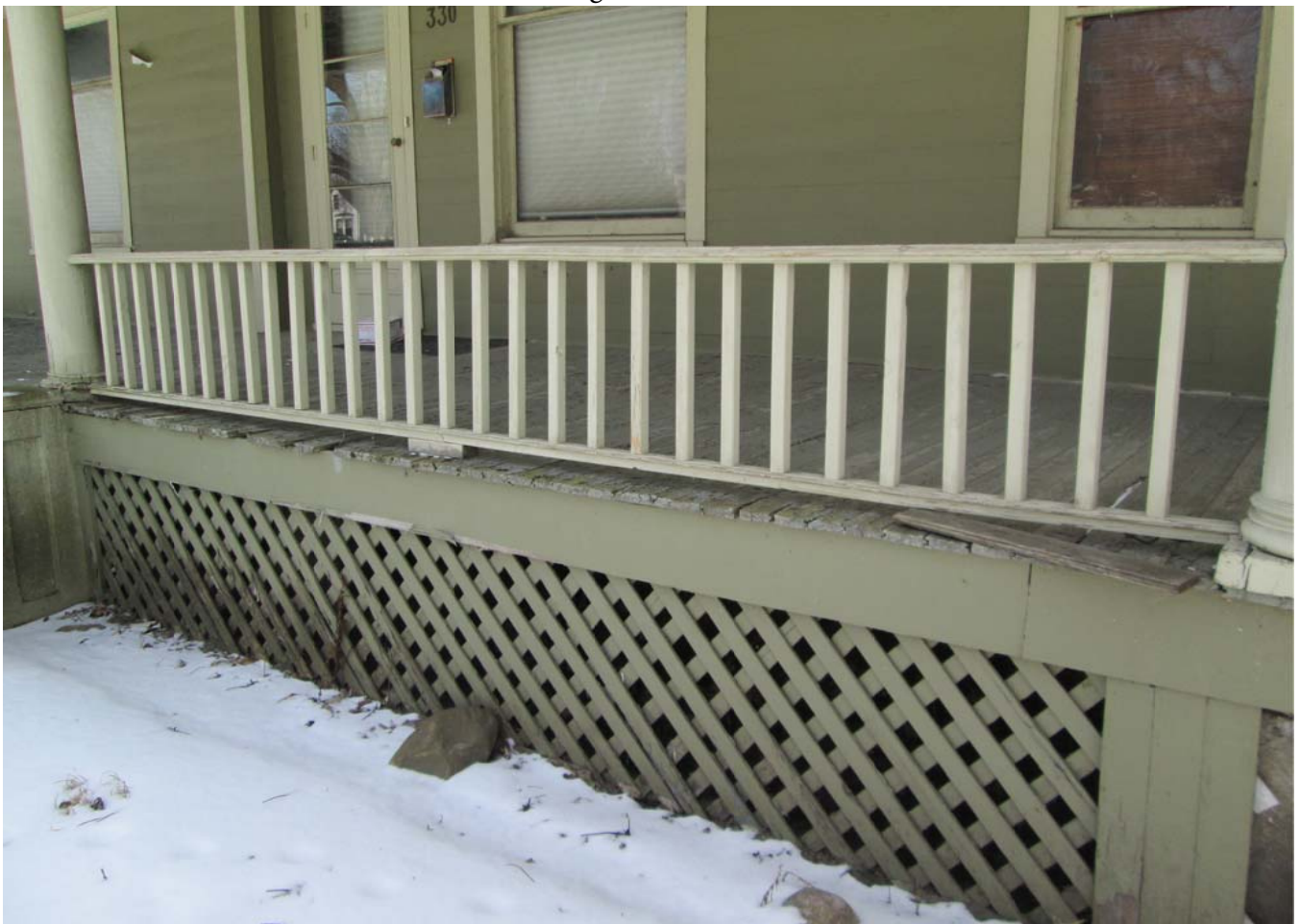
330 E Forest, Porch Detail. Facing Southeast
