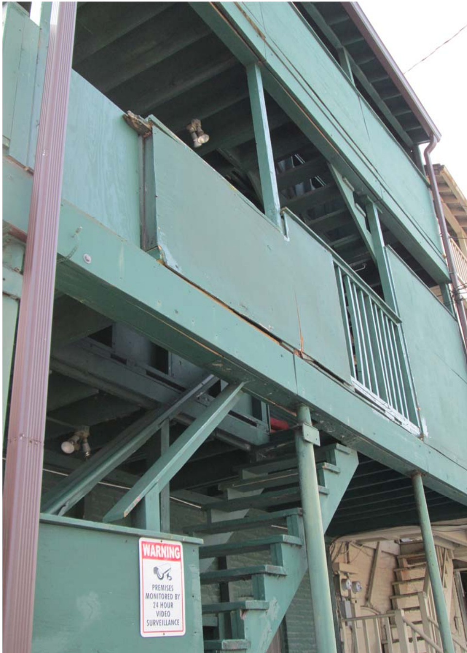
29 E Cross Street, Facing Southwest to Staricase Detail
