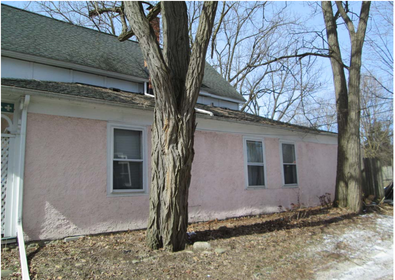
301 Maple Street, Facing Northwest to East Elevation. Proposed New Window Location at Center
