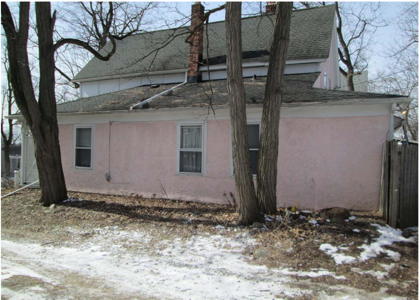
301 Maple Street, Facing West-Southwest to East Elevation. Proposed New Window Location Left of Center
