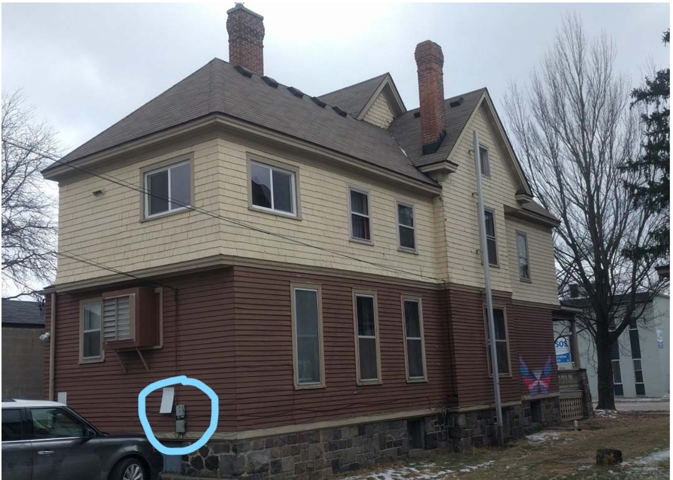
104 S Huron, Facing Northeast to South and West Elevations. Location of Solar Inverter Circled in Blue
