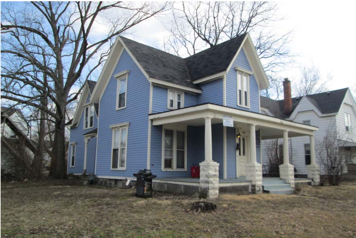
520 N Hamilton, Facing Southeast to Facade and North Elevation
