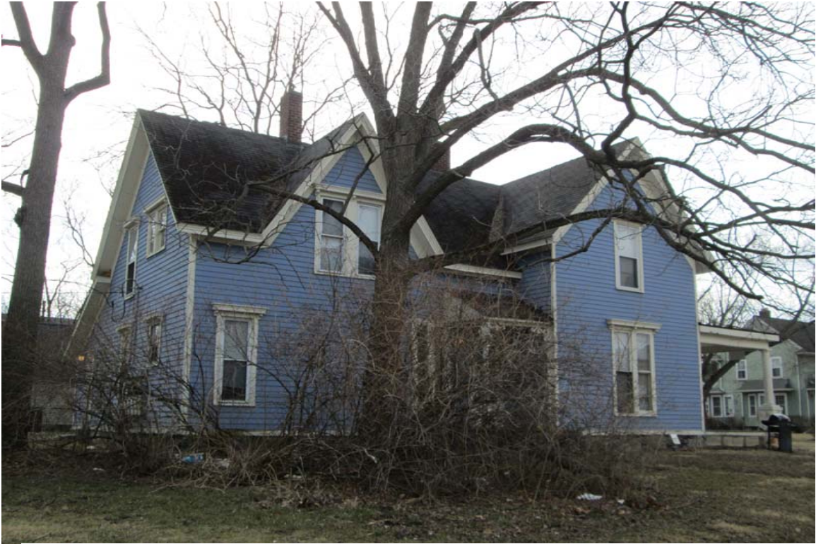
520 N Hamilton, Facing Southwest to North and West Elevations
