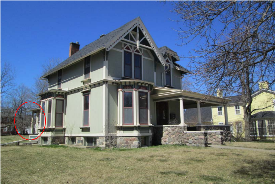
View to porch from right-of-way, facing northwest to facade and south elevation
