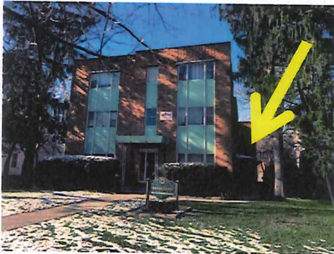
Front view from sidewalk
