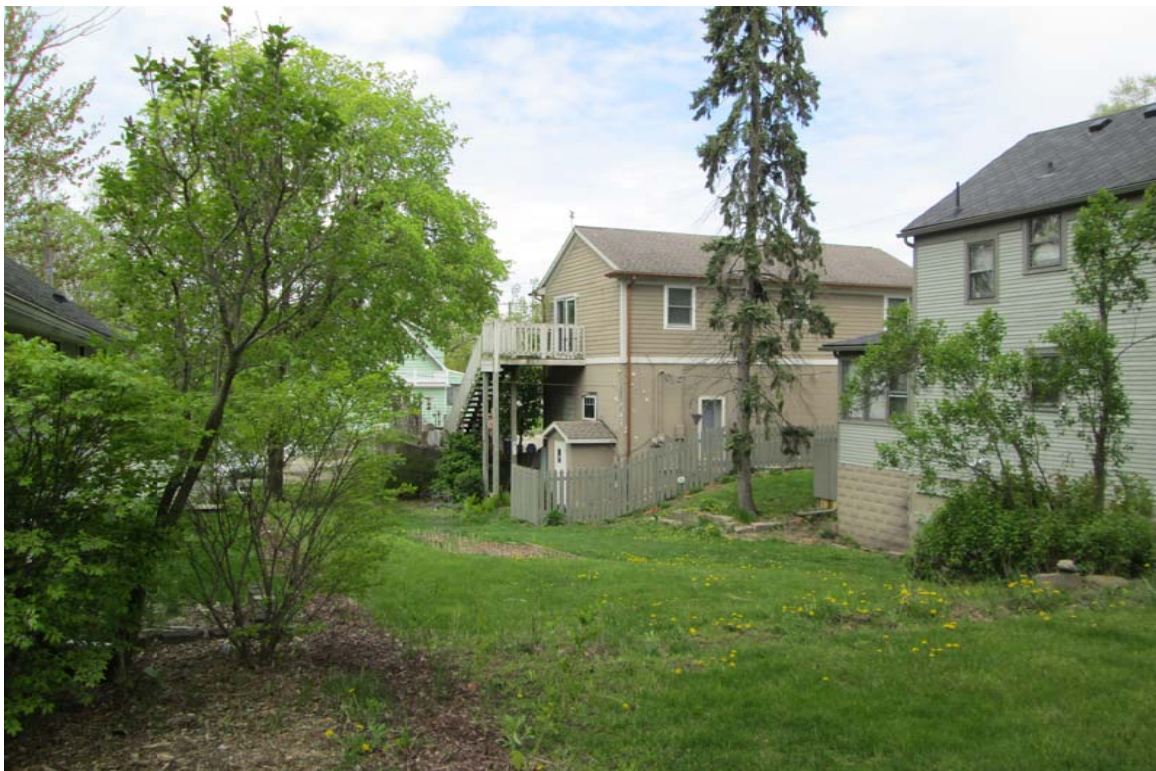
Facing northwest to west property line, view to the fence that is to be extended.
