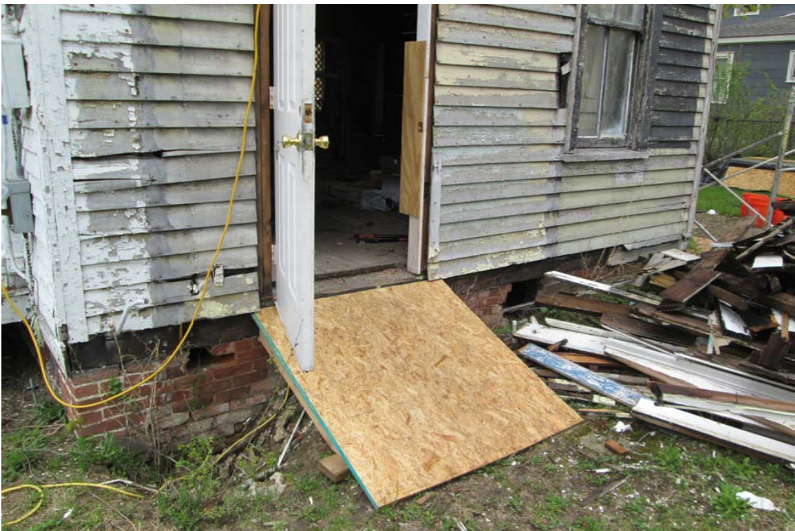
Looking north-northeast to south foundation wall or rear ell
