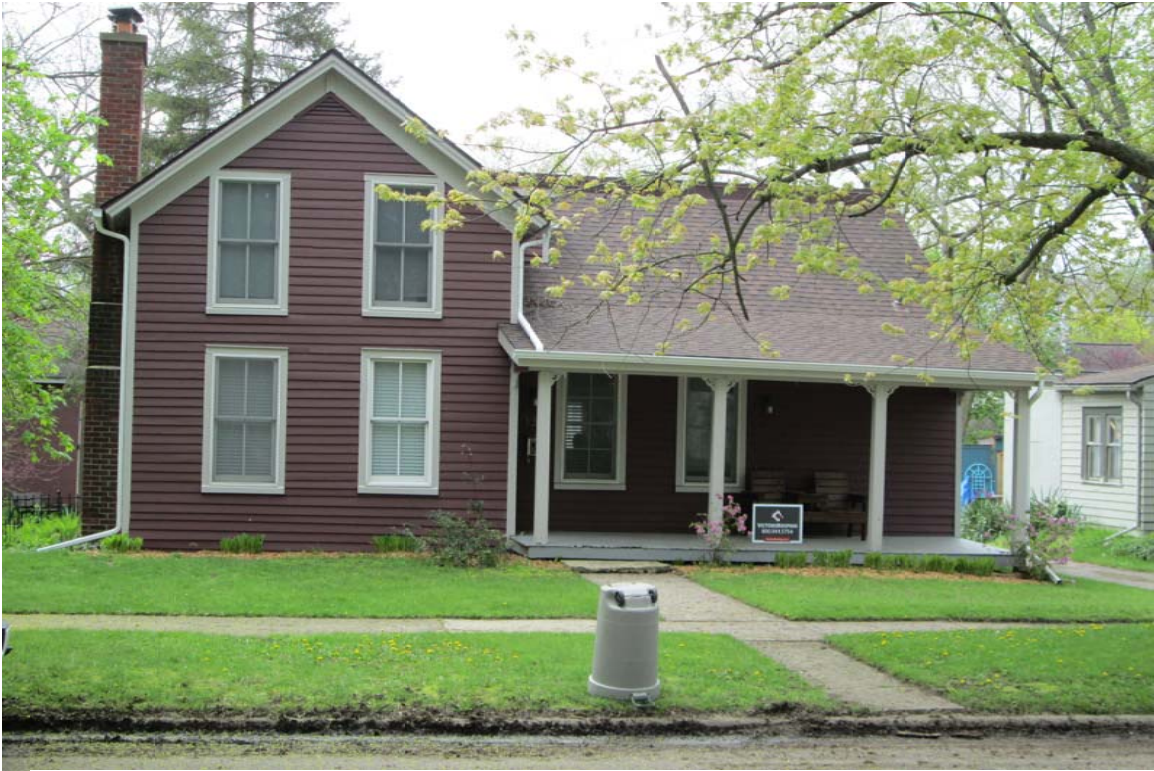
Facing south to house- Roof not being replaced, photo provided for reference.
