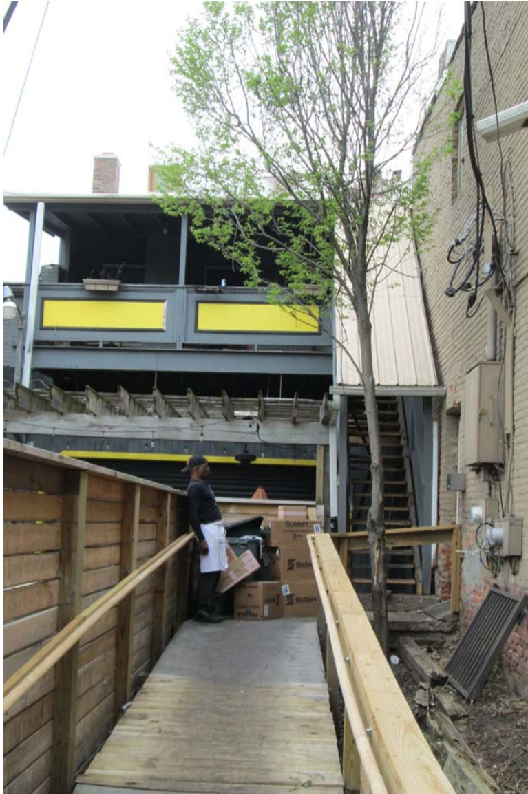
Facing north to stairs to be replaced on south elevation.
