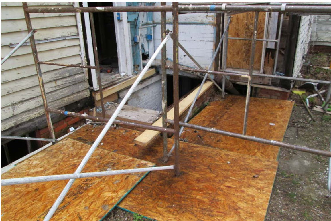
Looking northwest to east foundation wall of rear ell and south foundation wall of the house
