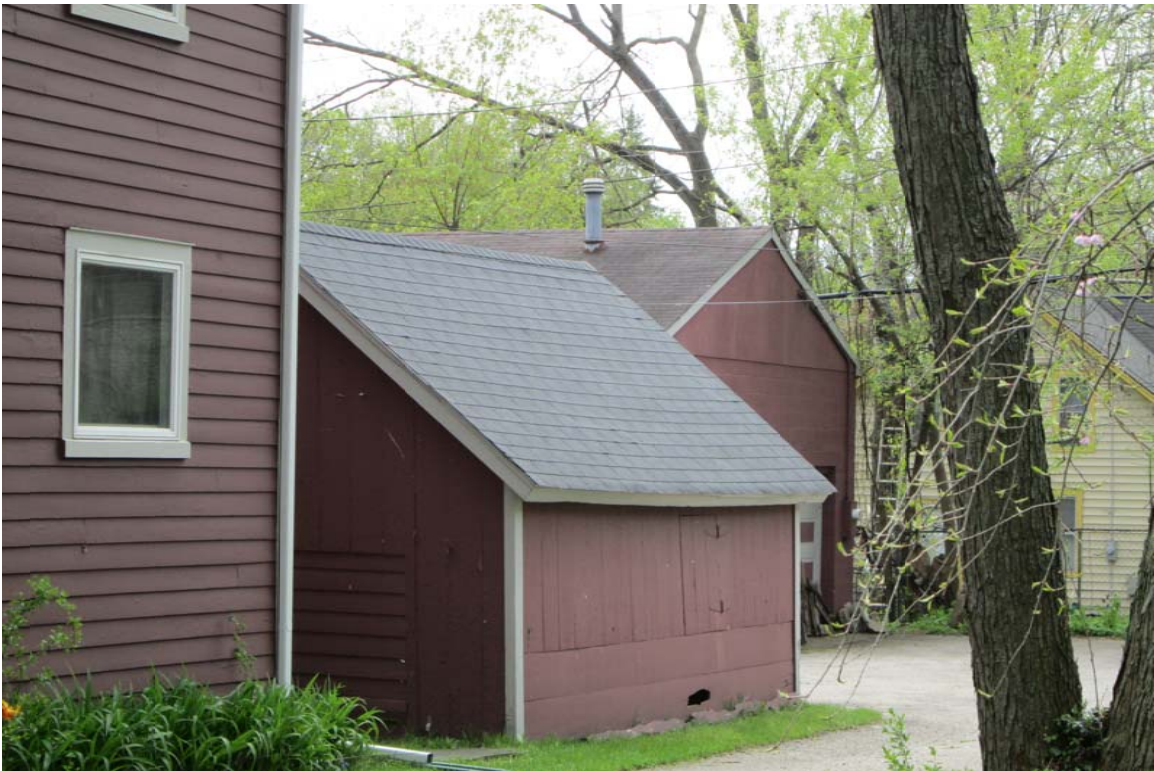
Facing southeast to garages with roofs to be replaced (behind house).
