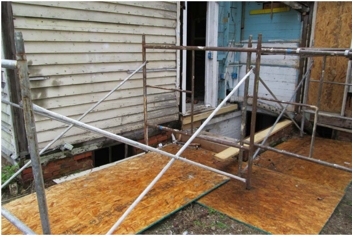
Looking northwest to east foundation wall of rear ell
