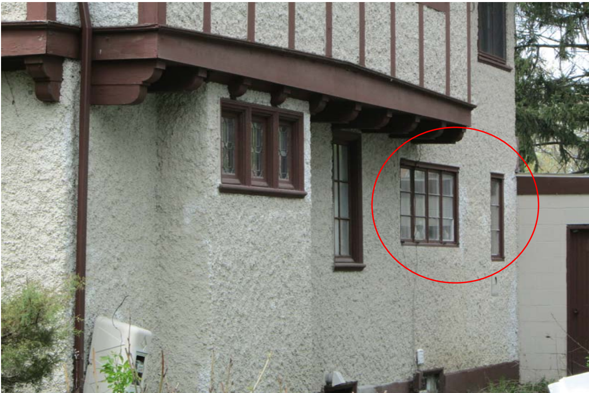
Detail of casement windows on north elevation proposed for replacement.
