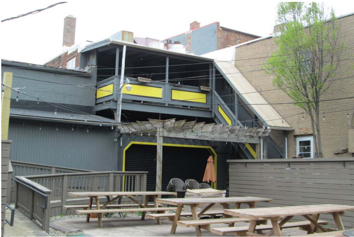
Facing northeast to stairs on south elevation and chimney on west elevation.
