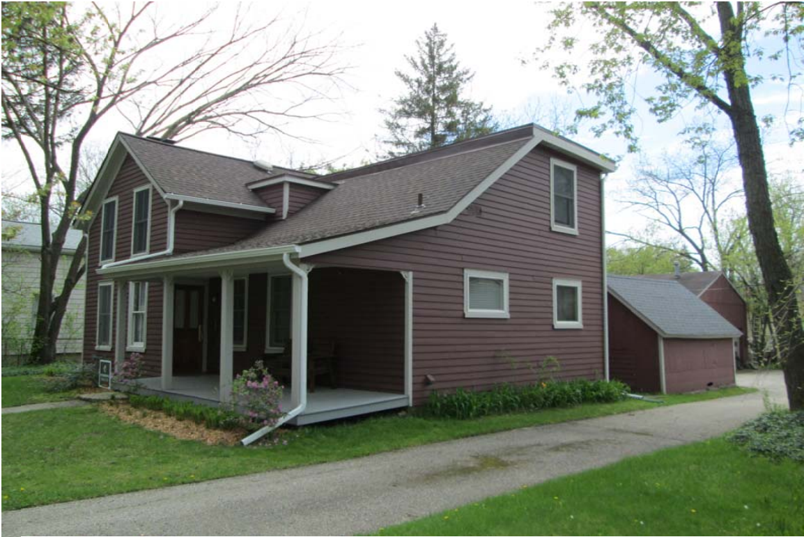
Facing southeast to house and garages.
