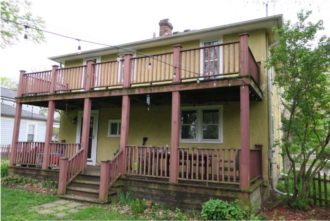
Facing northwest to south and east elevations.
