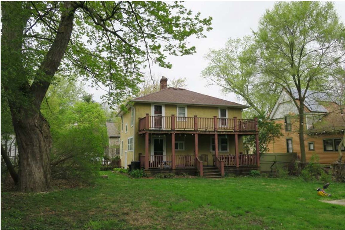
Facing northeast to south and west elevations.
