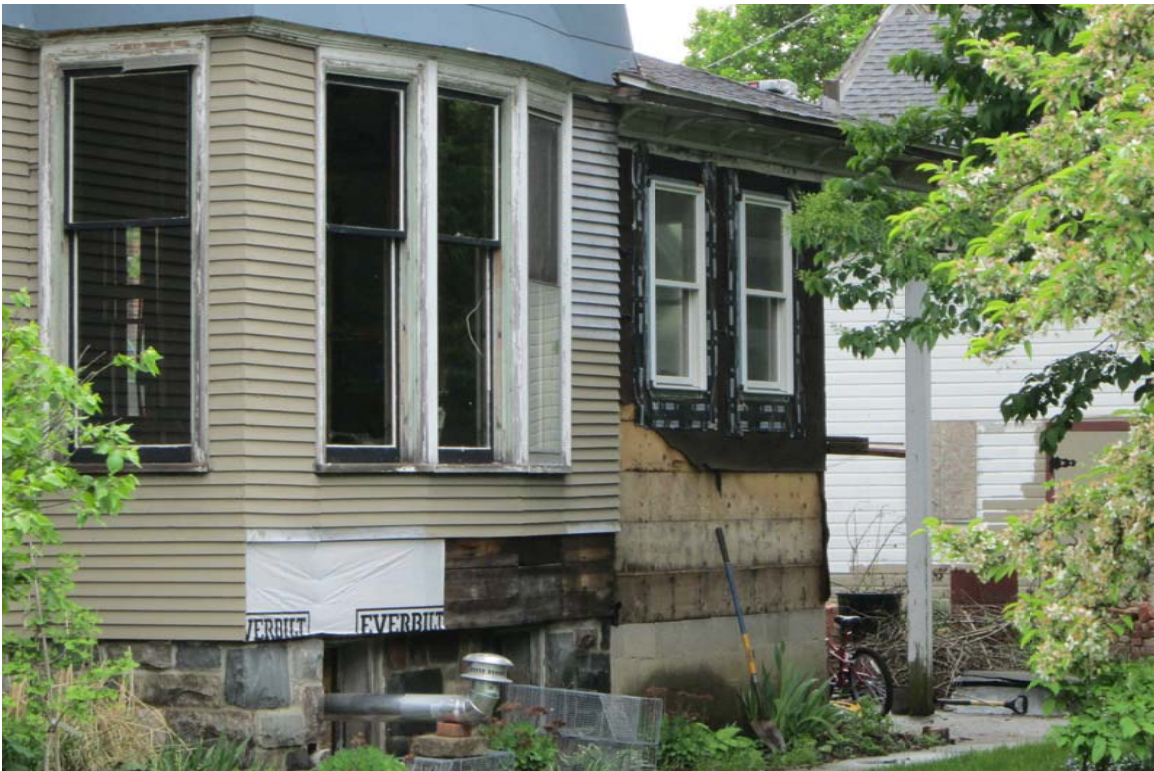
Facing northeast to replacement windows on south elevation.
