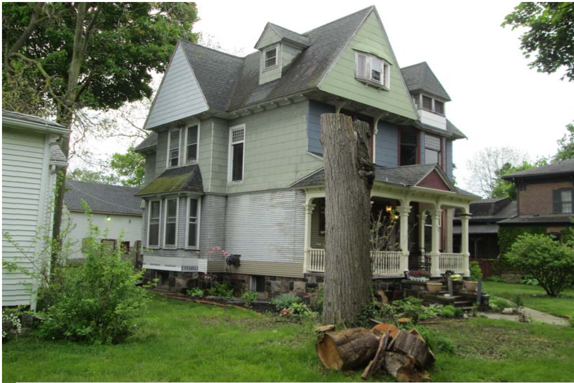
Facing southeast to facade and north elevation.
