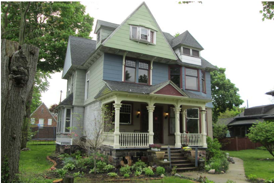
Facing southeast to facade and north elevation
