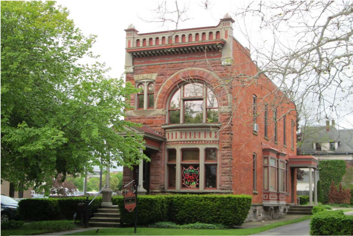
Facing southwest to facade and north elevation (for reference).
