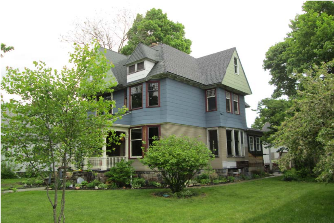
Facing northeast to facade and south elevation
