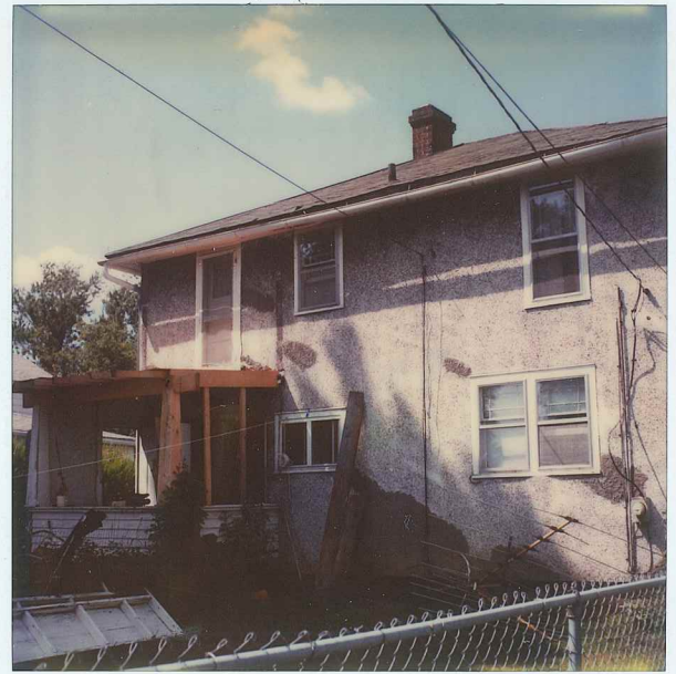
322 E Cross, August 1983, showing original south elevation
