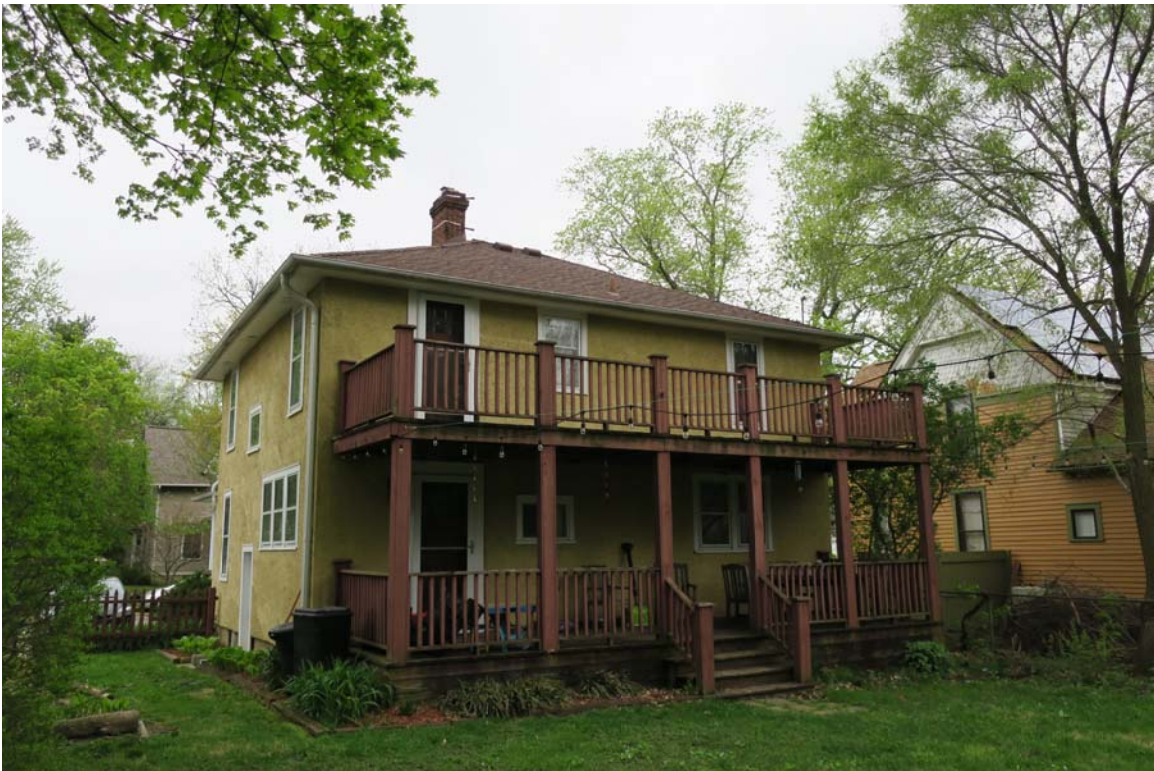
Facing northeast to west and south elevations, showing porch to be removed.
