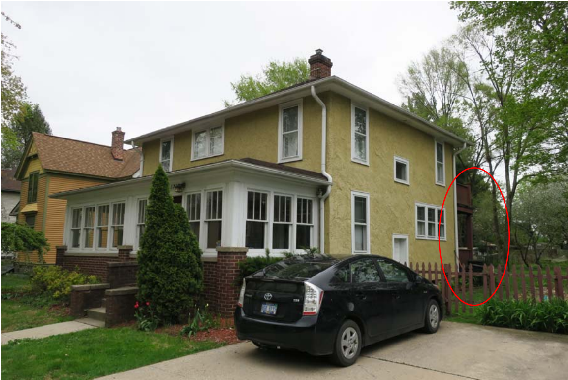
Facing southeast to Facade and west elevation- porch to be removed is on the rear of the house.
