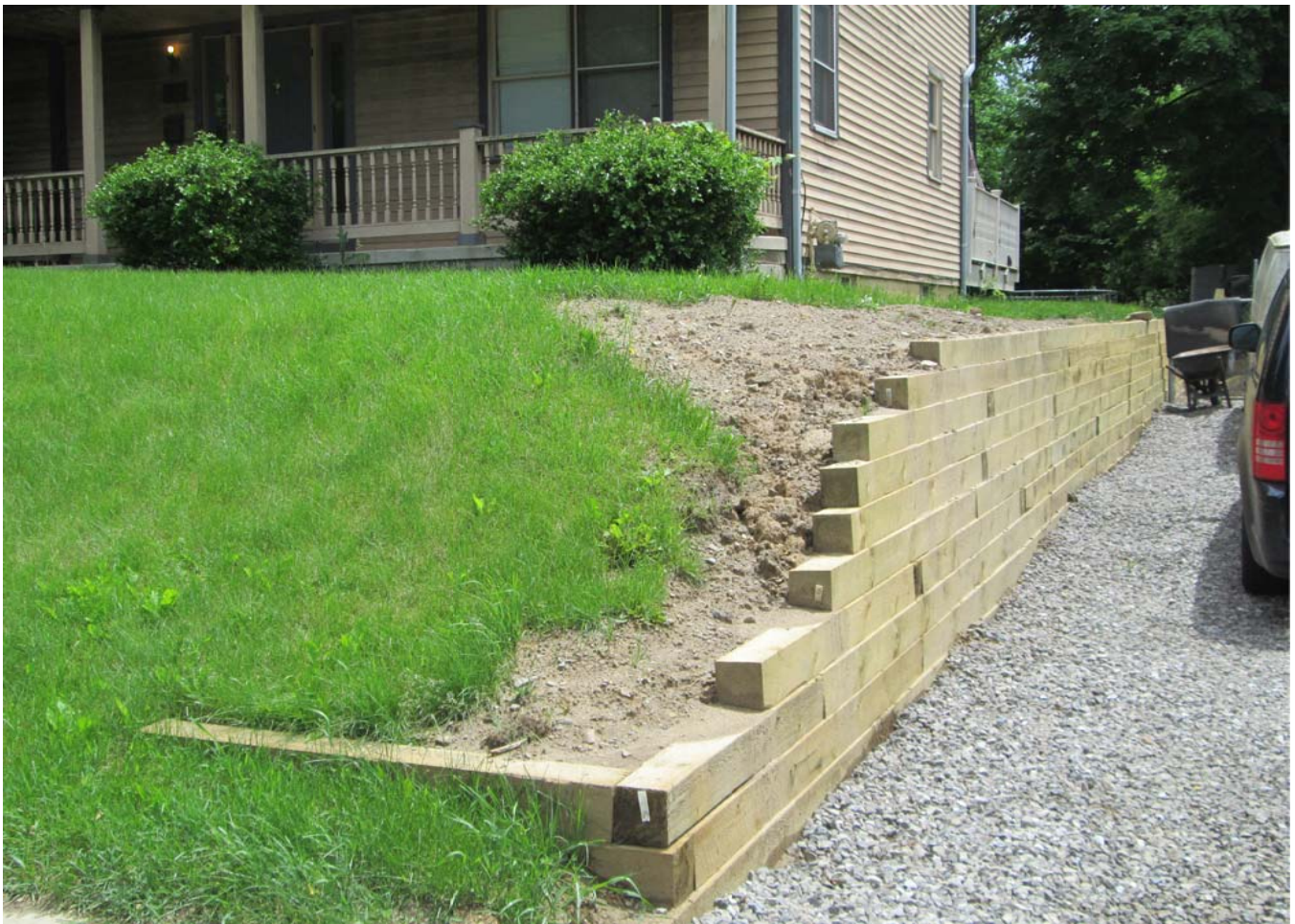
208 E Cross, facing southeast to new retaining wall.
