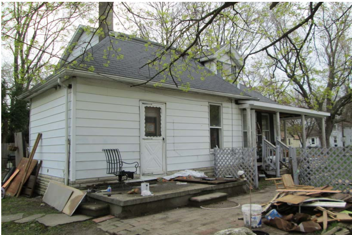
Facing southeast to west elevation.
