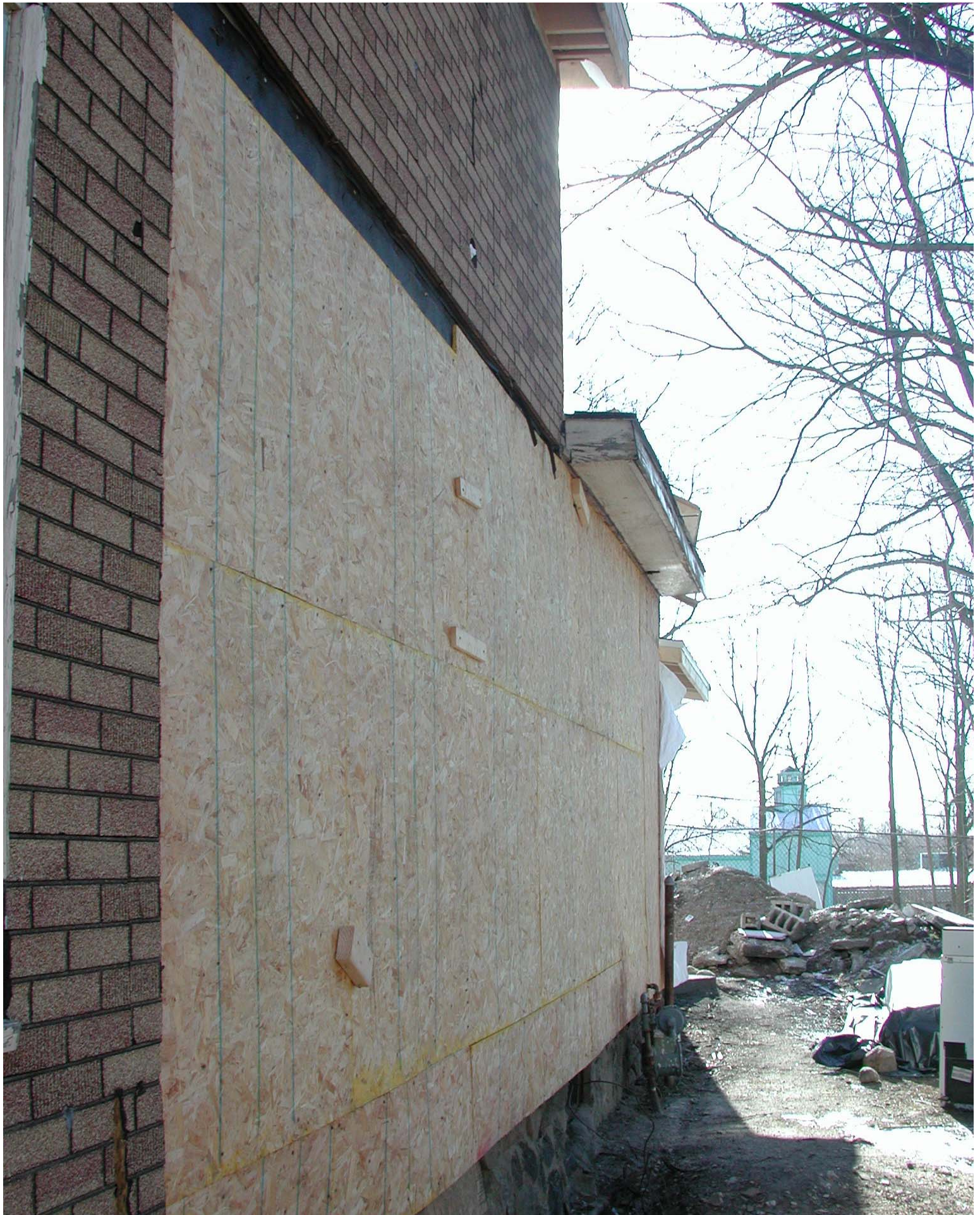
Photo showing former insulbrick siding being removed.
