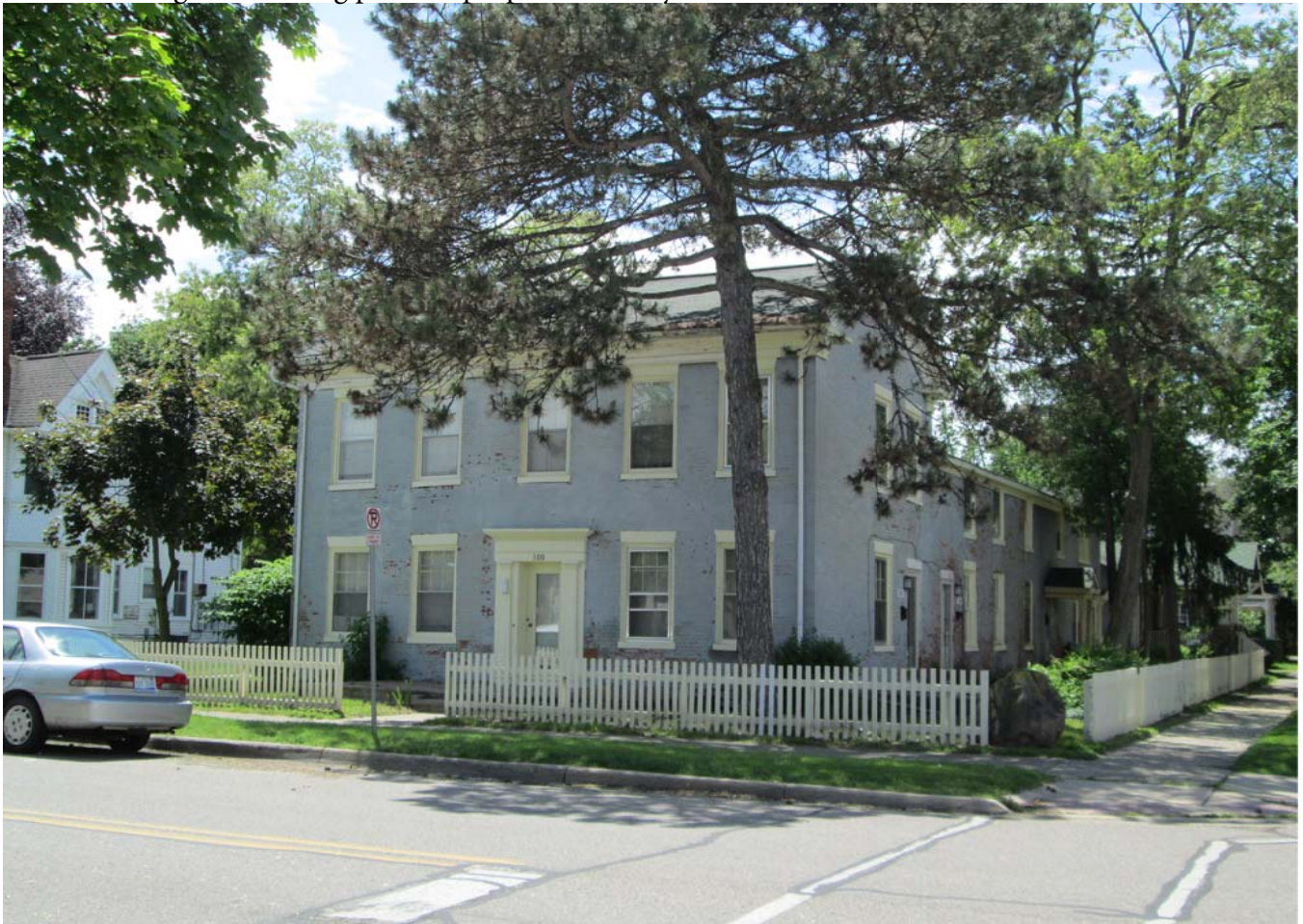
Facing southwest to facade and north elevation.
