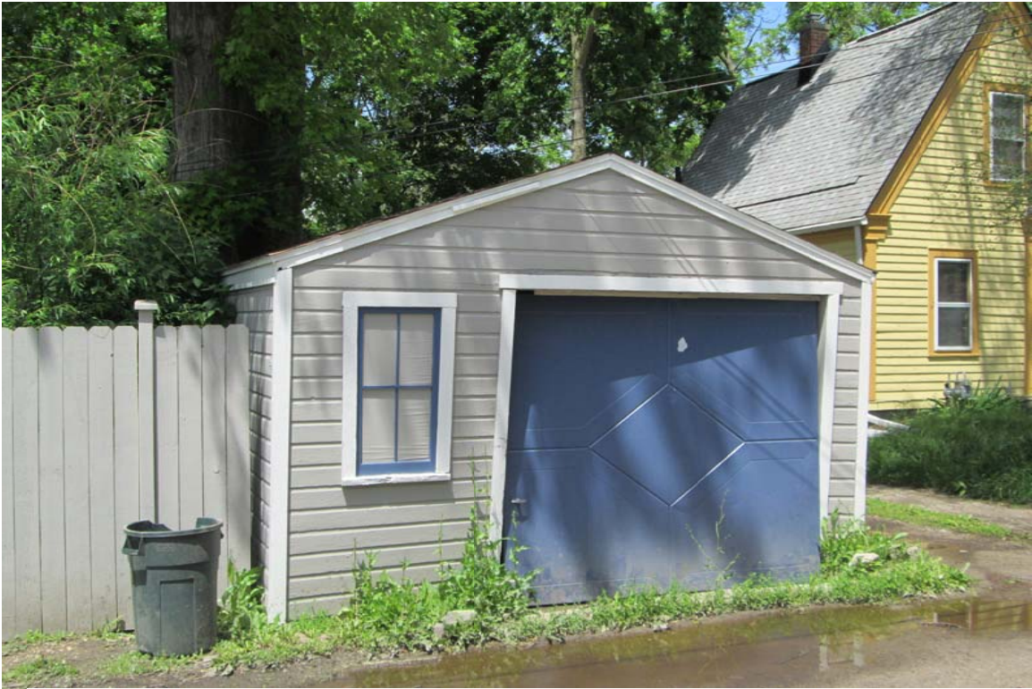
Facing north-northeast to south elevation of garage.
