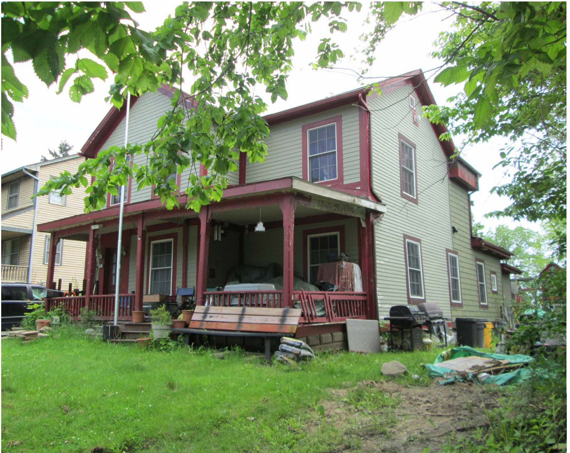
208 E Cross Street, facing southeast to facade and west elevation, showing siding change on west elevation.
