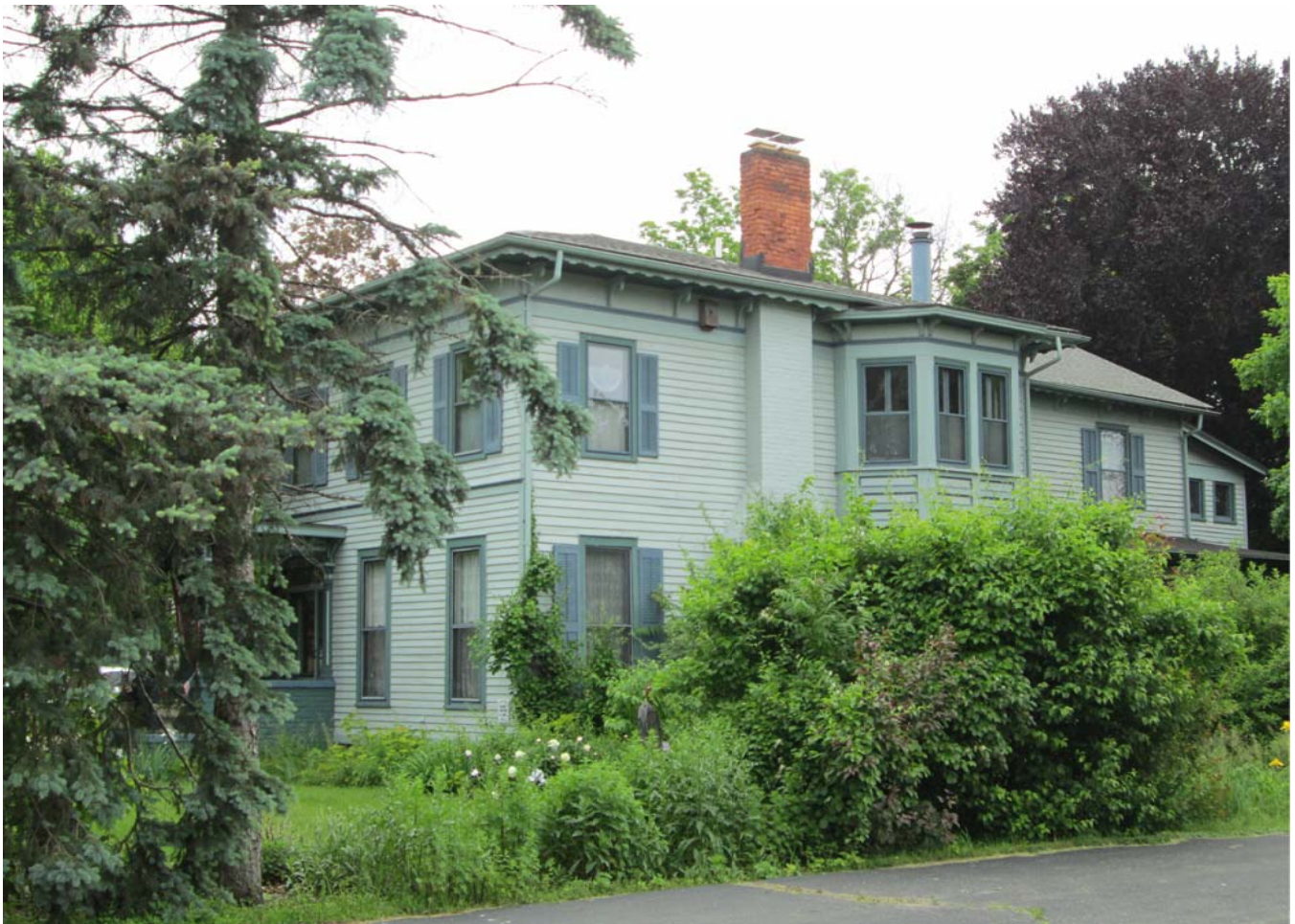
Staff photo, 214 N Huron, facing northeast to facade and south elevation. Chimney at center of photo.
