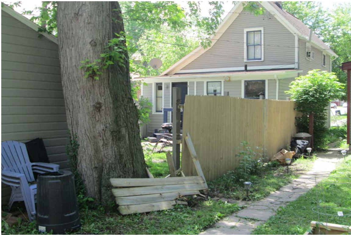
Facing southwest to damaged fence along north property line.
