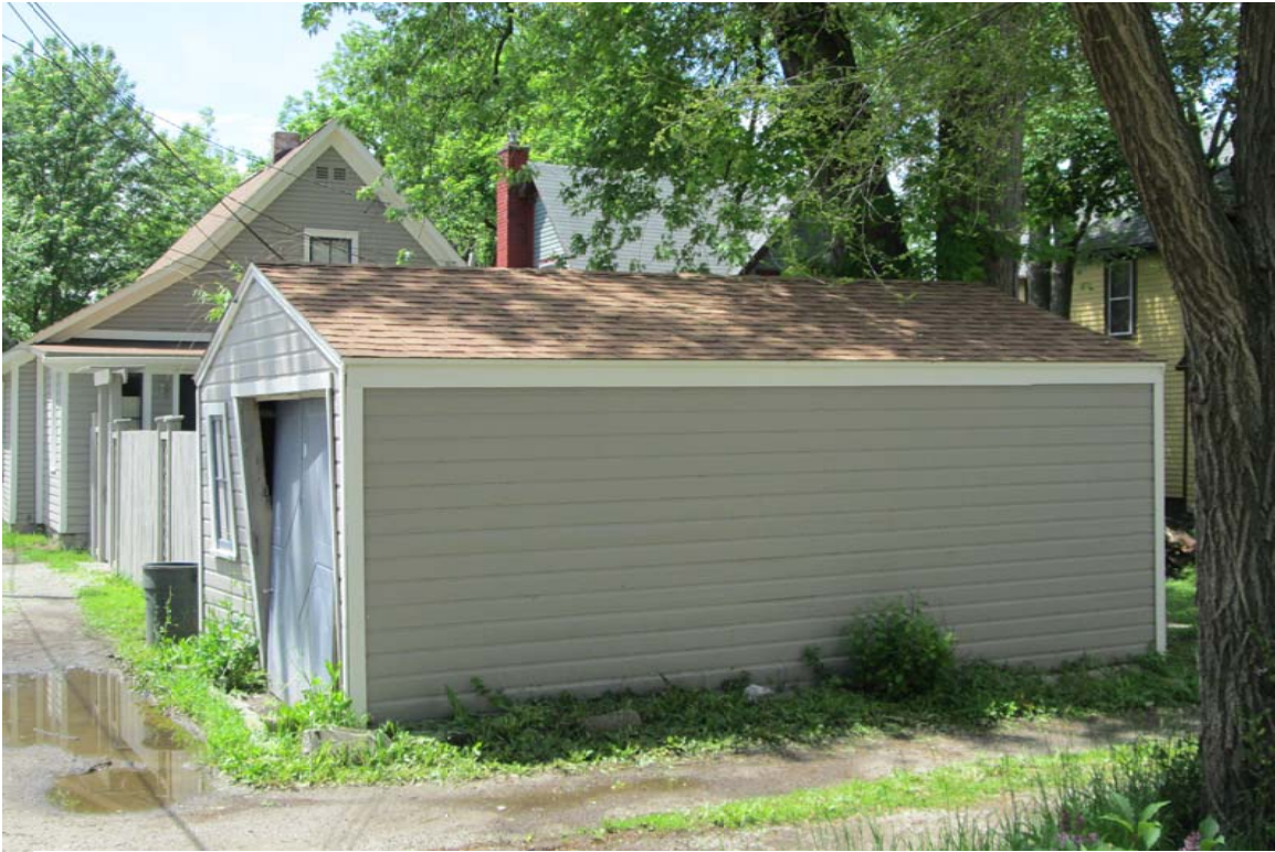
Facing west-northwest to east and south elevations of garage.
