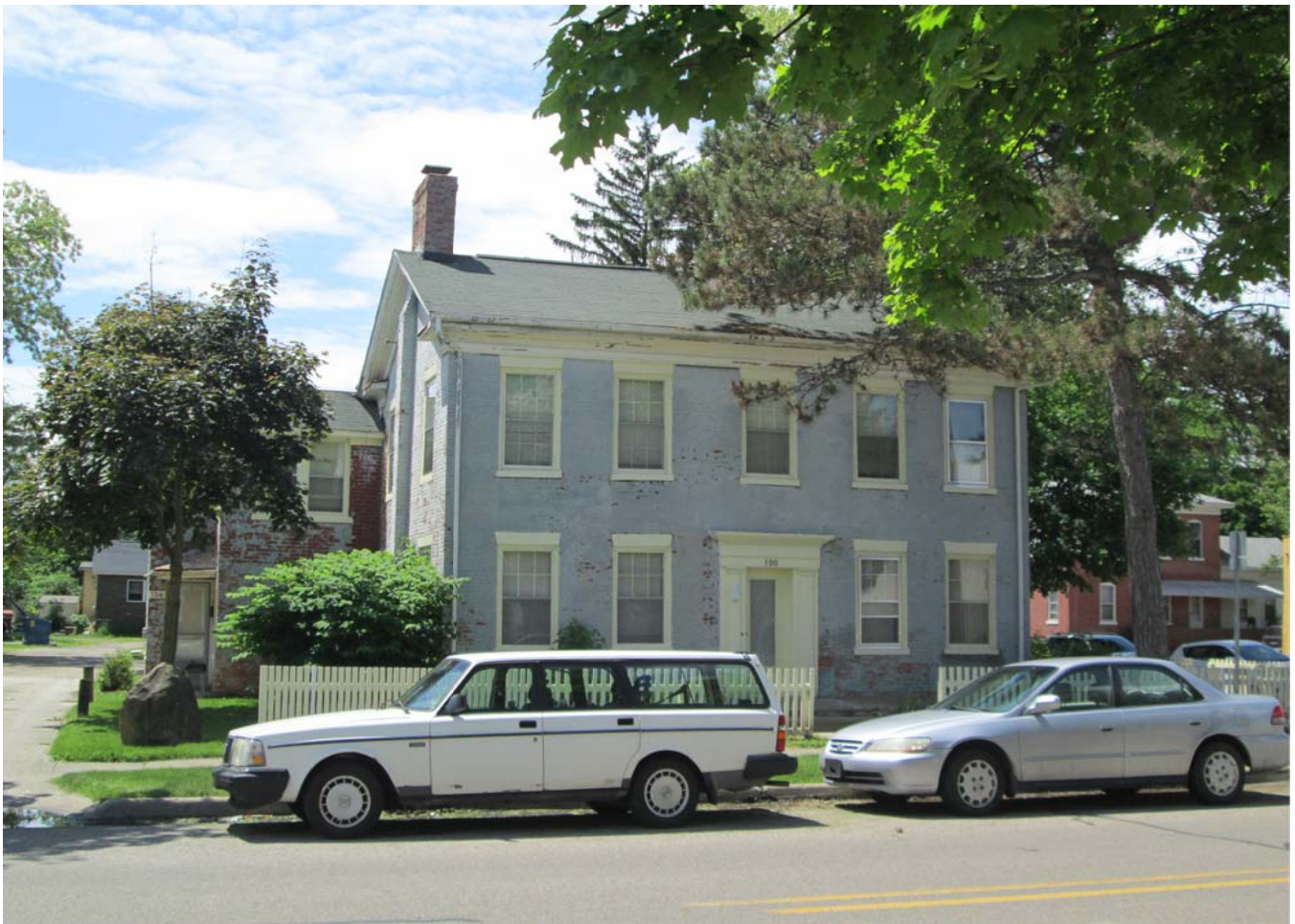
Facing west-northwest to facade and south elevation.
