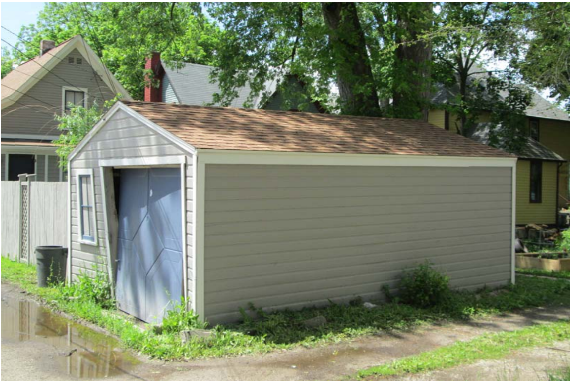
Facing northwest to south and east elevations of garage.
