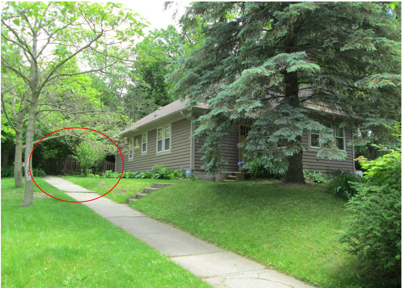
Facing southeast to house and current fence.
