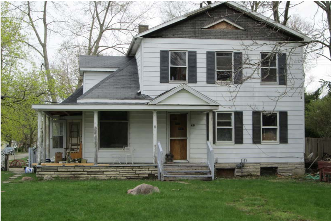
Facing north to facade.
