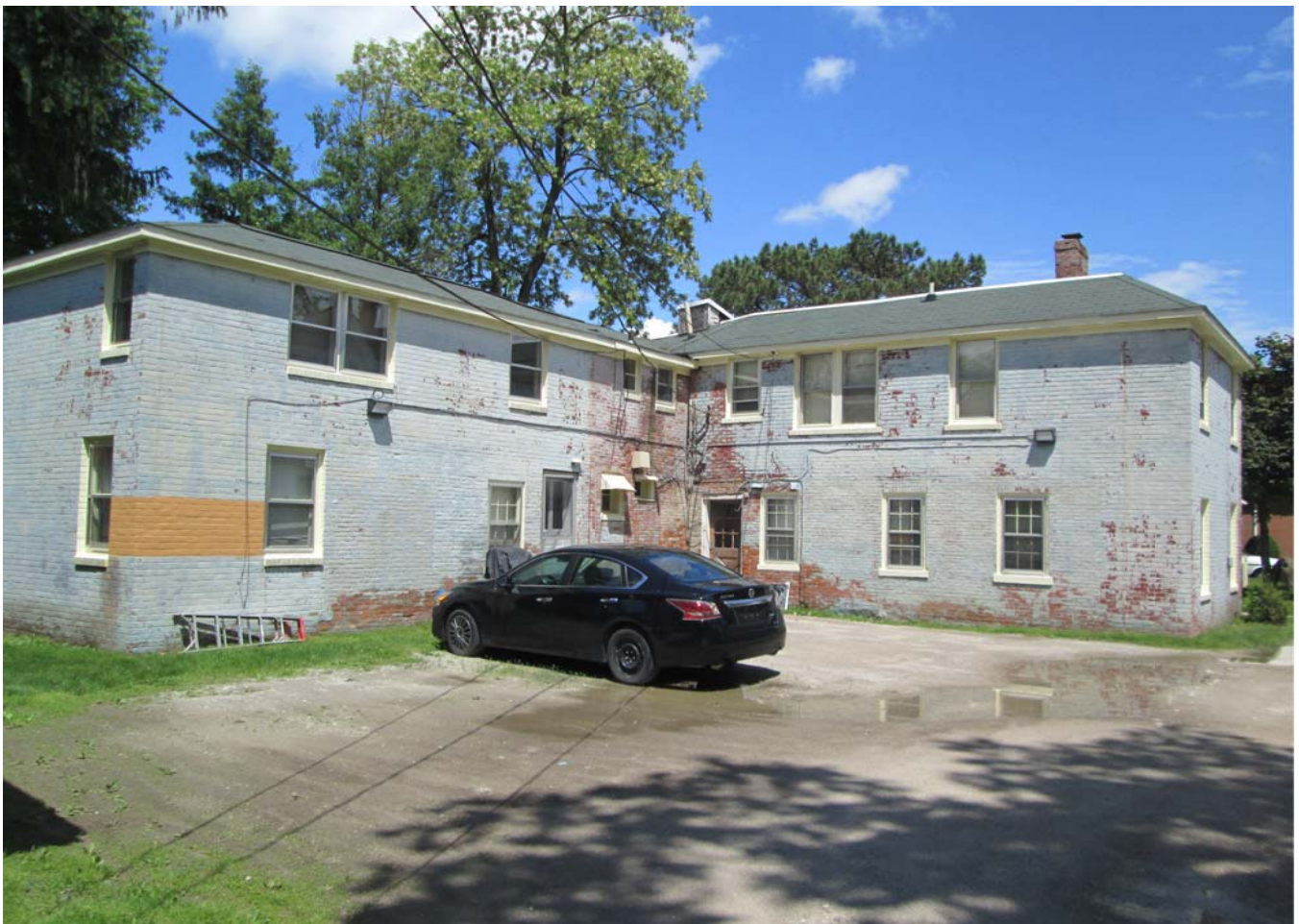
Facing northeast to west and south elevations.
