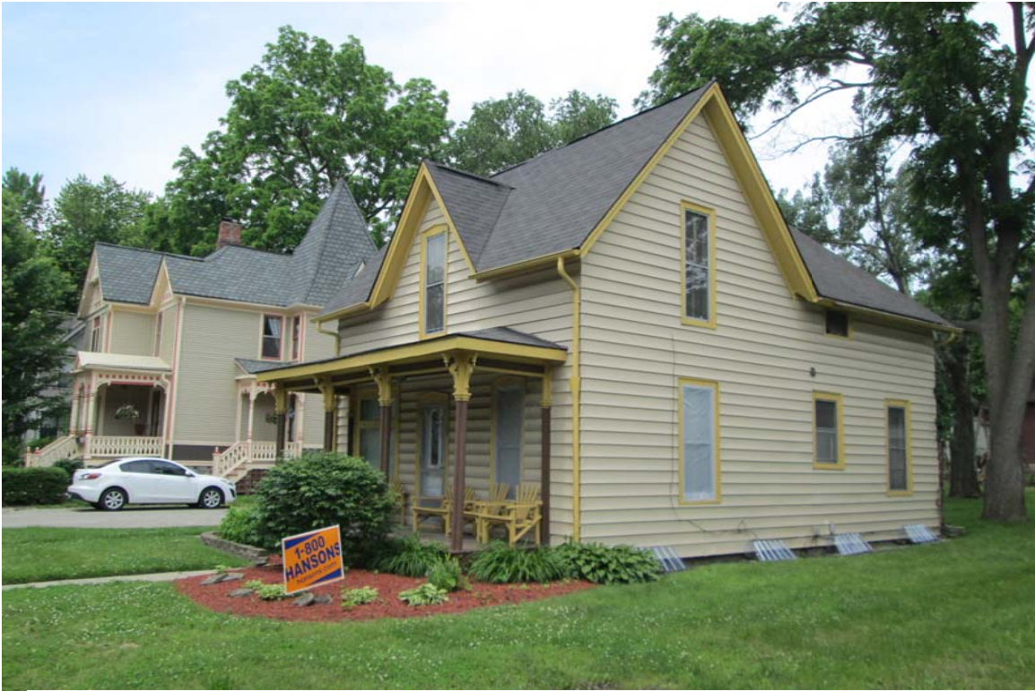
Facing northwest to facade and east elevation.
