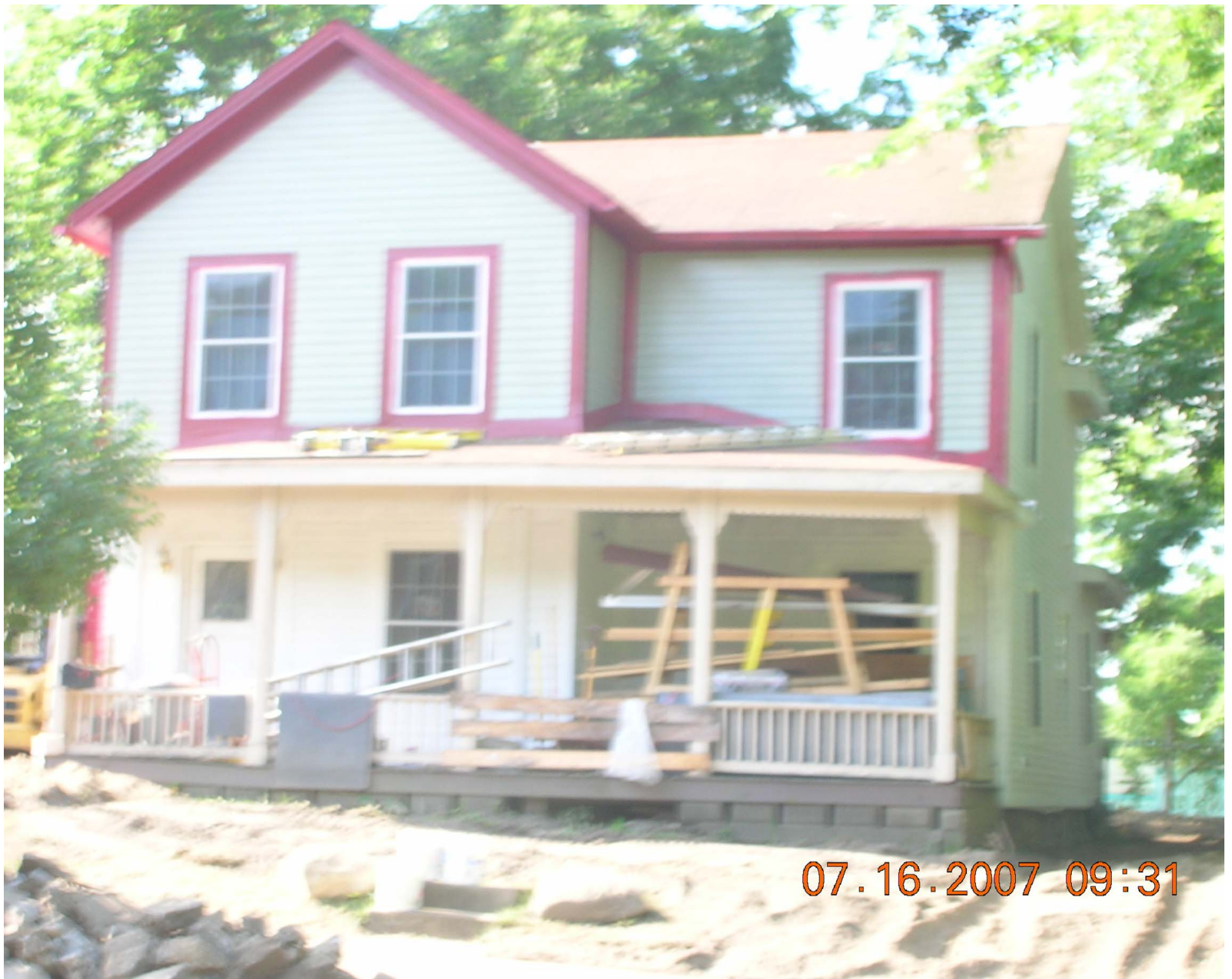
Photo showing siding on west elevation when first installed.
