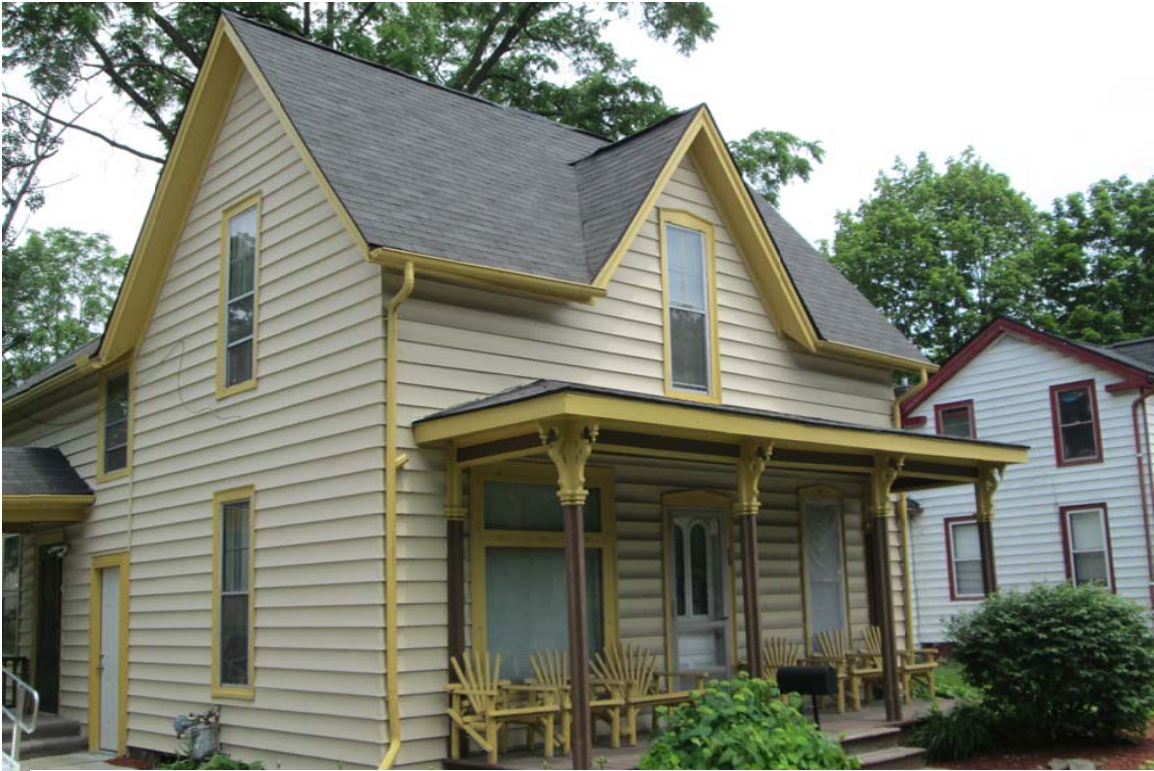
Facing northeast to facade and west elevation.
