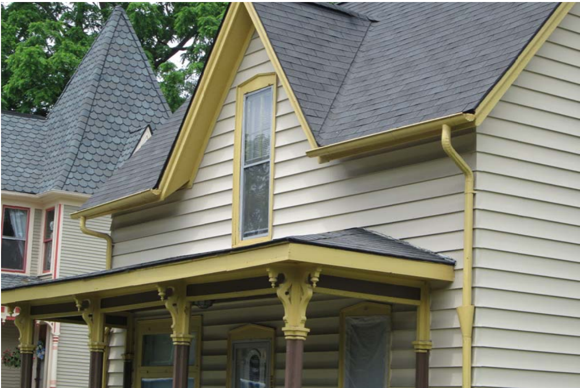
Facing northwest showing details of facade gutters.
