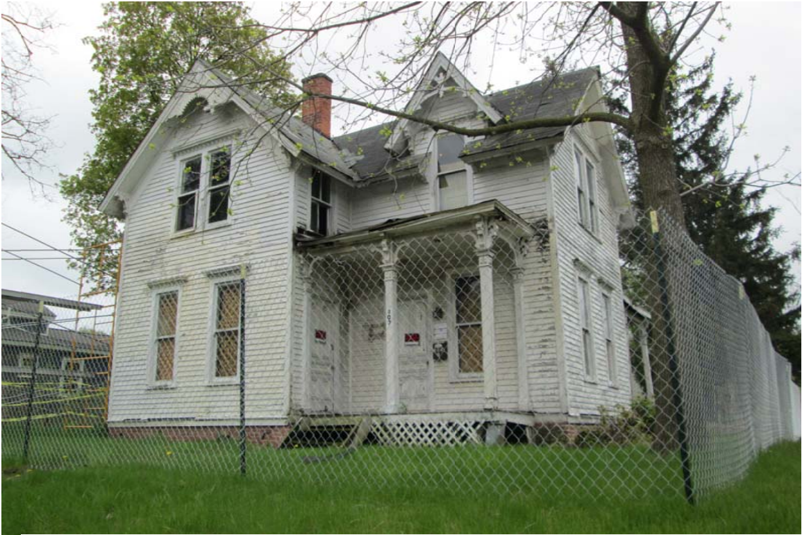
Facing southeast to facade and west elevation
