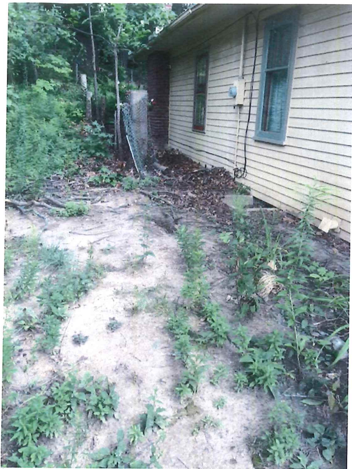
Area between 2 nd and 3 rd window on north side
