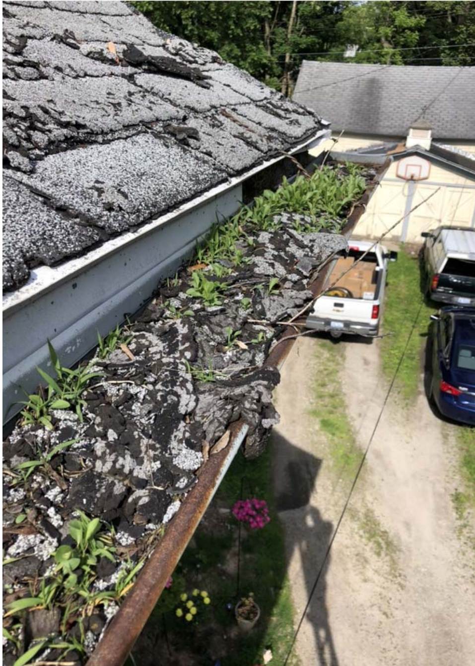
Applicant photos: 306 N Grove
