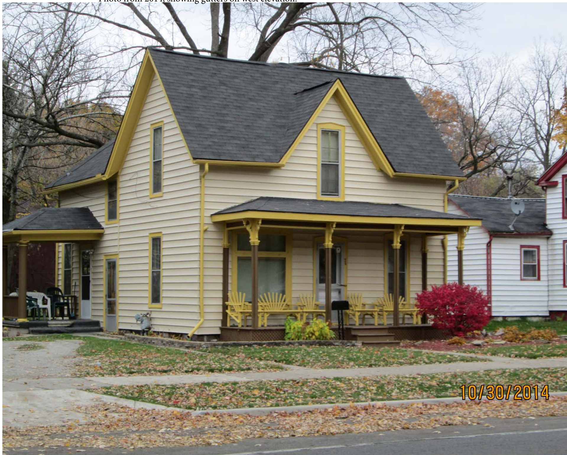
Photo from 2014, showing gutters on west elevation.
