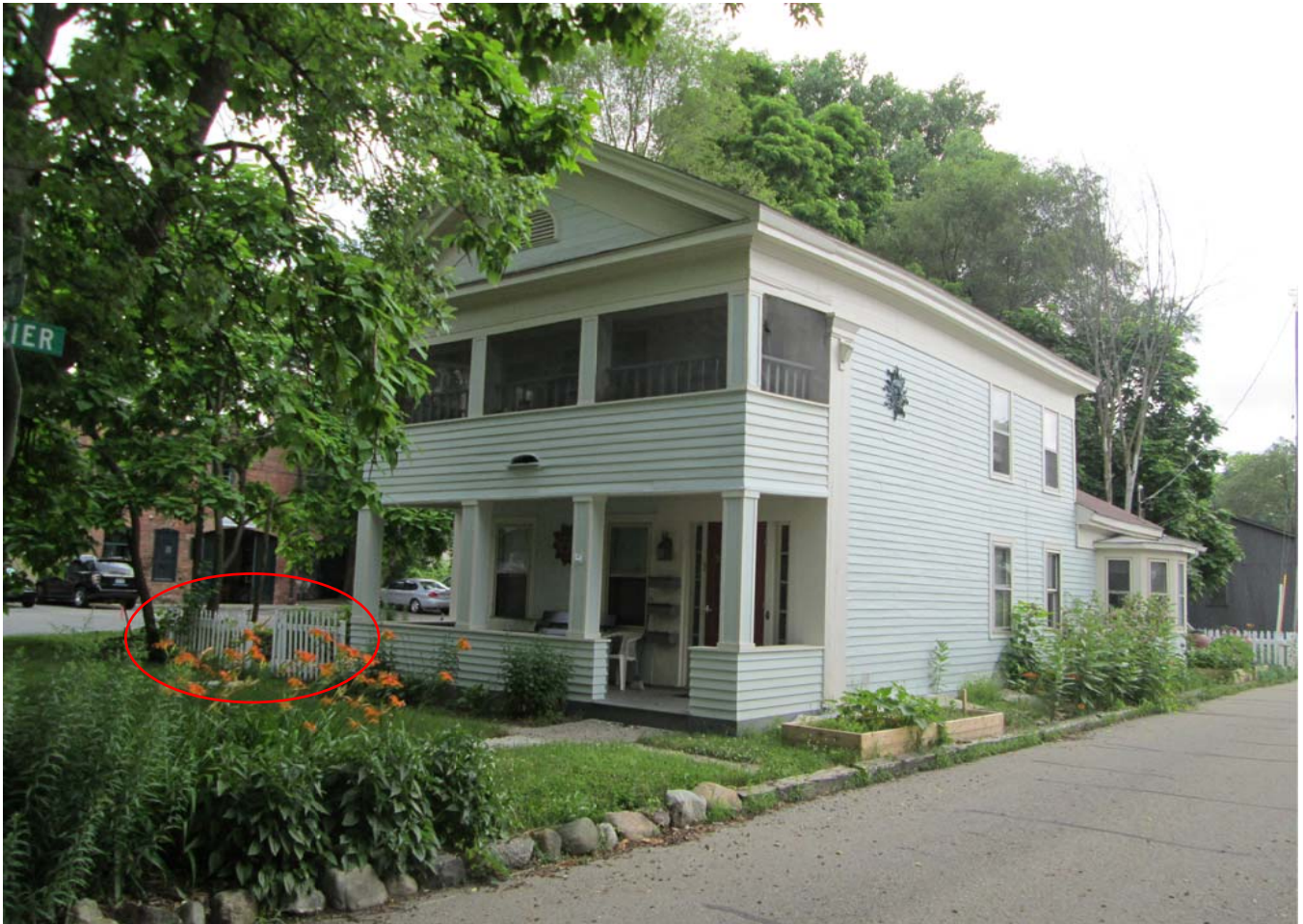
Facing northeast to facade and south elevation. Picket fence to receive gate at left of photo.
