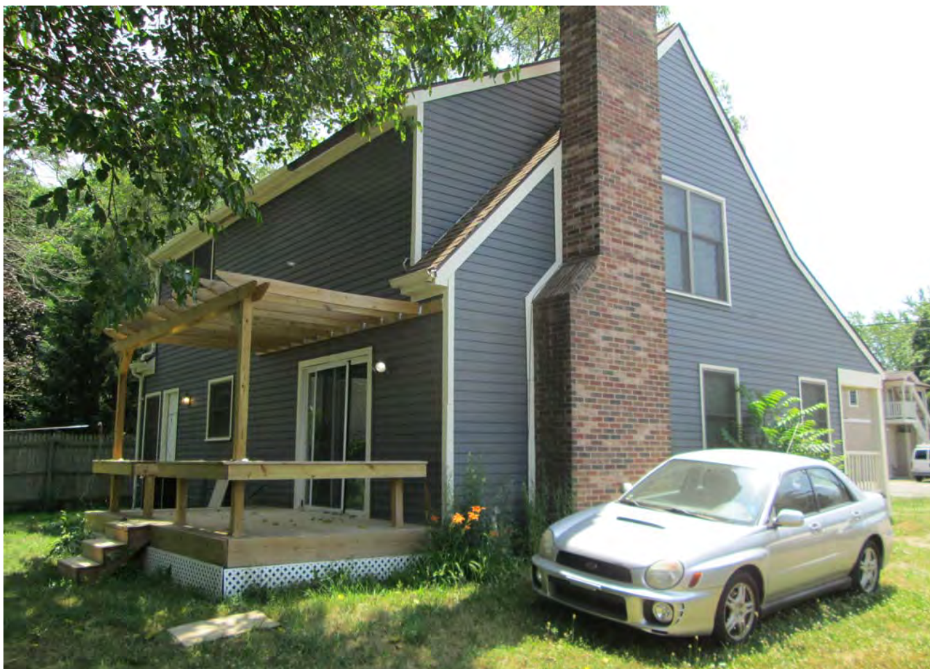
Facing southeast to deck/pergola showing the north and west elevations.
