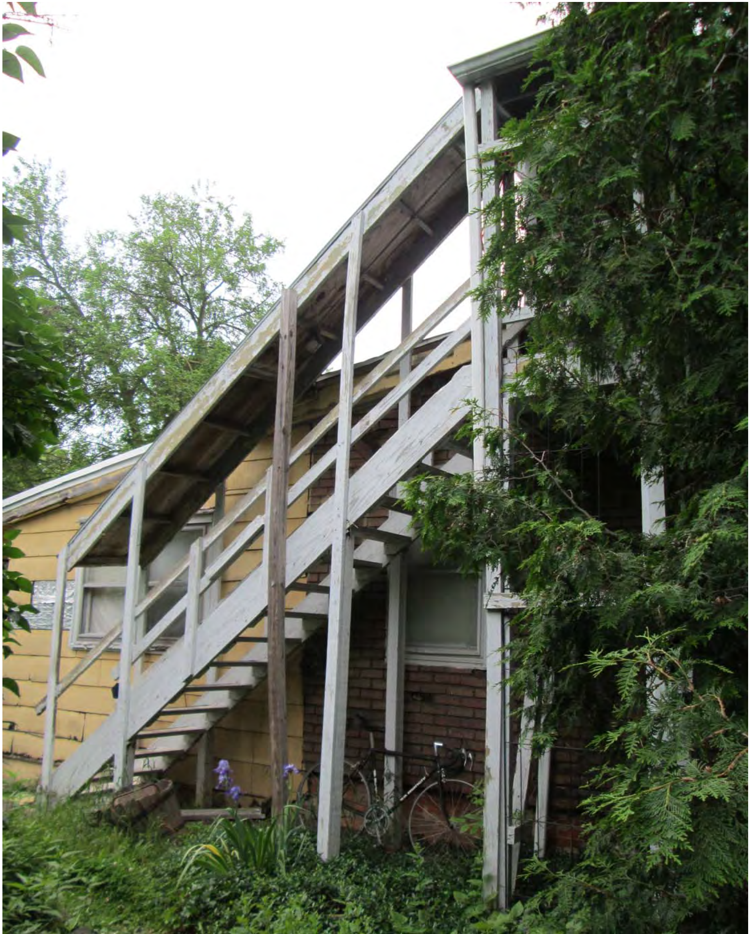
Facing northwest to staircase on south elevation. Staircase is entirely obscured from the right-of-way by large evergreen trees.
