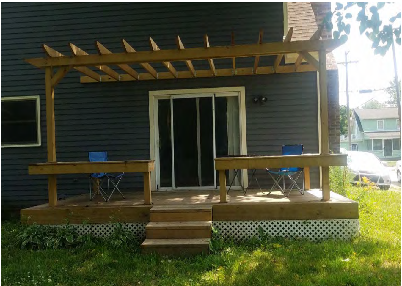
Facing south to newly constructed deck- to be stained and added framing on deck skirting.
