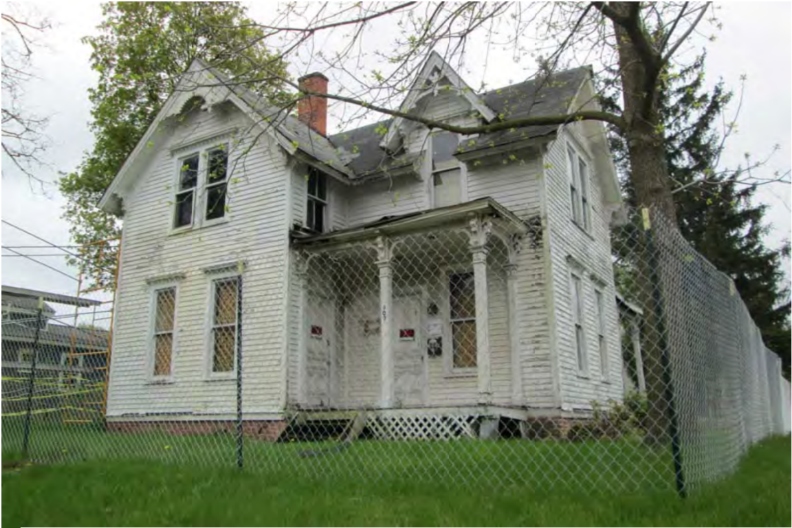
Facing southeast to facade and west elevation
