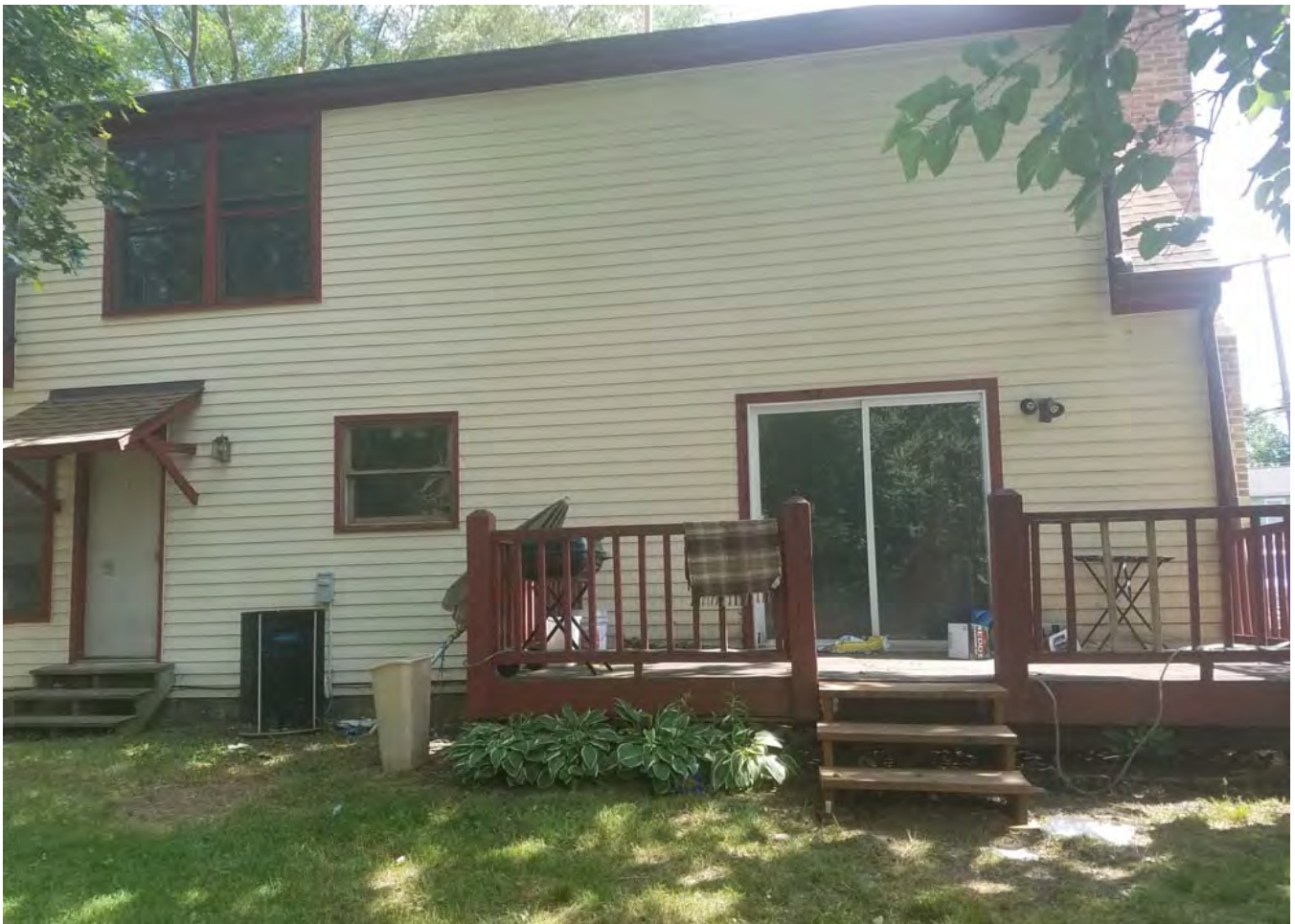
Facing south to deck prior to reconstruction.
