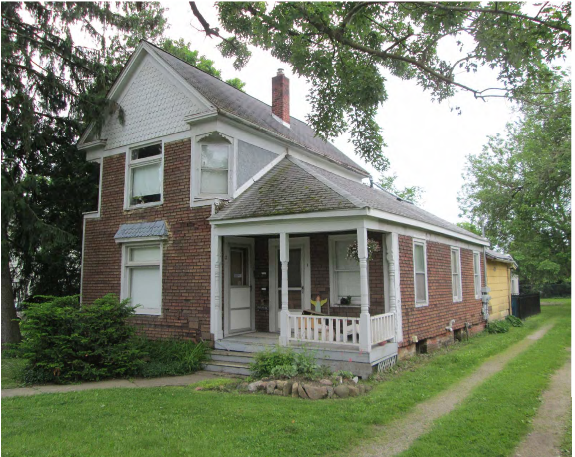
509 N River, Facing Southwest to Facade and North Elevation (for reference).
