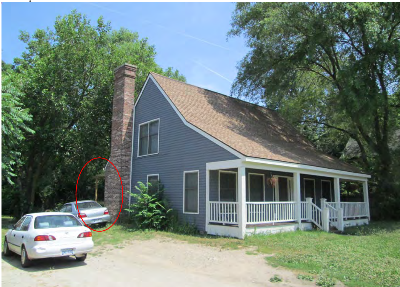
Facing northeast to the facade and west elevation. Showing the deck/pergola view from the right-of-way.
