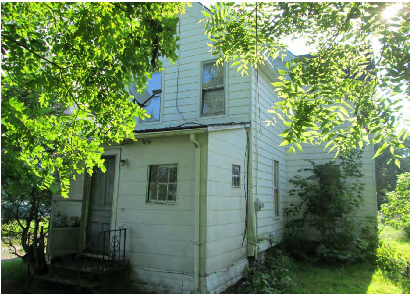
Facing northeast to west and south elevations.
