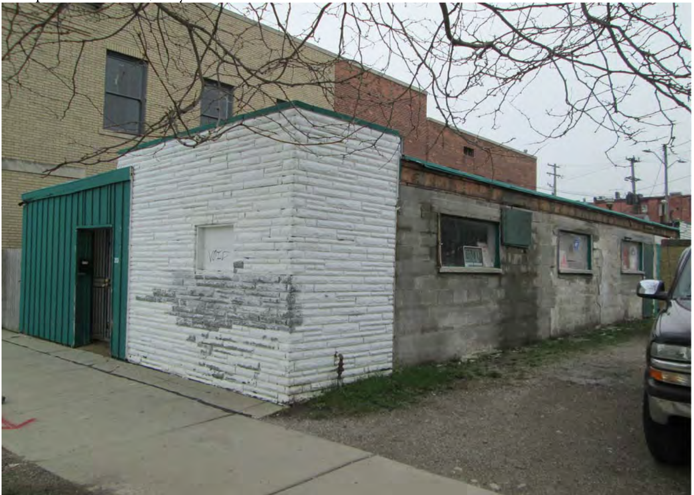
Facing southeast to facade and west elevation.
