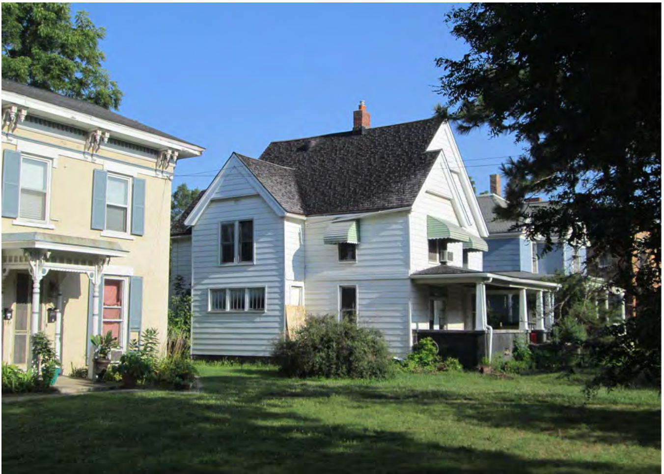
Facing northwest to facade and south elevation.
