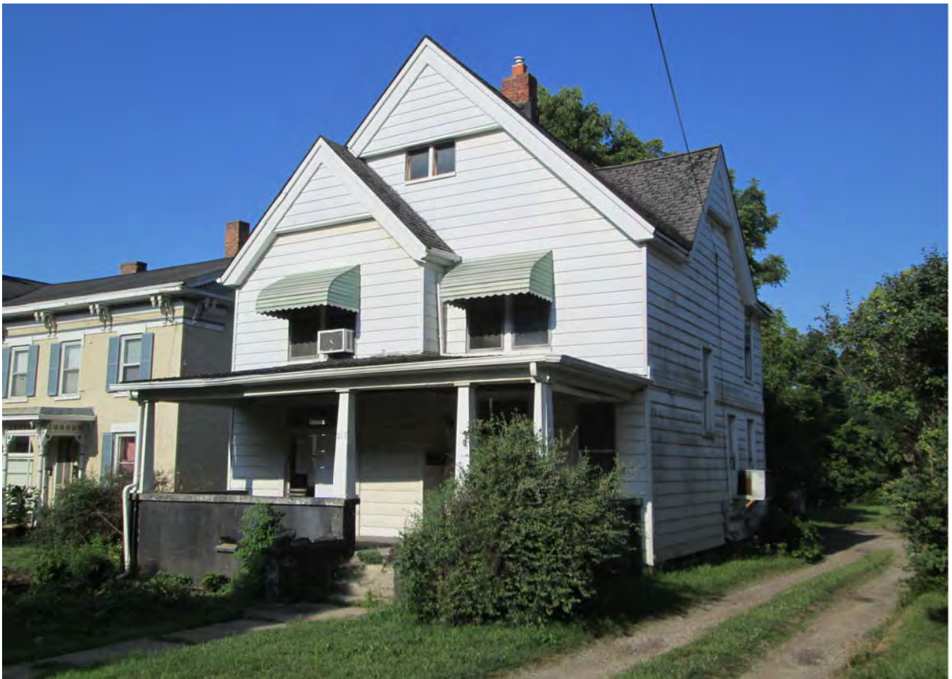
Facing southwest to facade and north elevation.
