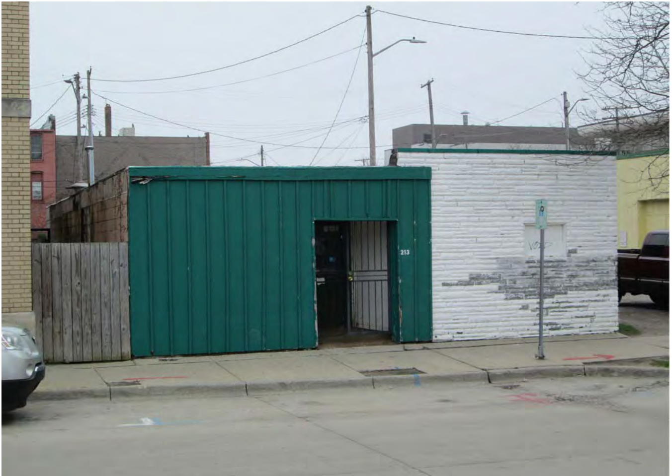
Facing southwest to facade and east elevation.
