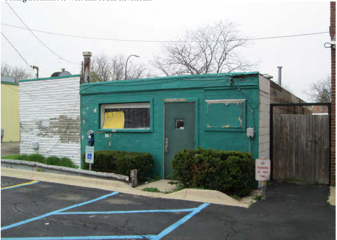
Facing northwest to south and east elevations.
