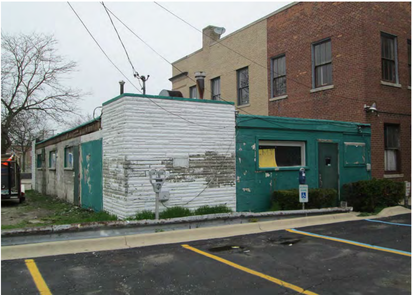
Facing northeast to west and south elevations.
