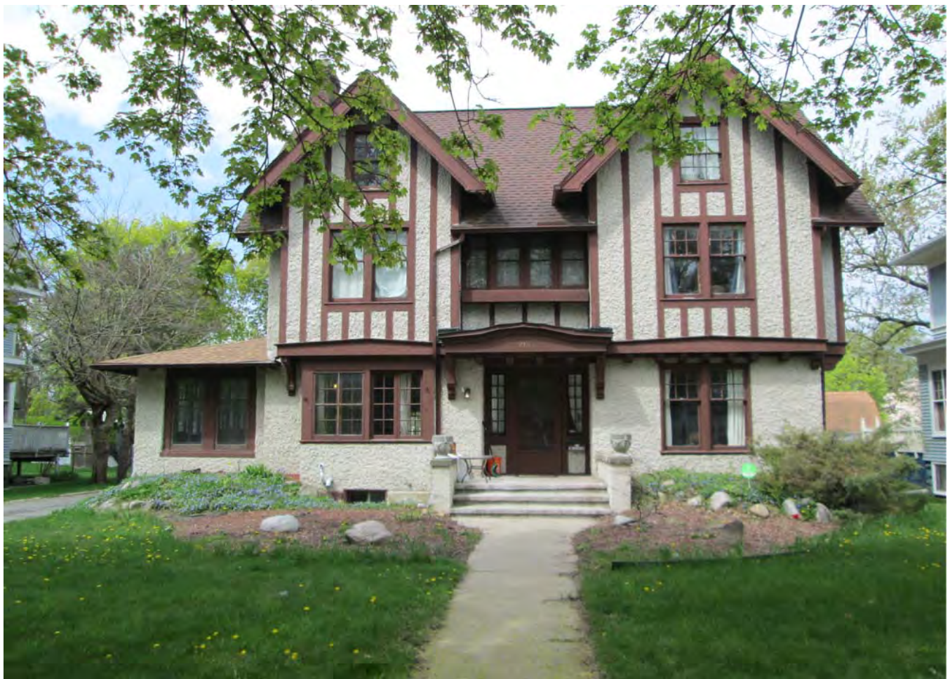
Facing west to facade.
