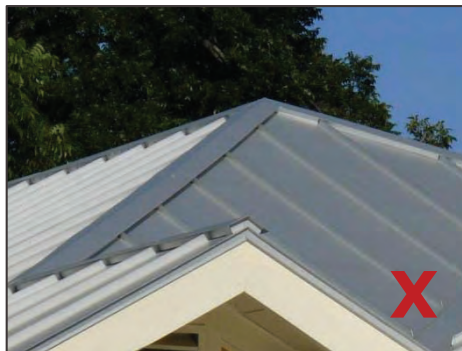
Do not use ridge caps with ridge cap vent (left) or end caps (right).
