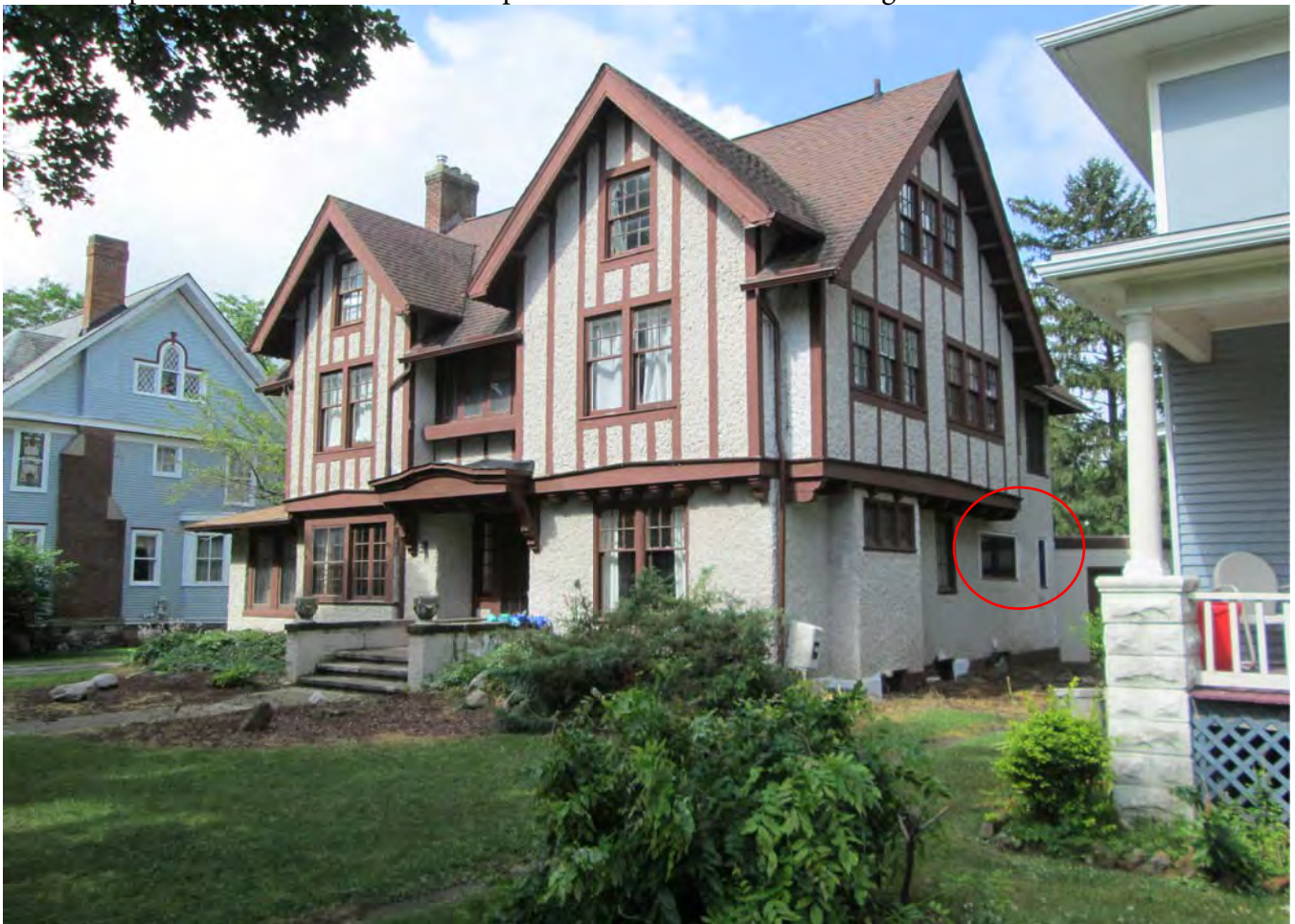
Staff photos 7/18/2019- windows replaced to-date at 216 S Washington
