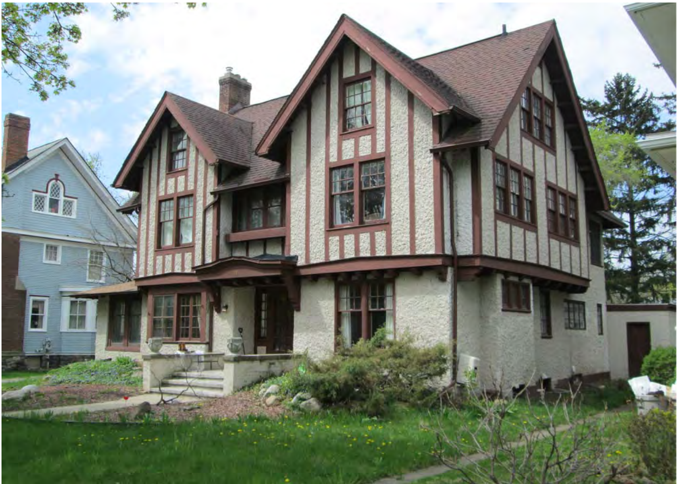
Facing southwest to facade and north elevation.
