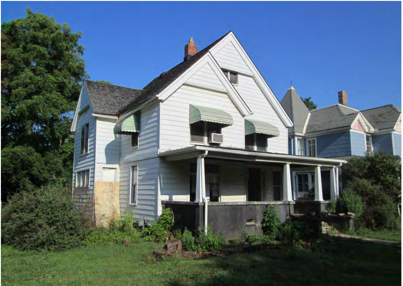
Facing northwest to facade and south elevation.
