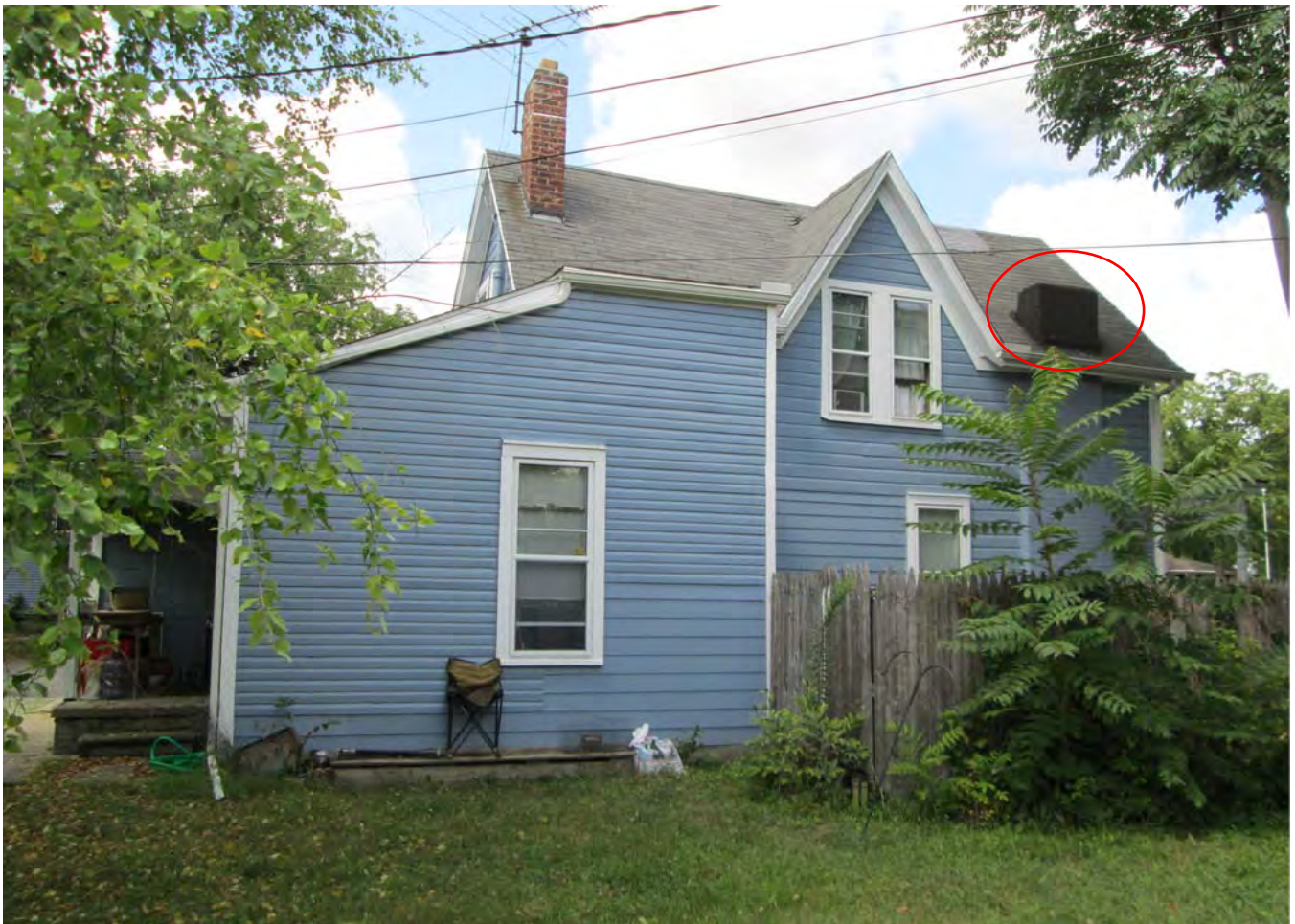
Facing west to east elevation. Chimney to be removed at right.
