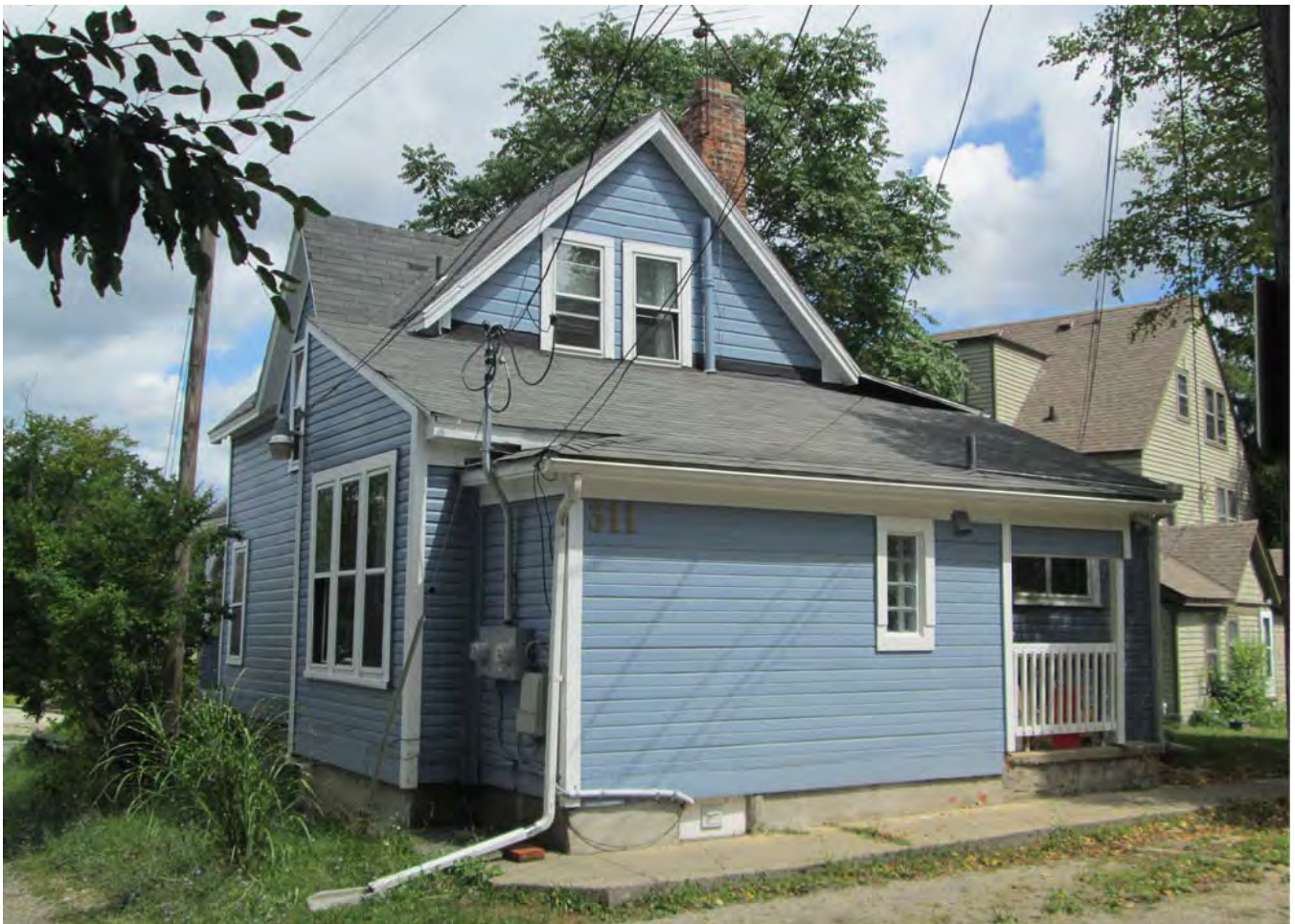
Facing northeast to west and south elevations.
