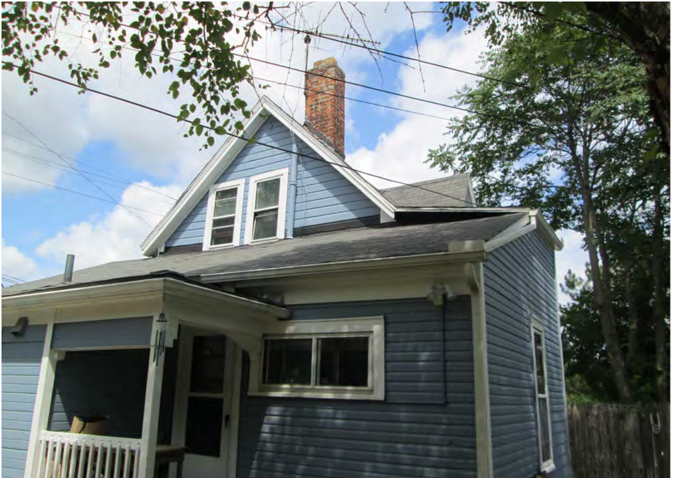
Facing northwest to south elevation.
