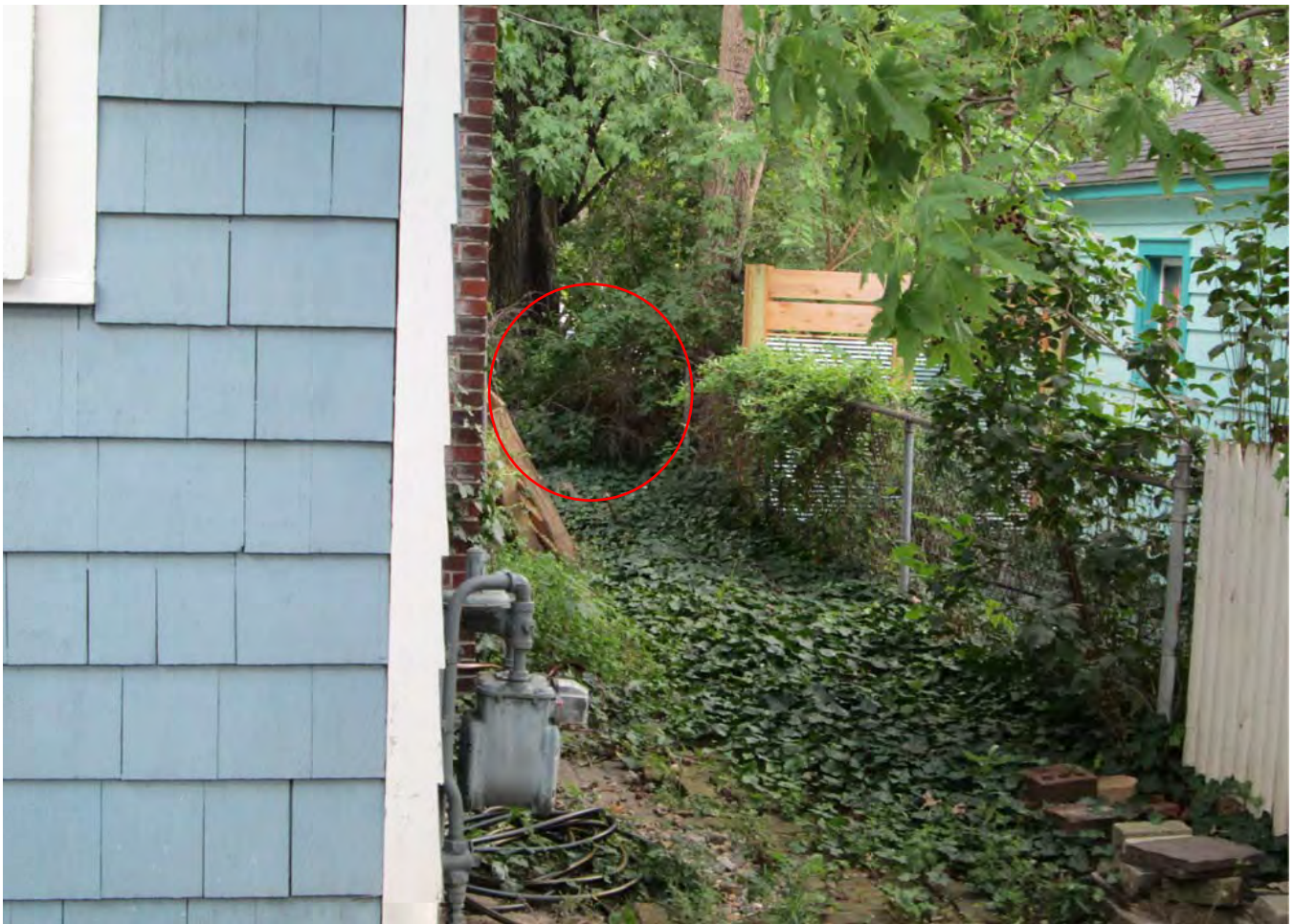
Facing east along south property line. Fence to be replaced circled.
