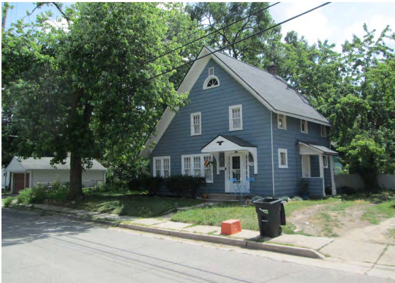
Facing southeast to facade and west elevation. Chain Linke Fence located along alley east of house.
