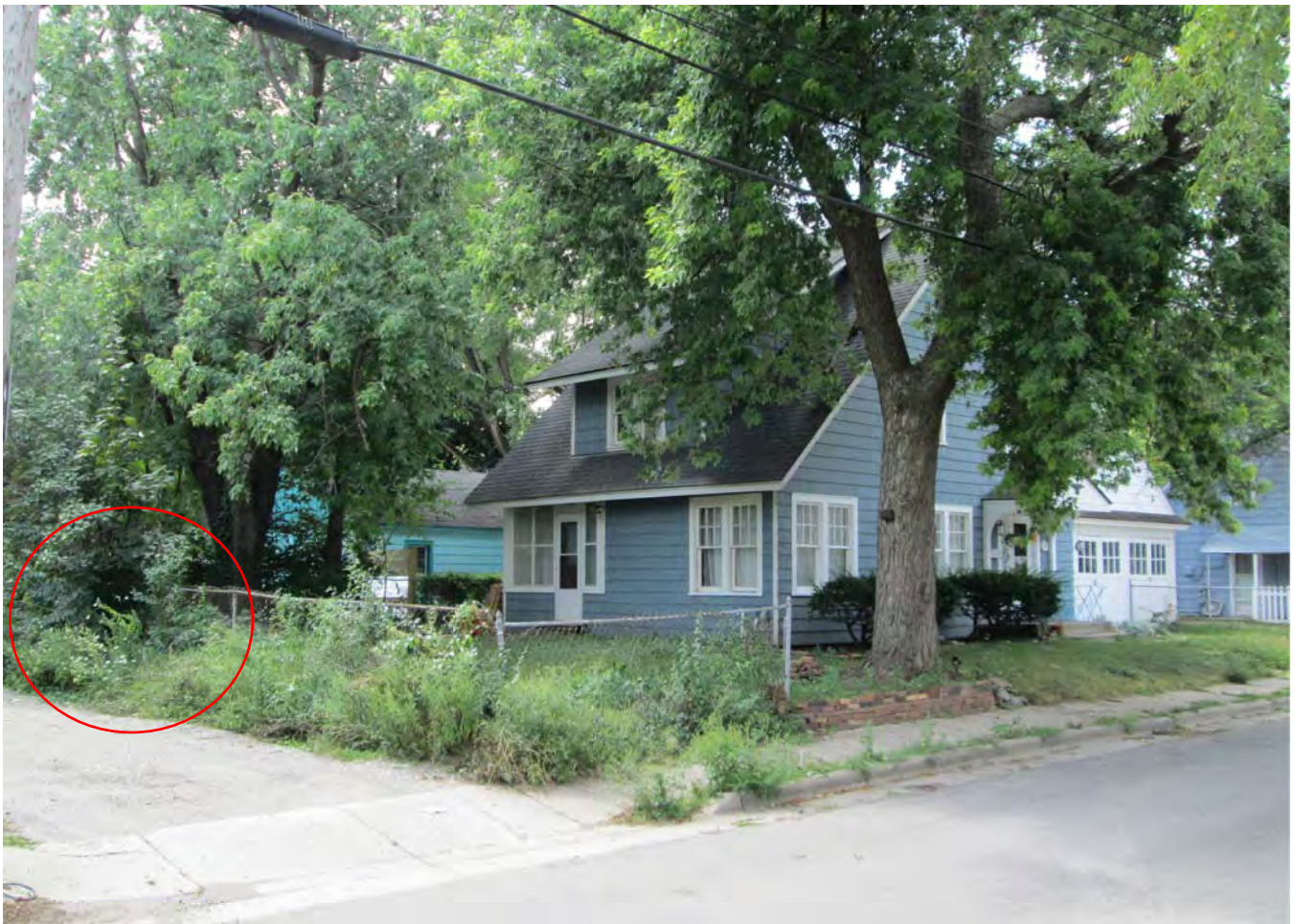
Facing southwest to facade and east elevation. Highlighted fence to be replaced.
