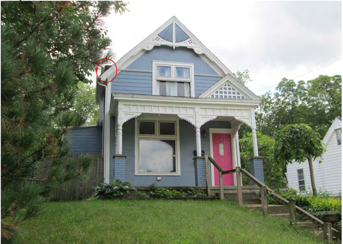
Facing south to facade. Chimny to be removed at left.
