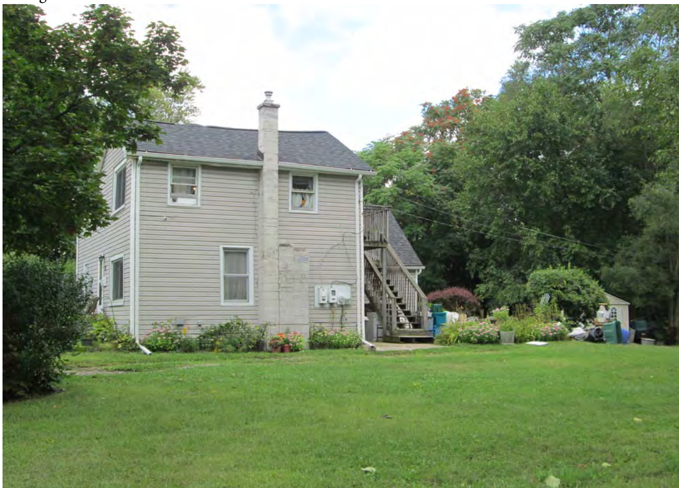
Facing northeast to facade and south elevation from right-of-way, staircase to be replaced at right.
