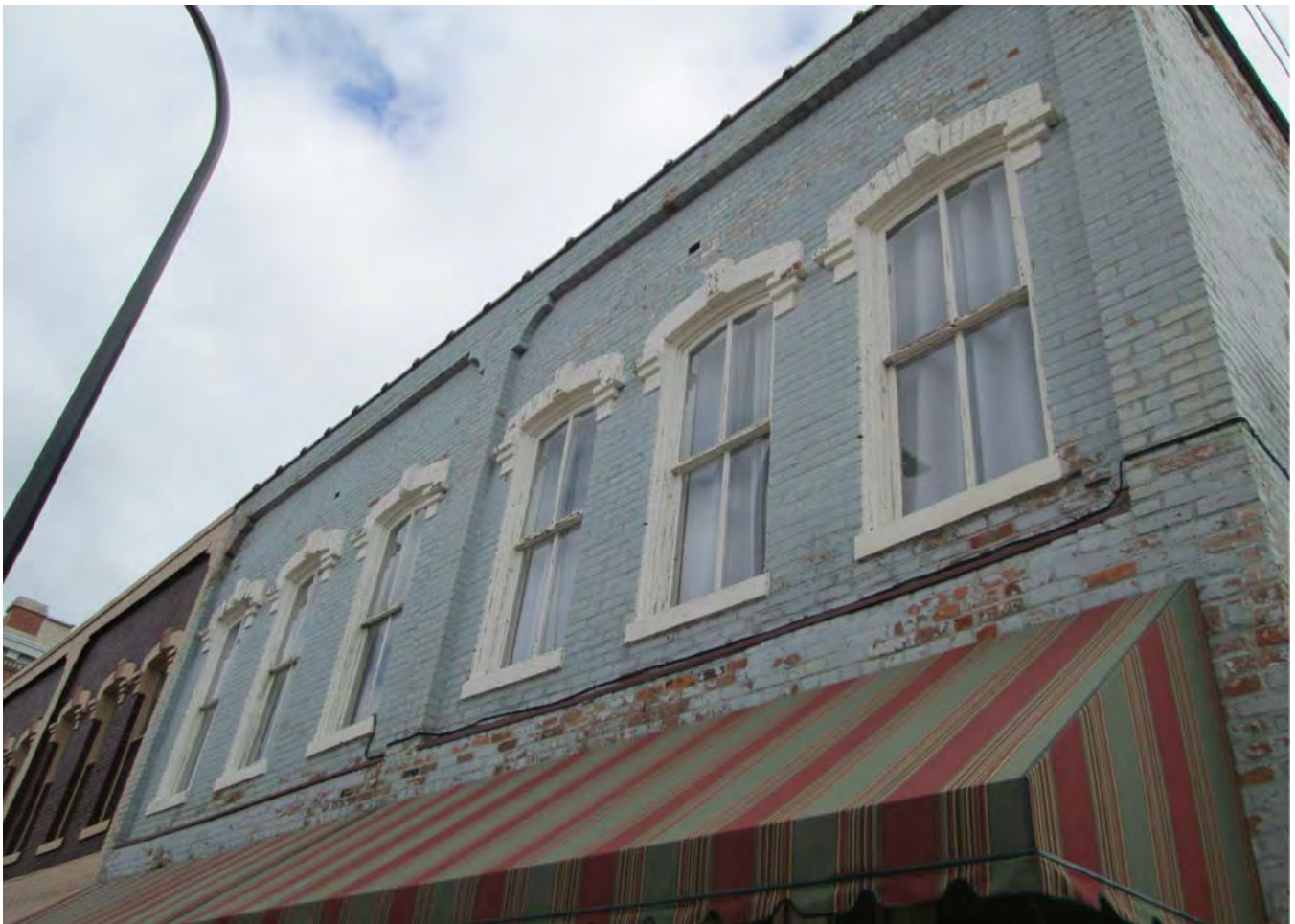
Facing northeast to facade second story windows.
