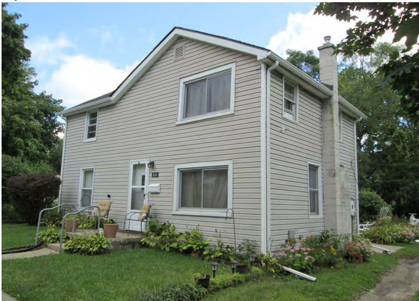
Facing northeast to facade and south elevation
