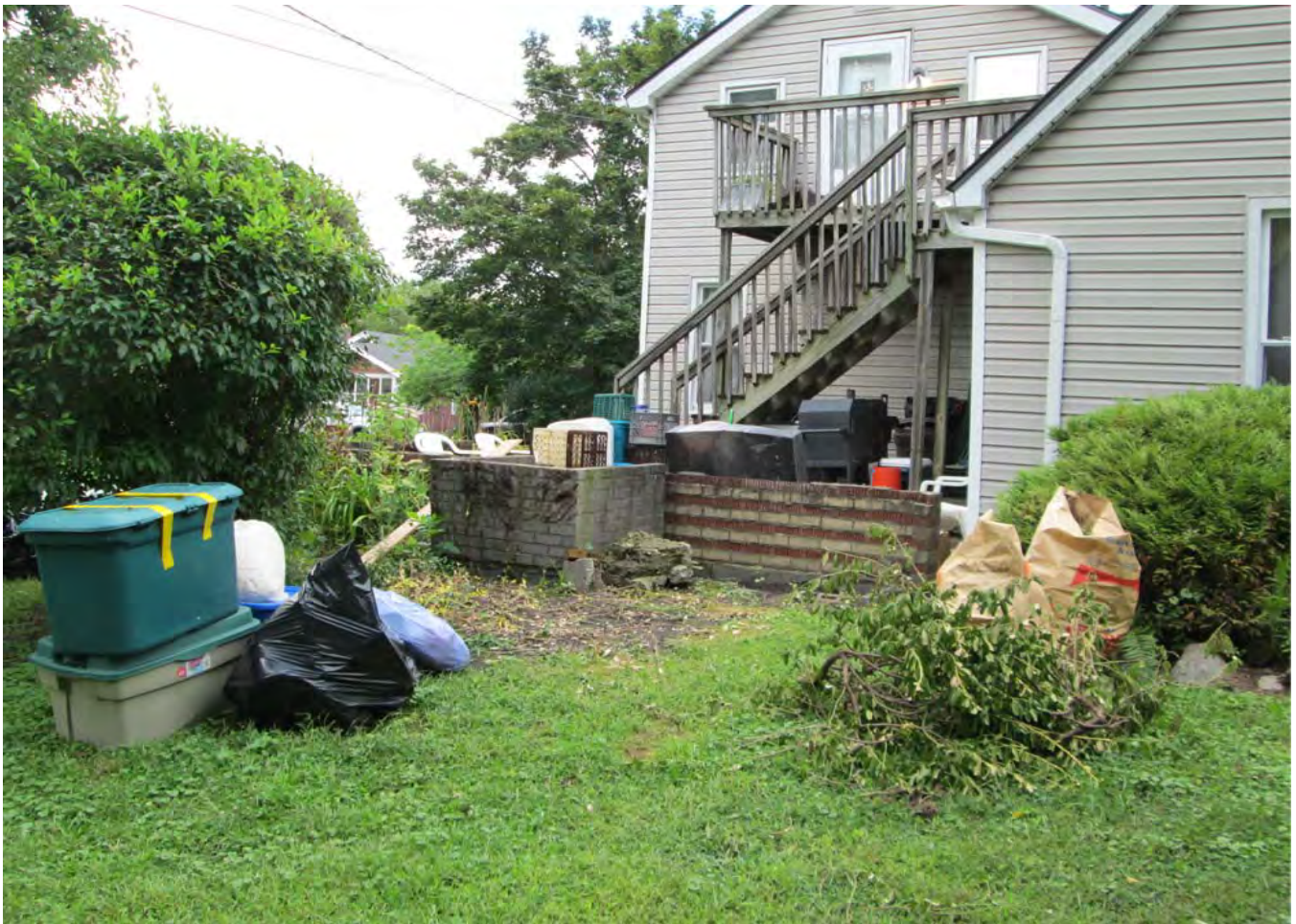
Facing west to rear east elevation and existing stair/balcony.
