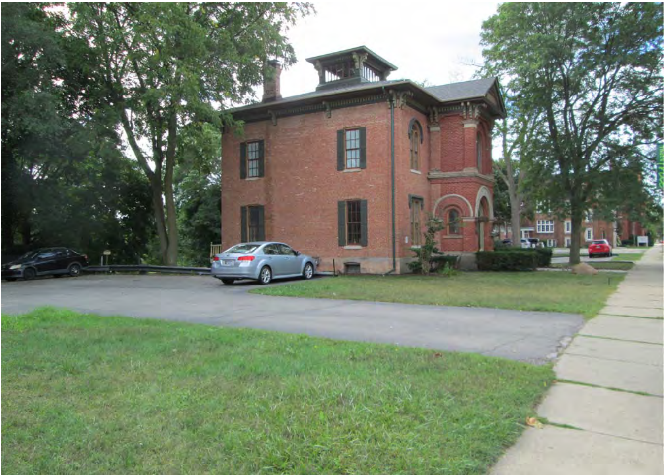
Facing south-southeast to south property boundary.
