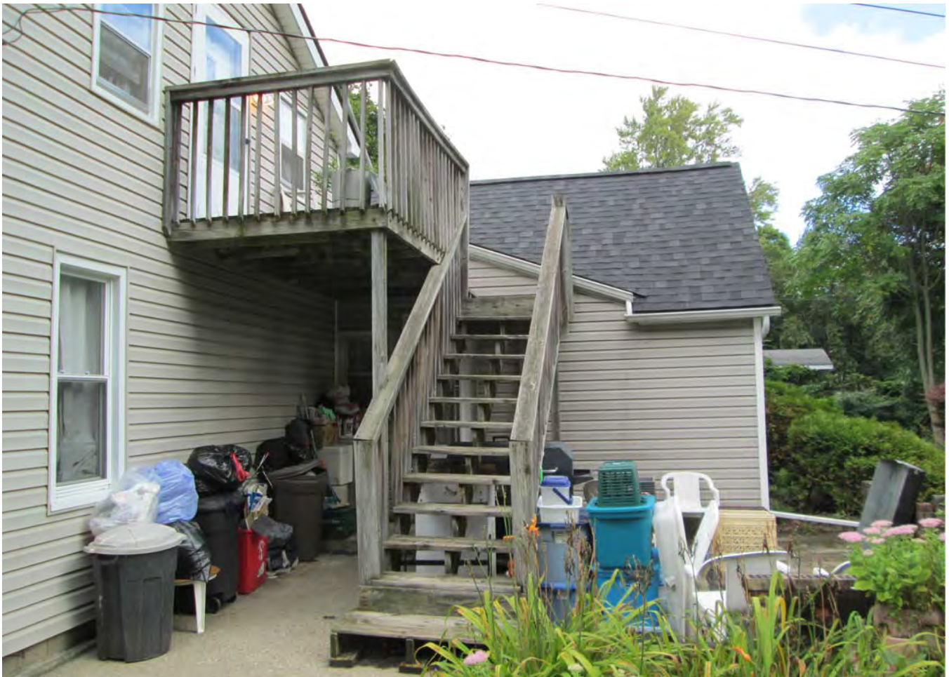
Facing north to stairs and balcony.
