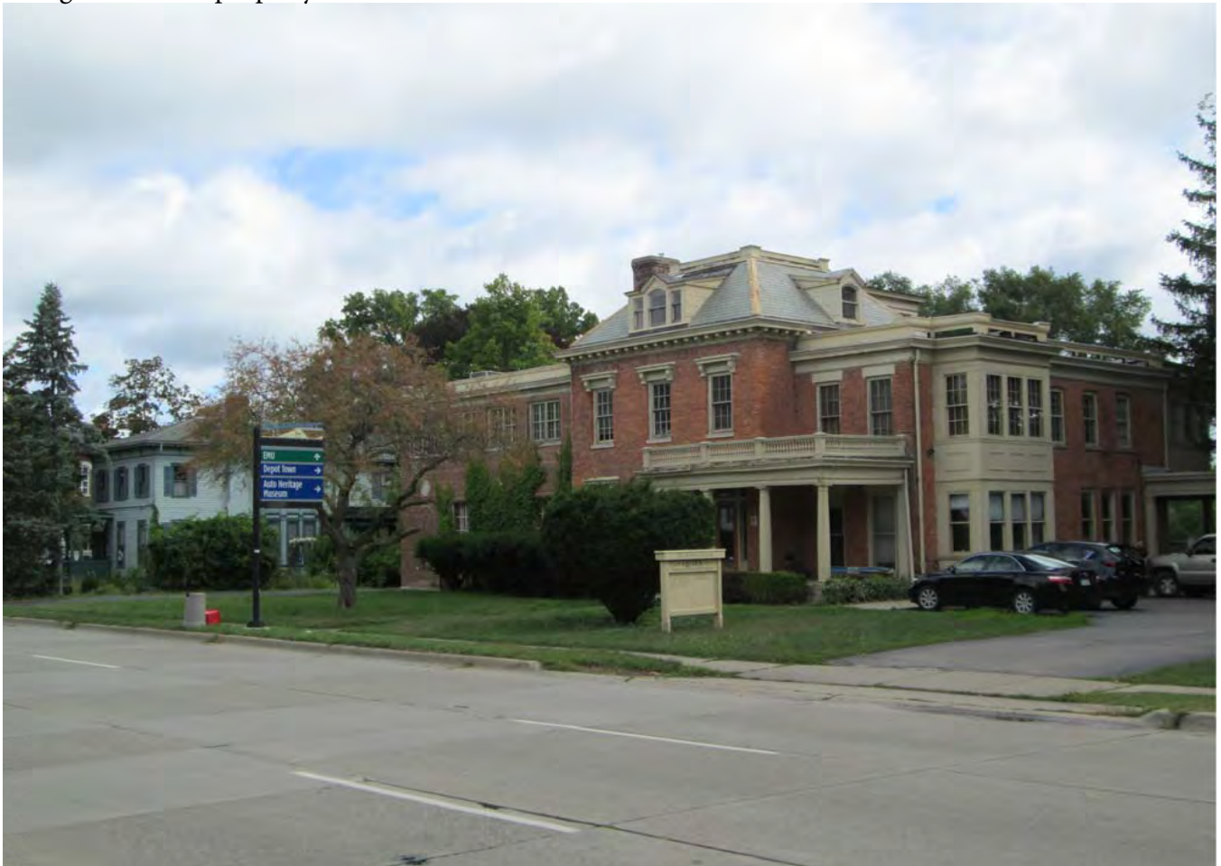
Facing northeast to house.
