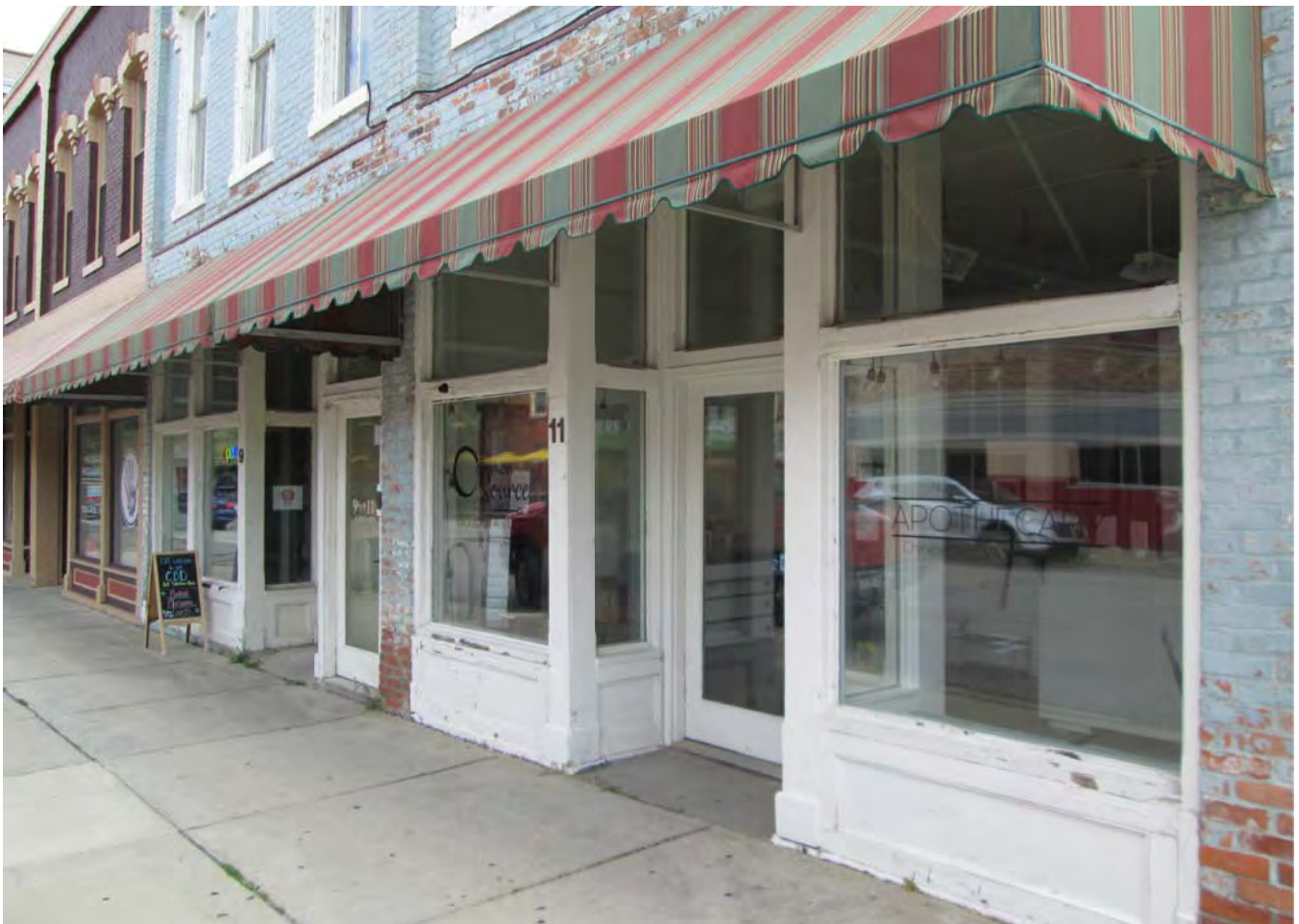
Facing northeast to storefront.
