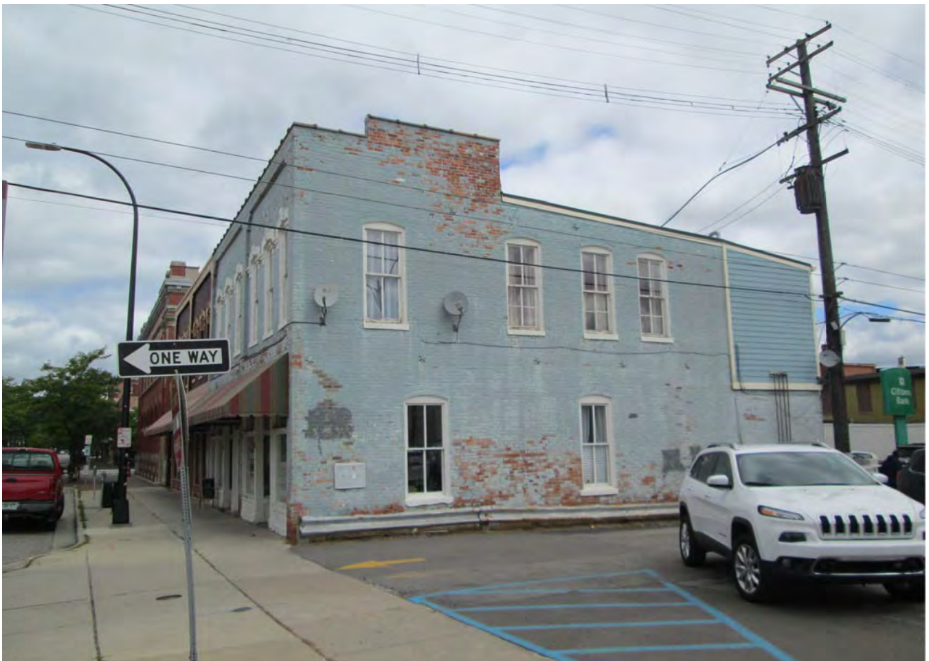
Facing northeast to facade and south elevation.
