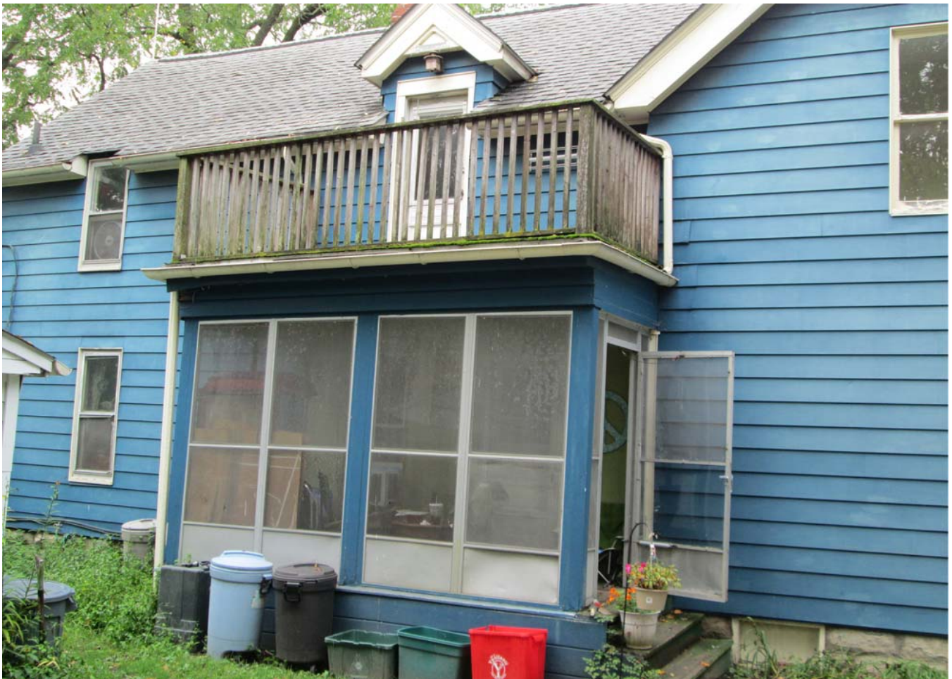
Facing southwest to east elevation porch
