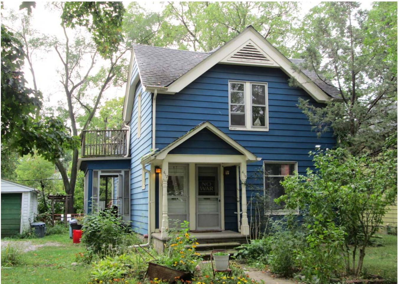
Facing southwest to facade and east elevation.
