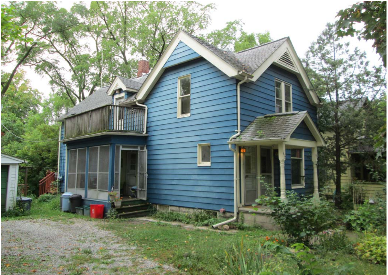
Facing southwest to facade and east elevation.
