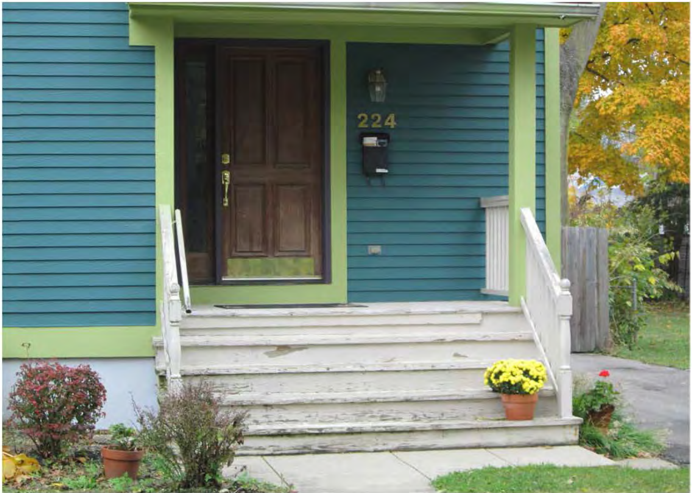
Staff photos of 224 N River, facing east-southeast to facade and facade porch.
