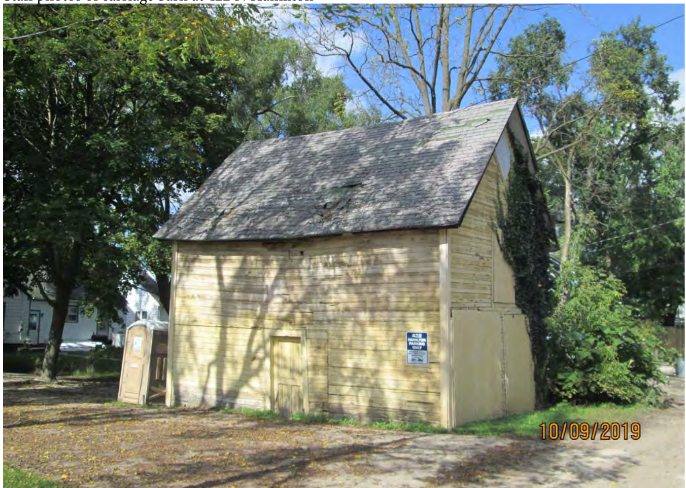
Facing northwest to south and east elevations.
