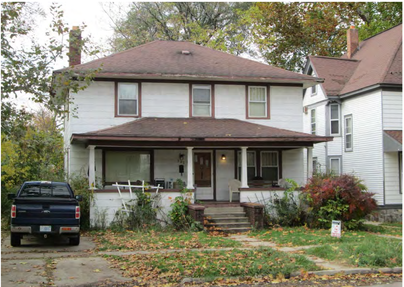
Facing west to facade.
