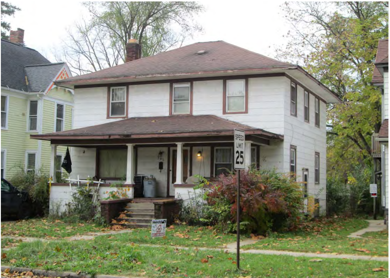
Facing southwest to facade and north elevation.
