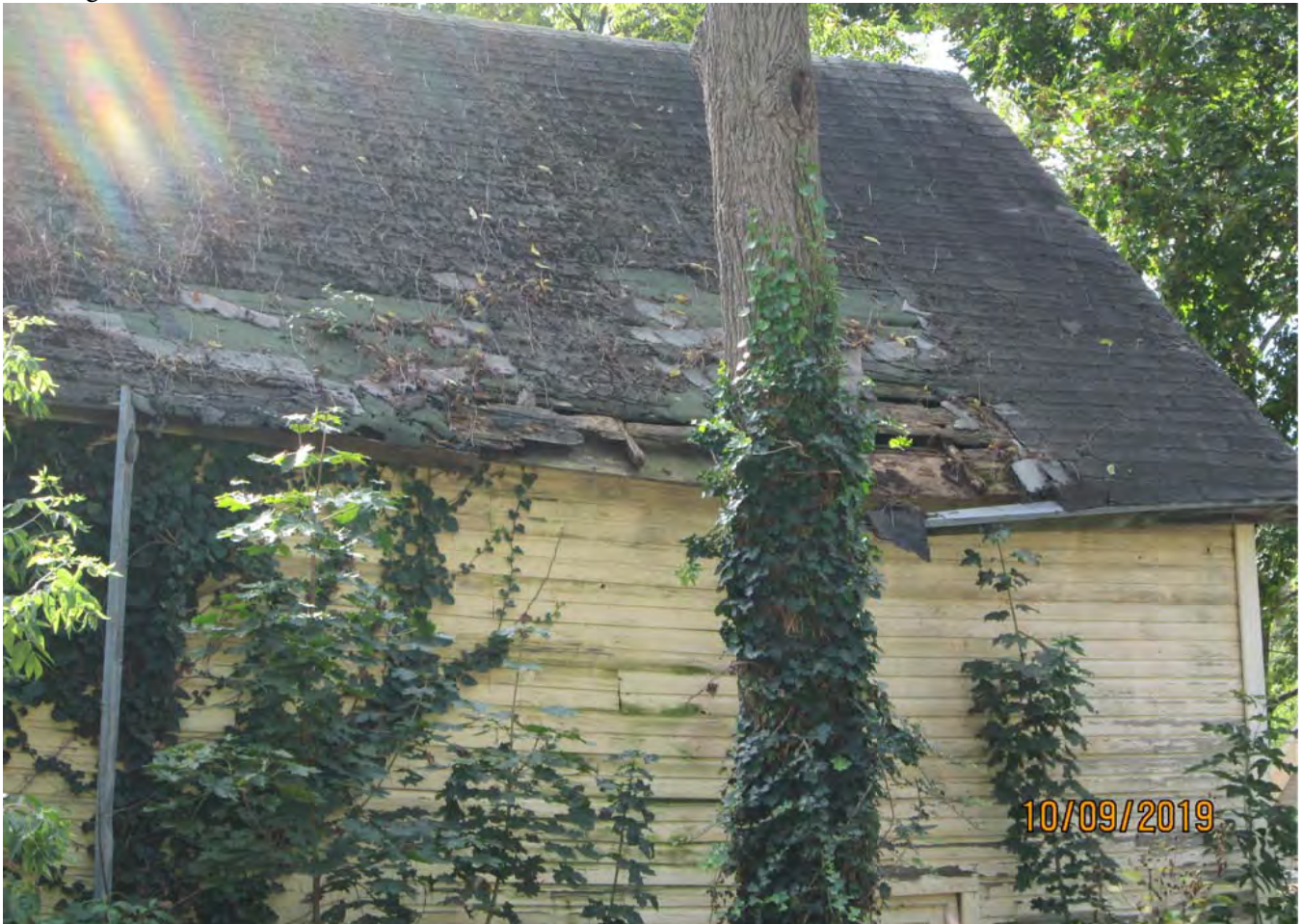
Roof detail- north slope.
