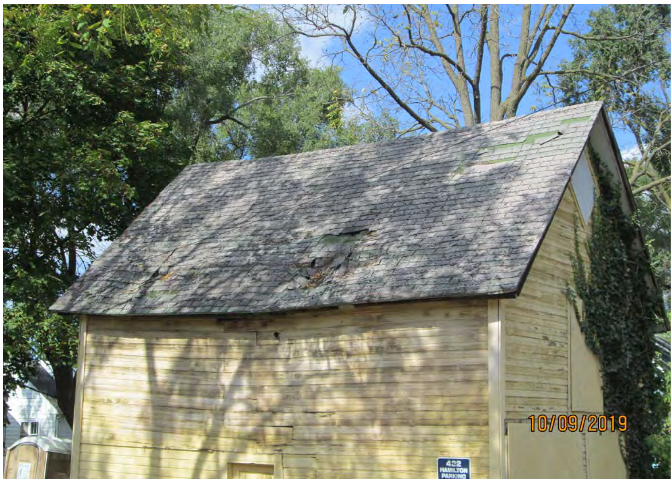
Roof detail- south slope.
