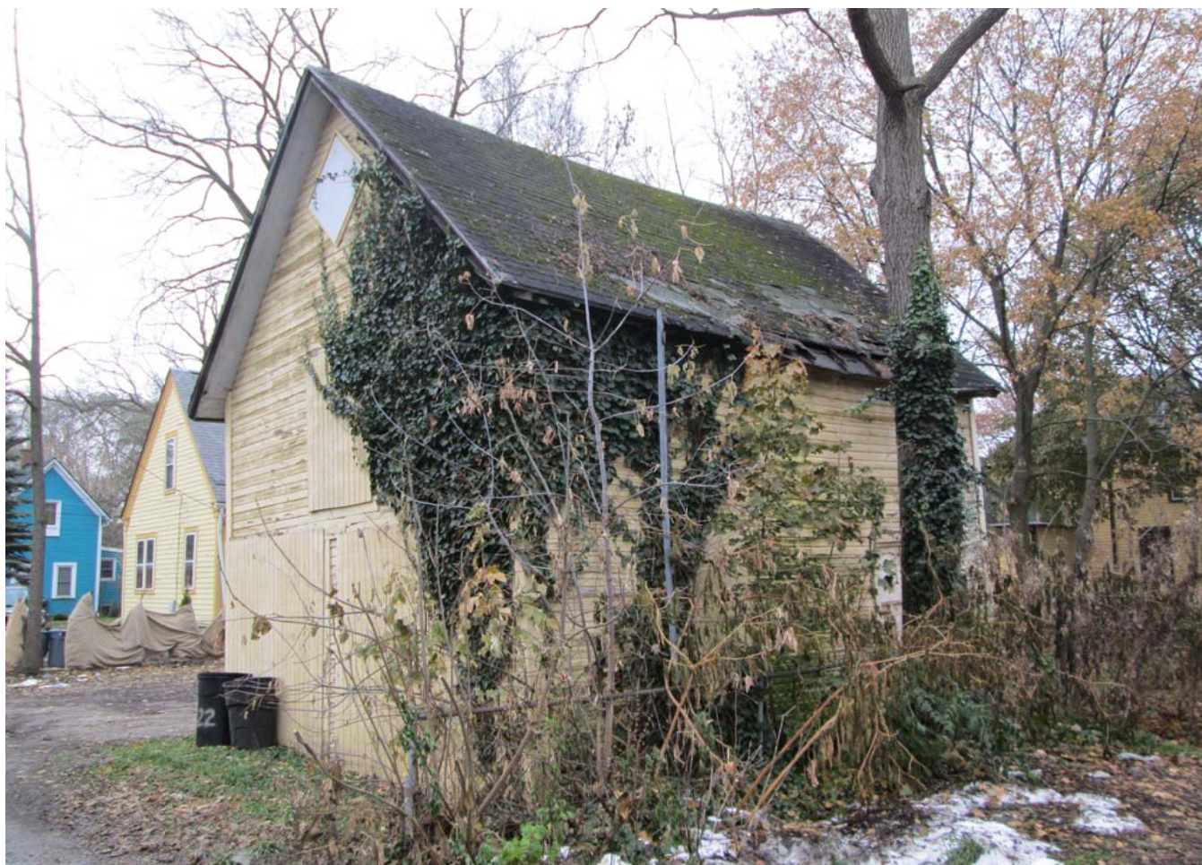
Facing southwest to north and east elevations
