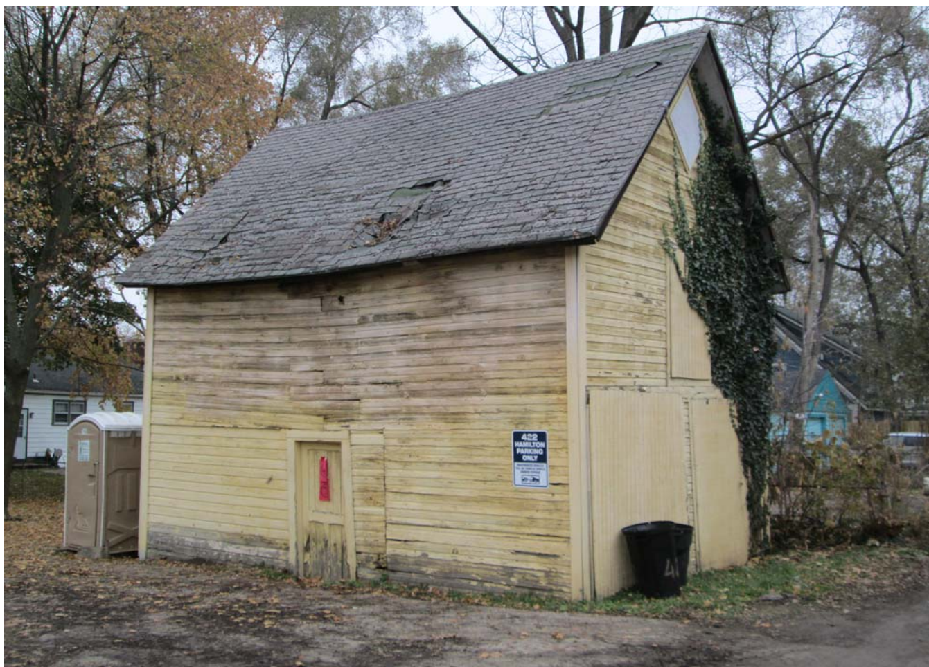
Facing north west to south and east elevations
