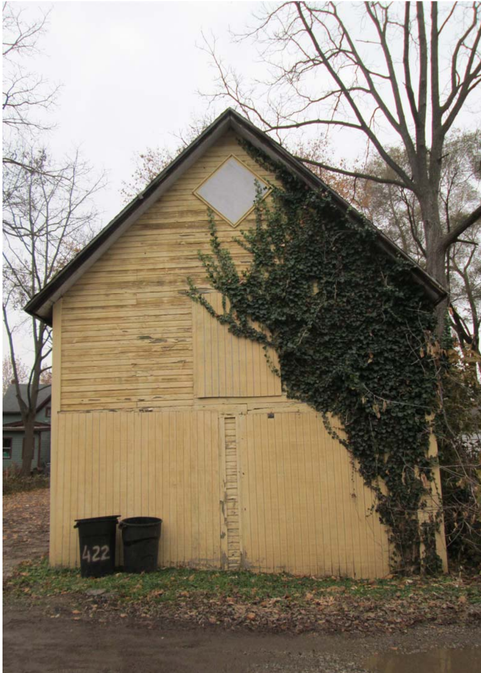
Facing west to east elevation.
